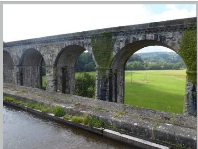
Plate 36. Aqueduct and Viaduct
