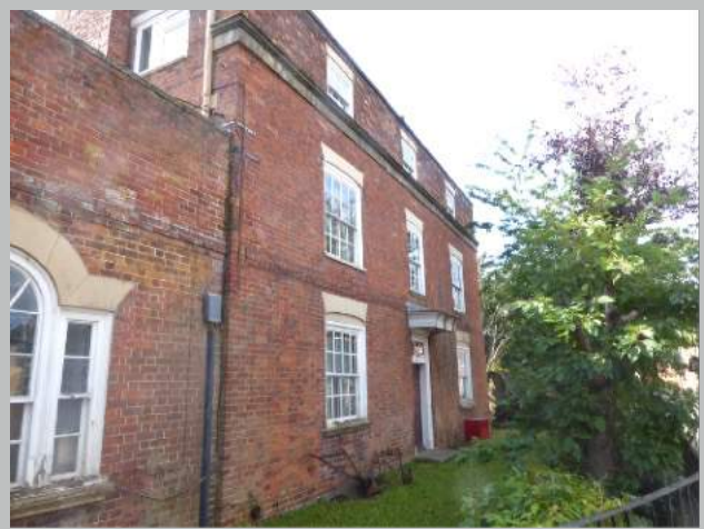
Plate 18. Another Georgian House
