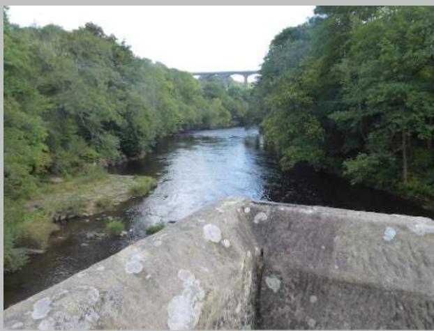
Plate 31. Pontcysyllte Aqueduct from the River Dee
