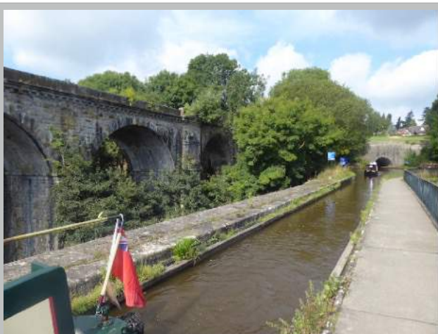
Plate 35. View N along Chirk Aqueduct
