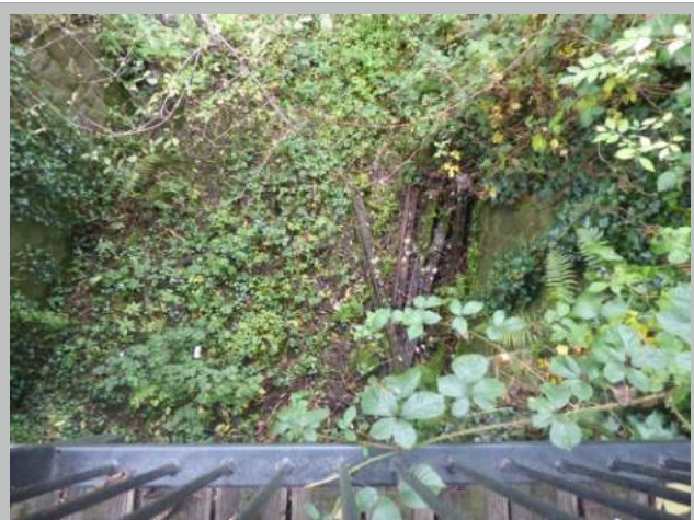
Plate 40. Stone embankment and loose tracks
