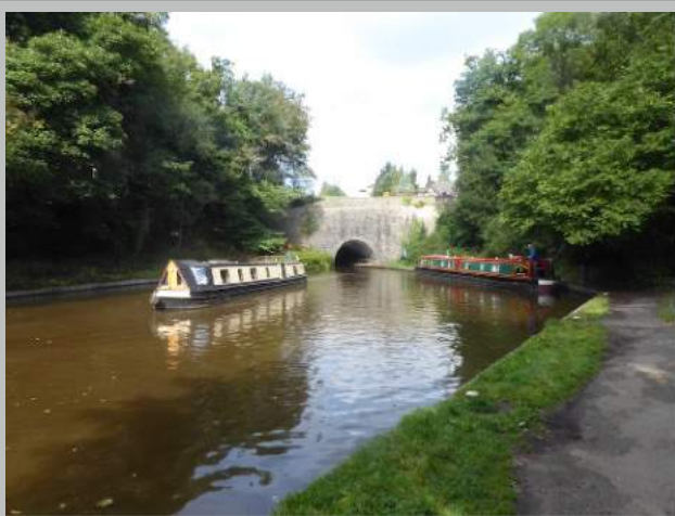
Plate 33. S Portal and "Waiting Area"
