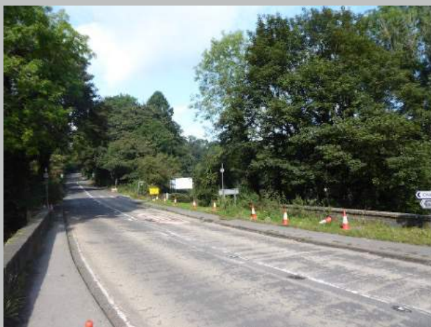
Plate 52. Telford's embankments on both sides of the road
