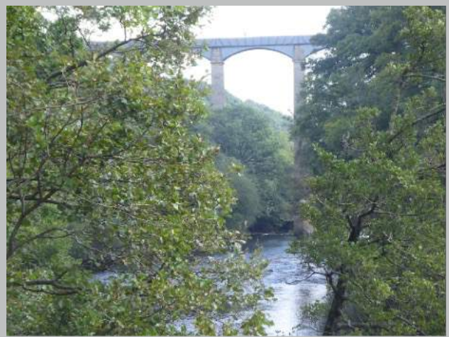
Plate 32 Pontcysyllte Aqueduct from the River Dee
