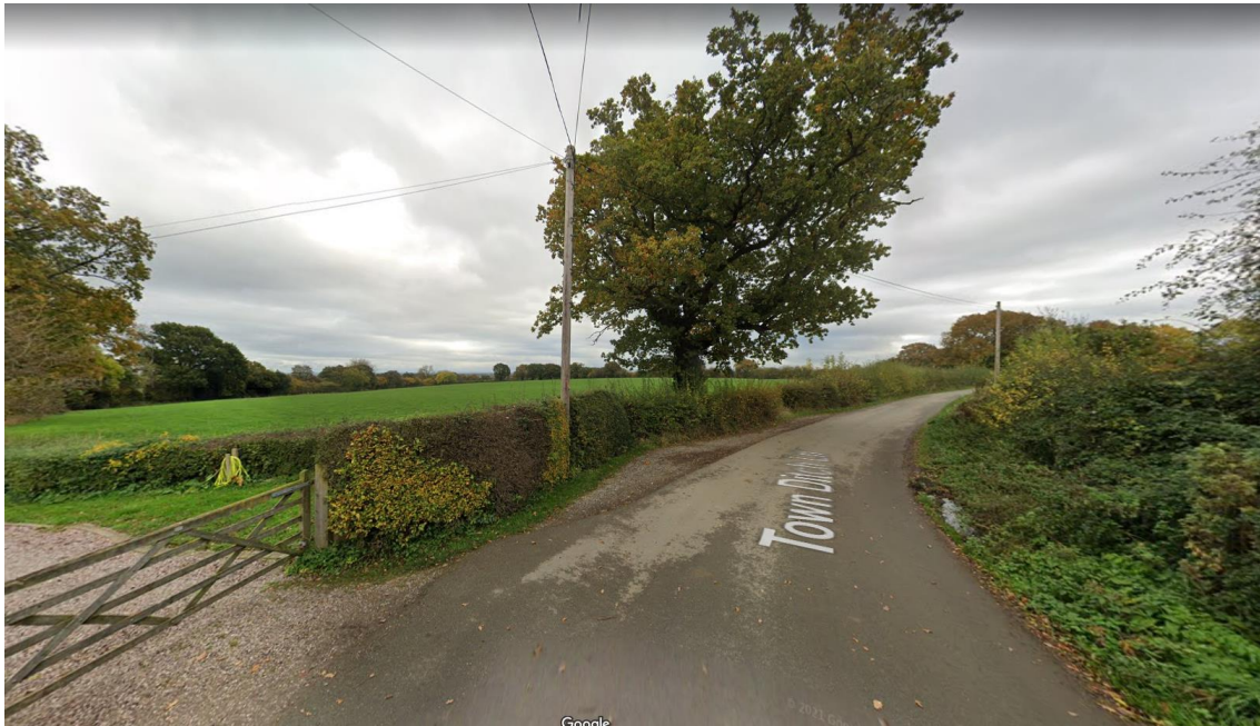
Figure 3 – View of existing access looking East.
