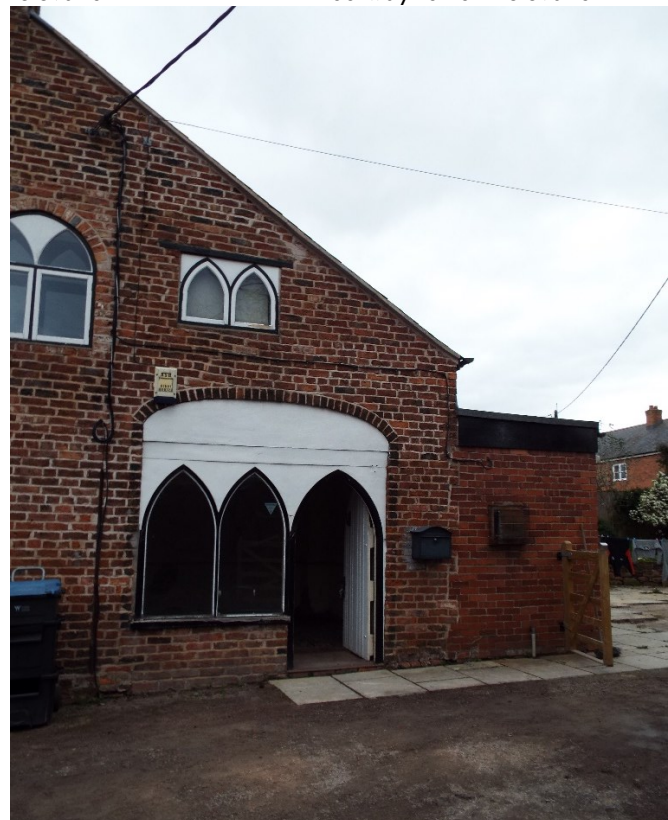
Southern side of west elevation
