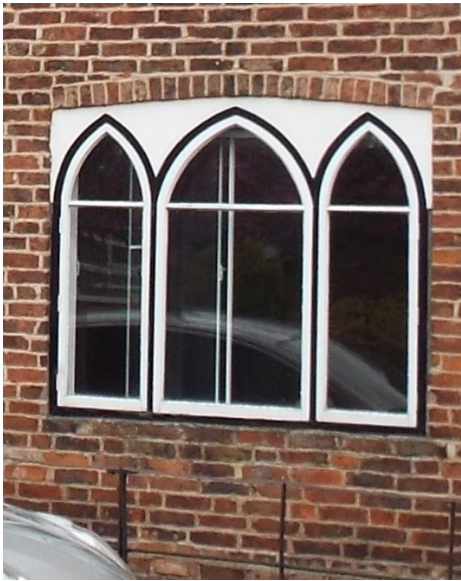
Window to north elevation
