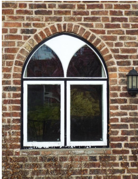
Window to north elevation
