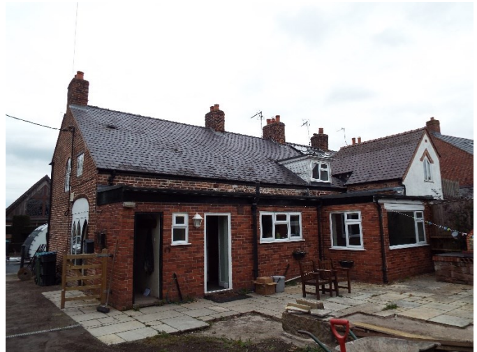
The southern façade
