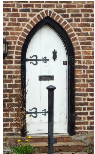
Doorway to north elevation
