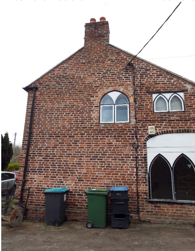
Northern side of west elevation
