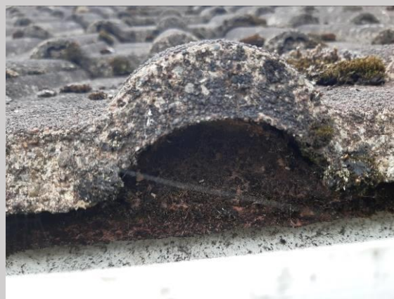
Photograph 10: Filled tile end
