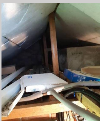
Photograph 5: Storage in larger roof void
