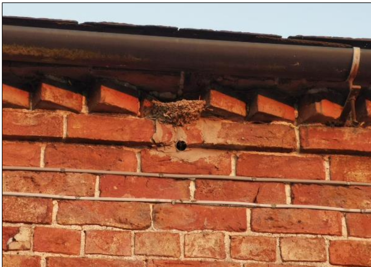
Plate 6 – Swallow nest cup below a gutter on the barn facing north-west
