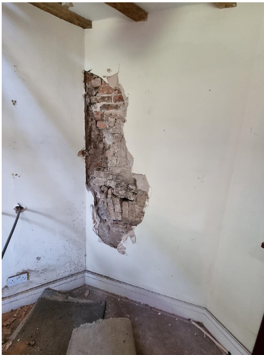
Photo 19: Detail of exposed chimney breast in former parlour, view to south west
