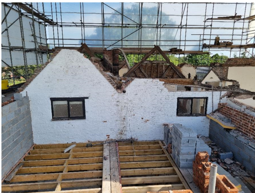
Photo 6: First floor western elevation, northern and central bays. View to east
