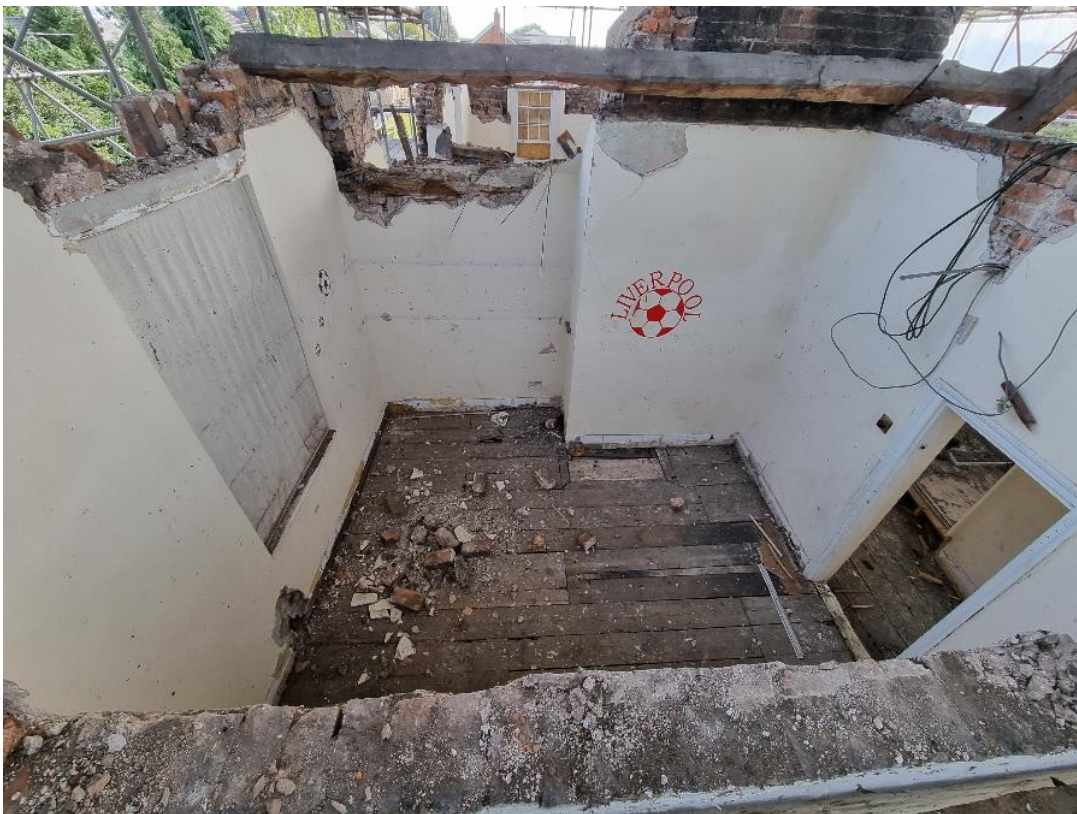
Photo 12: Bedroom 3 facing south
