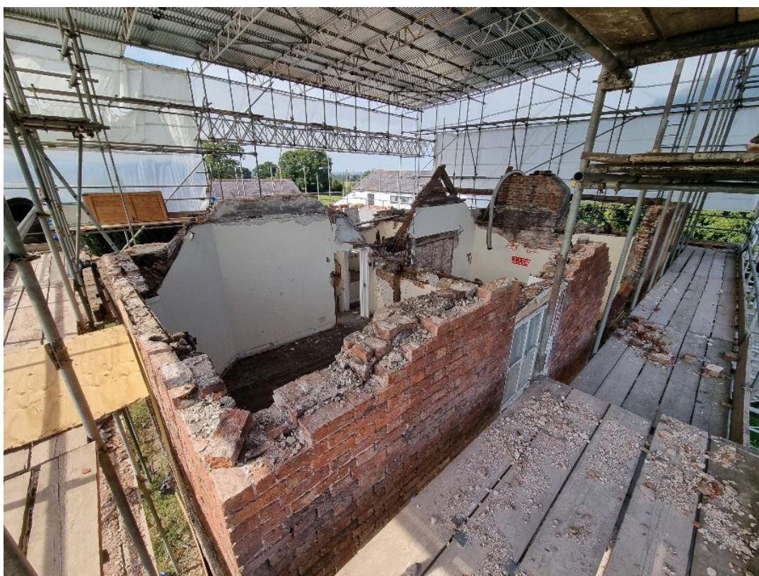
Photo 8: Eastern elevation, first floor, facing north west
