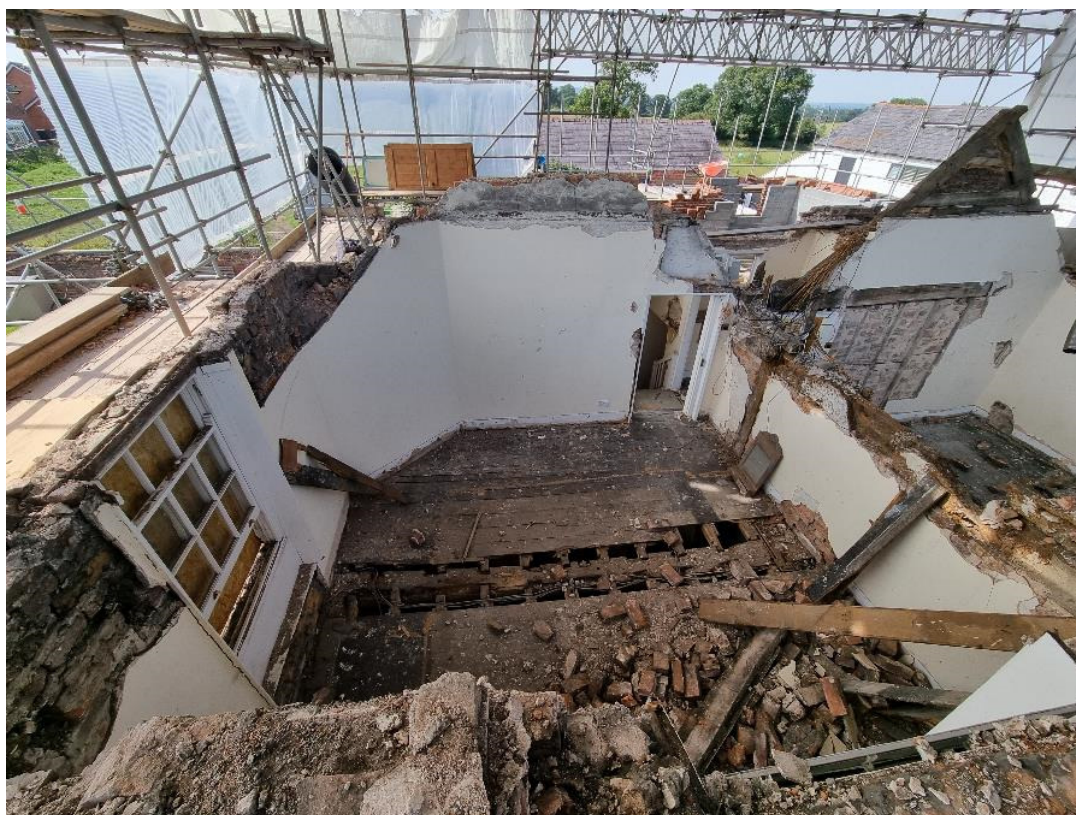
Photo 10: Bedroom 1 facing west
