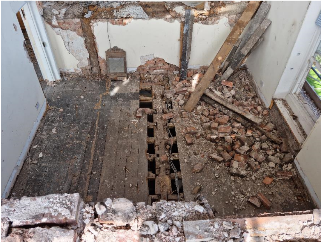
Photo 13: Bedroom 1 facing north
