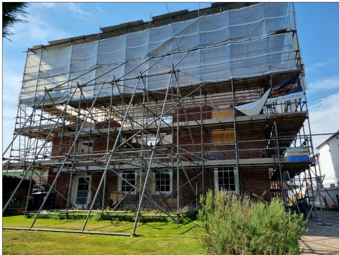
Figure 2: Holt Hill, eastern elevation
