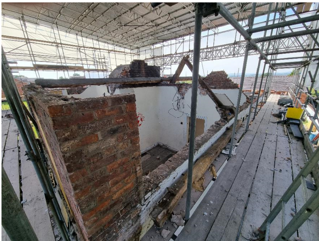
Photo 9: Northern elevation, first floor, facing west
