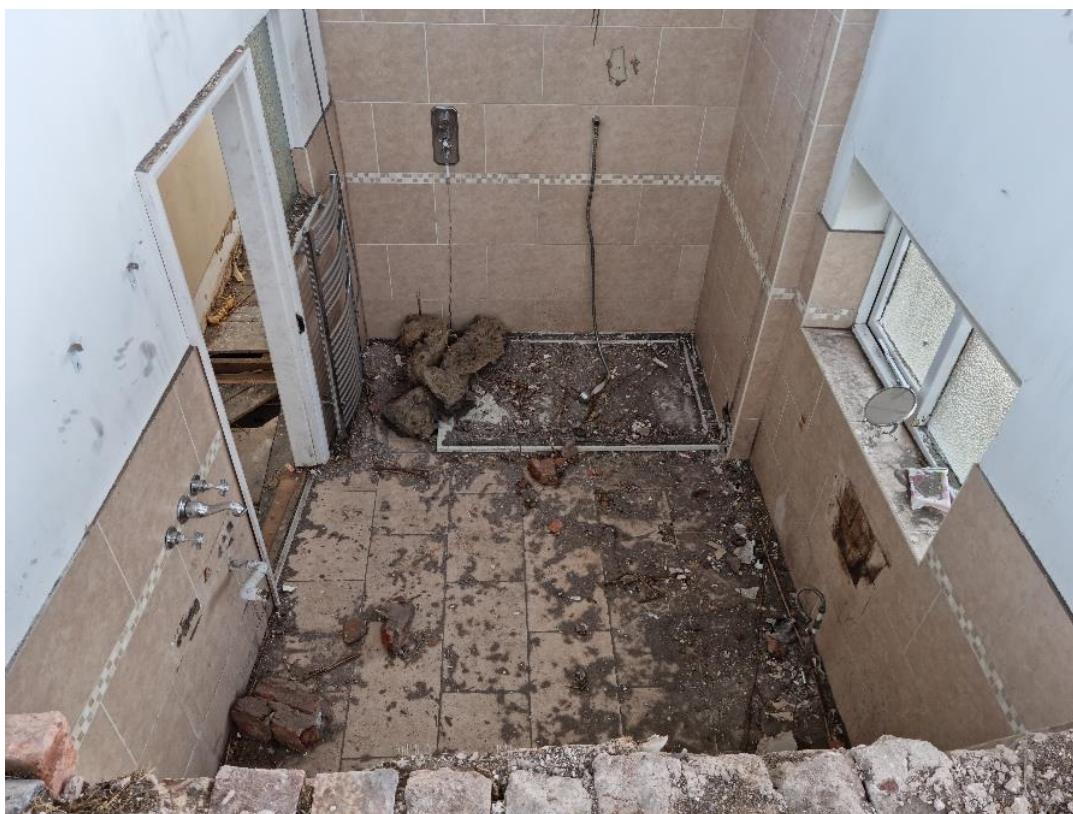
Photo 17: Bathroom, facing south
