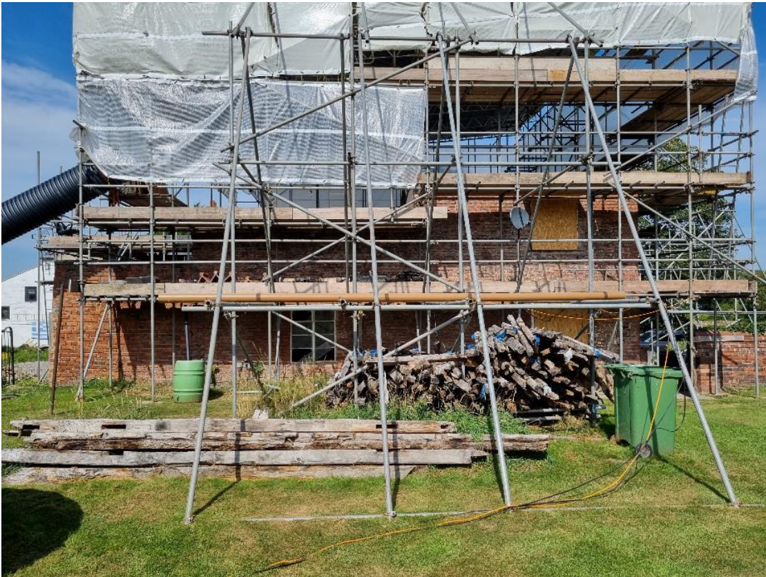
Photo 4: Southern elevation, view to north
