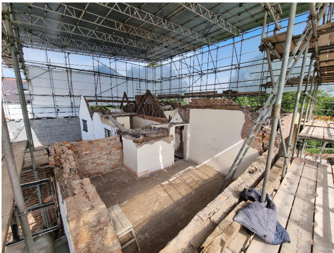
Photo 7: First floor, Bedroom 4 facing north east
