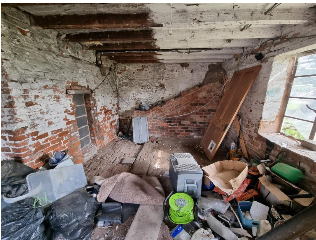
Photo 23: Garage, view to east
