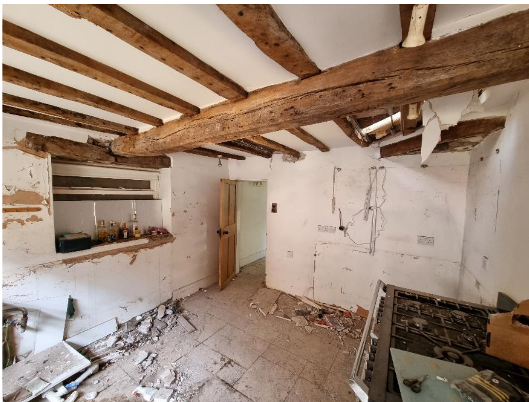
Photo 25: Kitchen, view to north east
