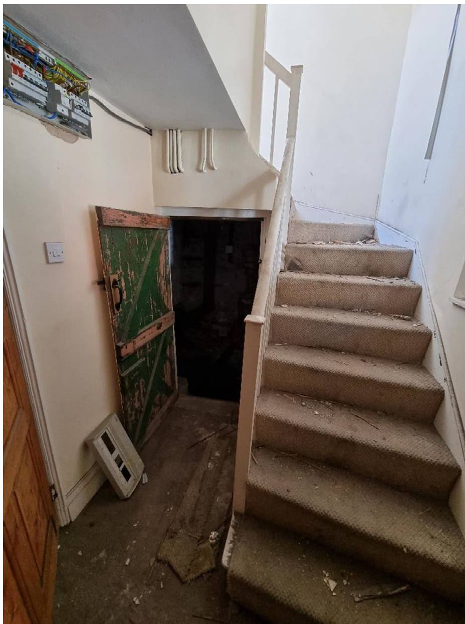
Photo 24: Hallway, view to south
