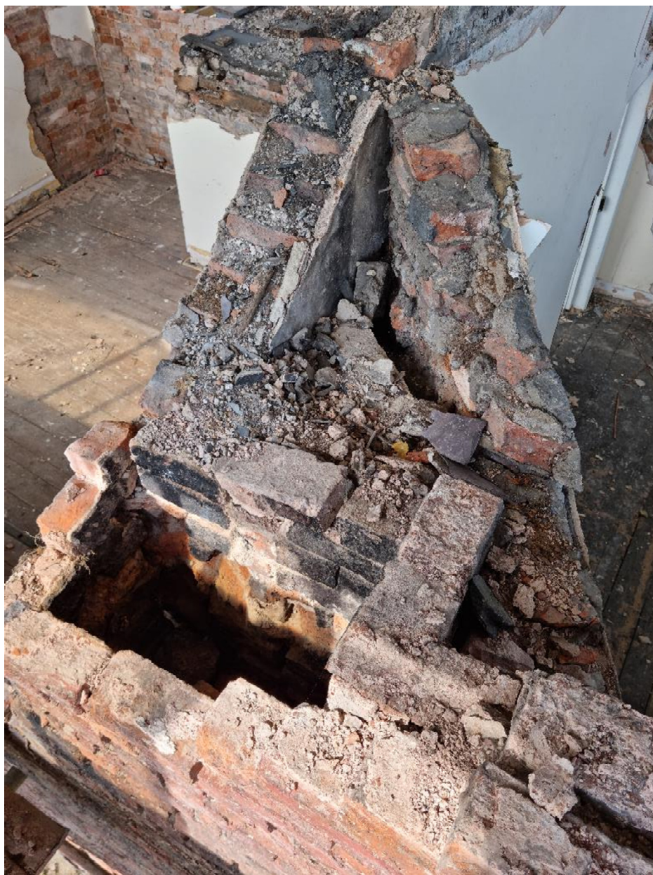
Photo 15: Detail of corner chimney, Bedroom 1, facing north west
