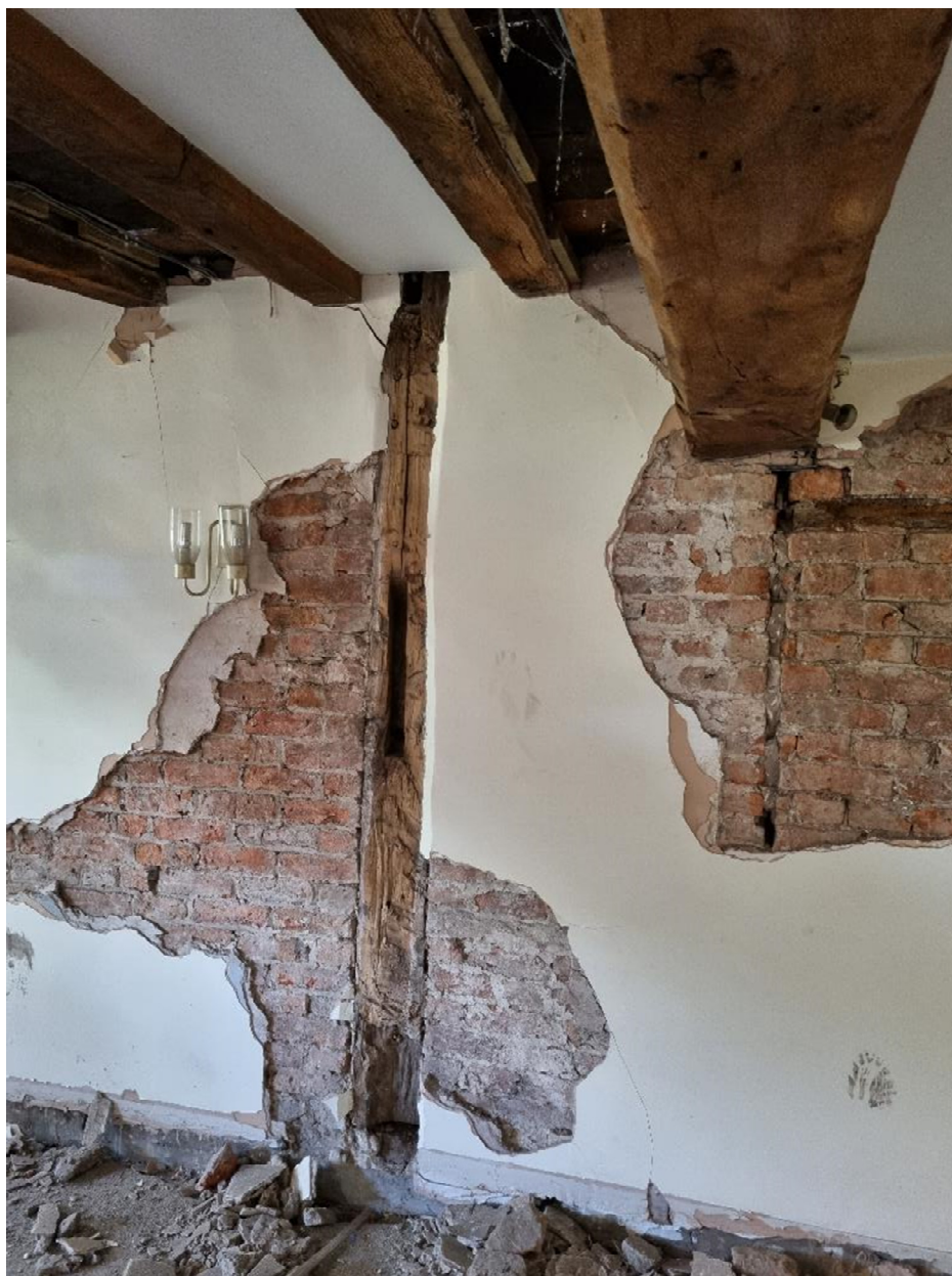
Photo 21: Detail of exposed wall upright and lintel embedded in wall to west, lounge, view to south
