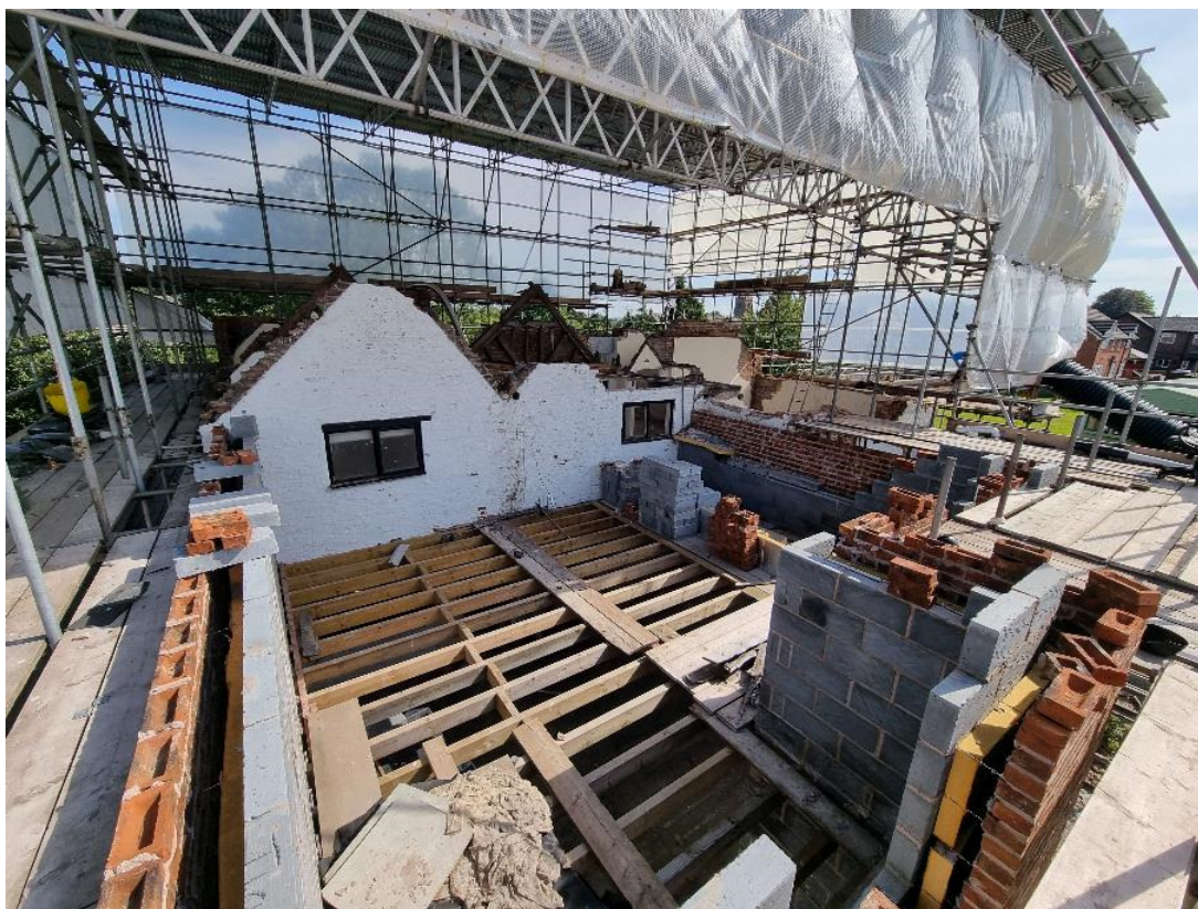
Photo 5: First floor western elevation, view to south east across new extension
