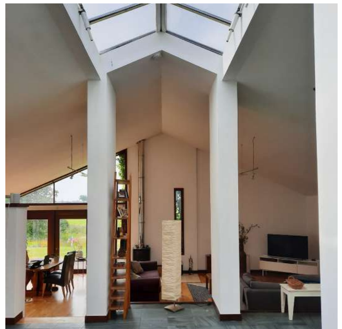
Right: Existing roof-light that runs the length of the corridor
