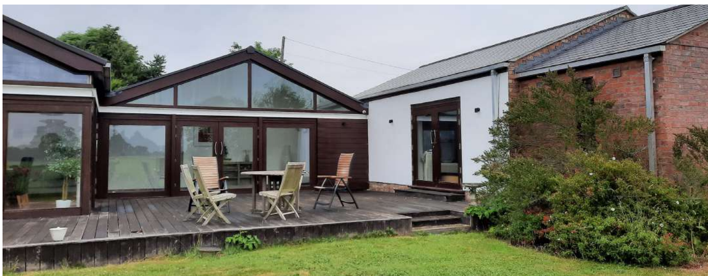
Above: The existing south elevation of the pitched roof corridor link - to be demolished
