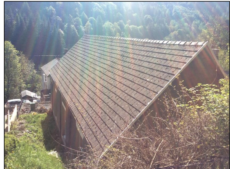
Northern elevation and western gable end.
