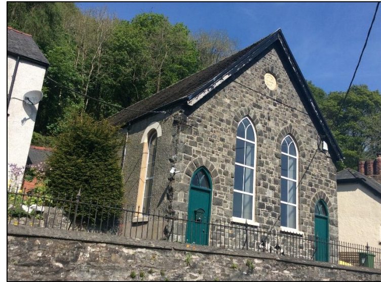
Southern elevation and eastern gable end.
