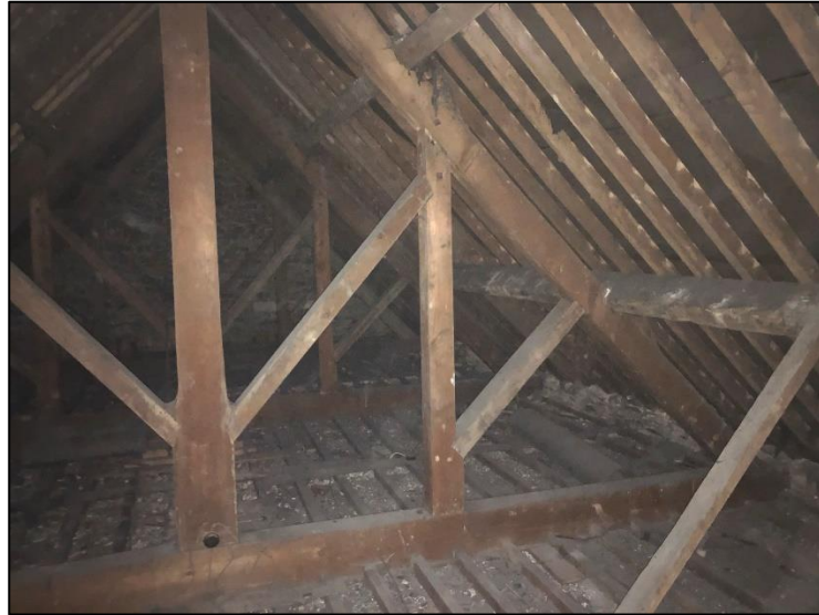
Loft space two, looking east.
