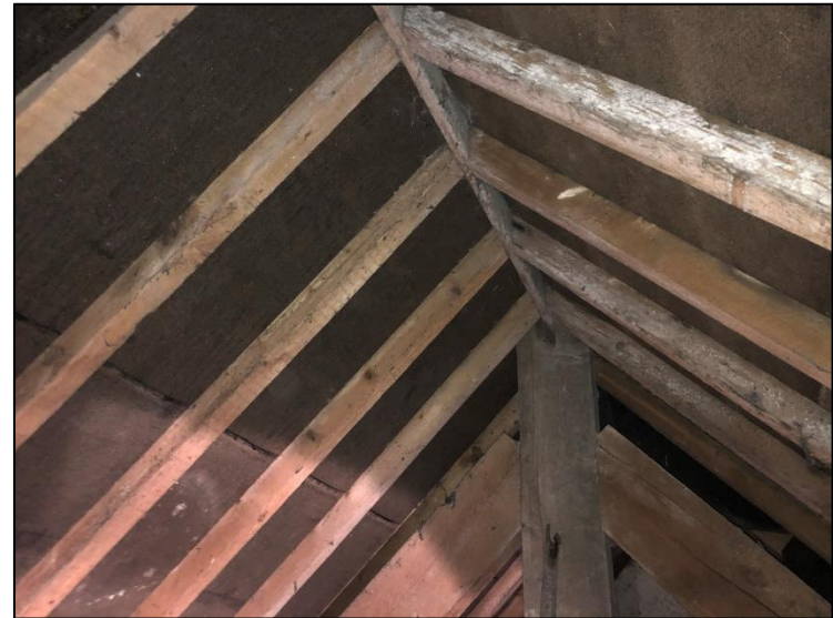
Loft space one, roof structure.
