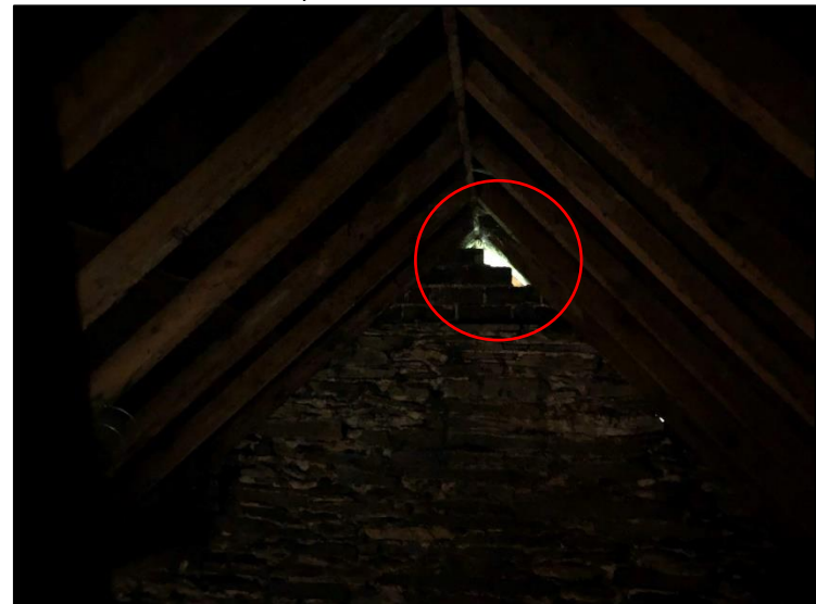
Loft space one, gaps in the apex of western gable end.
