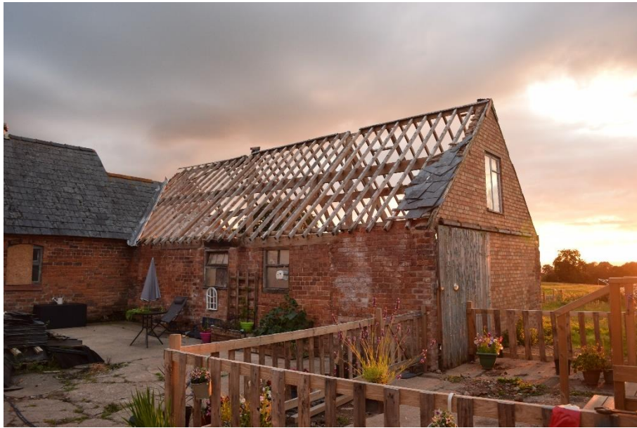
Figure 4.10. Barn 1.3 from west
