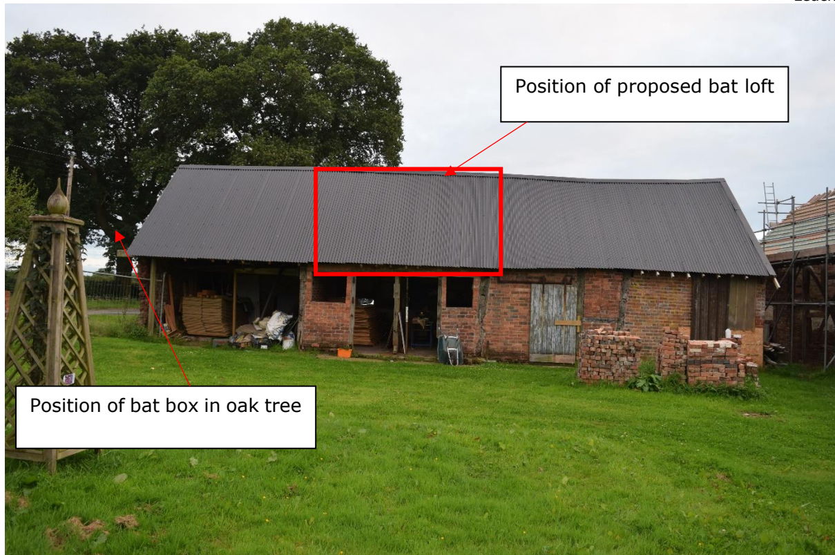
Figure 5.5. Mitigation on barn 2 and tree
