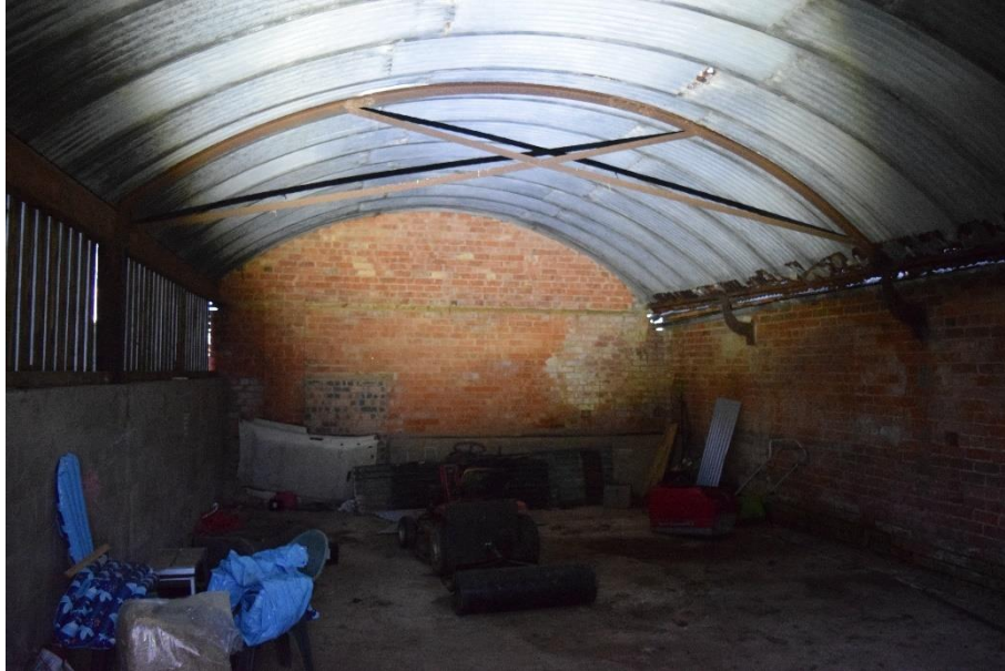
Figure 4.12. Interior of B1.4
