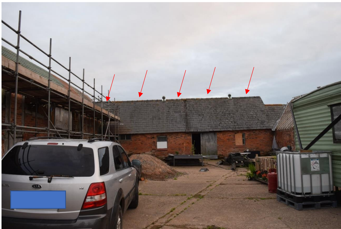
Figure 5.4. Showing approximate positions of bat access under ridge tiles on 1.2
