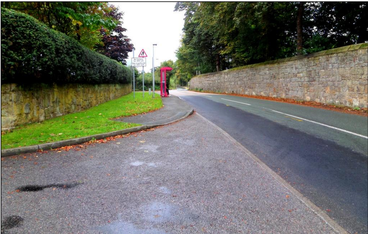
2.4x185m visibility to the left from the site exit
