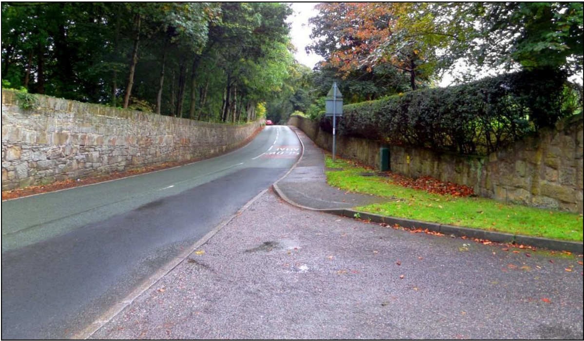
2.4x240m visibility to the right from the site exit
