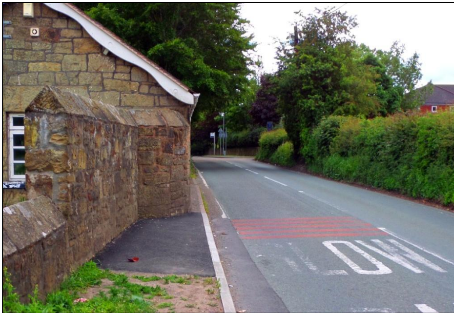
Approach from the North
