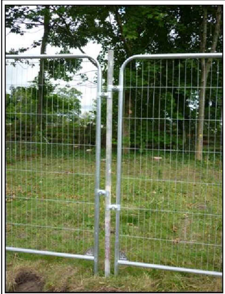
Tree Protective Fencing Specification
