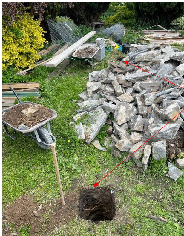
(x2 excavated hole locations)
