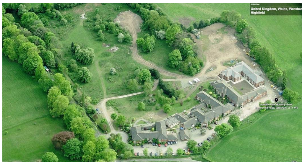
Early birds-eye view of Pendine Park showing the walled boundary to Summerhill Road and dense boundaries (pre quadrangle and laundry block construction – see below)
