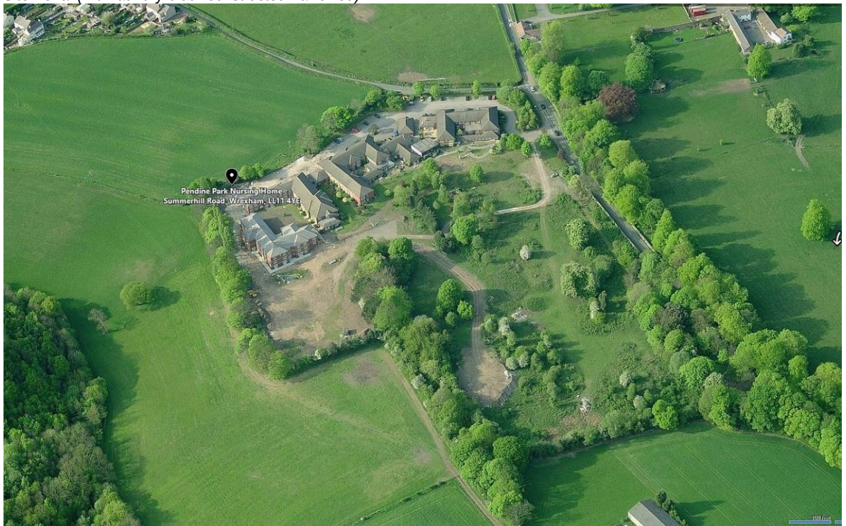
Pre Quad Building & Laundry block construction Birdseye view 1 (for illustration only)
