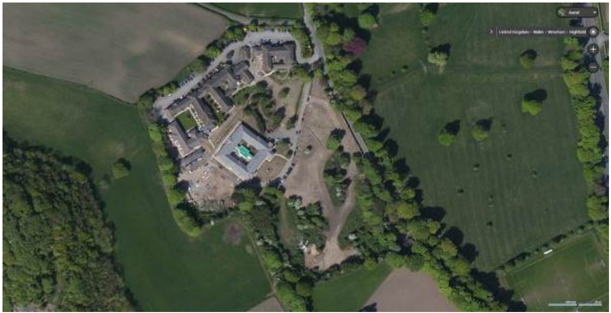
Site aerial (pre-laundry block construction)
