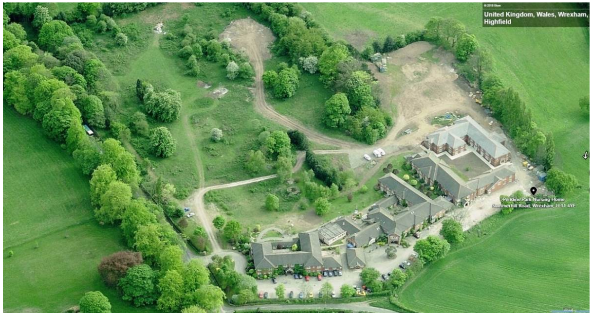
Pre Quad Building & Laundry block construction Birdseye view 4 (for illustration only)
