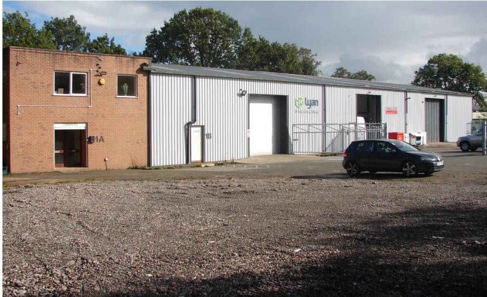
The southern elevation of the building ( Target Note 7 ) from the proposed development site.
