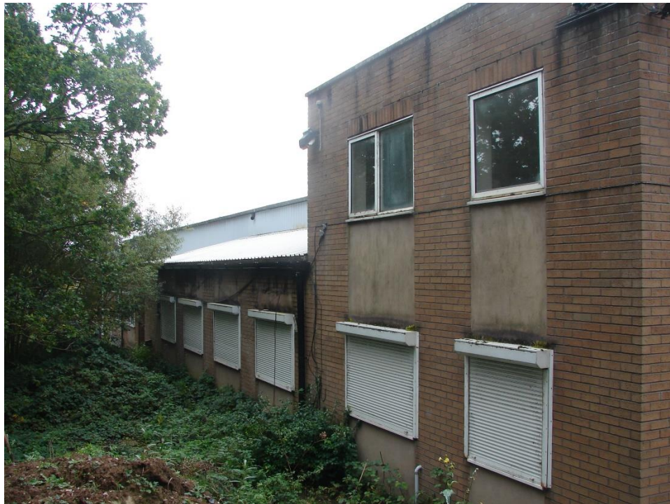
Part of the northern elevation of the building ( Target Note 7 ).
