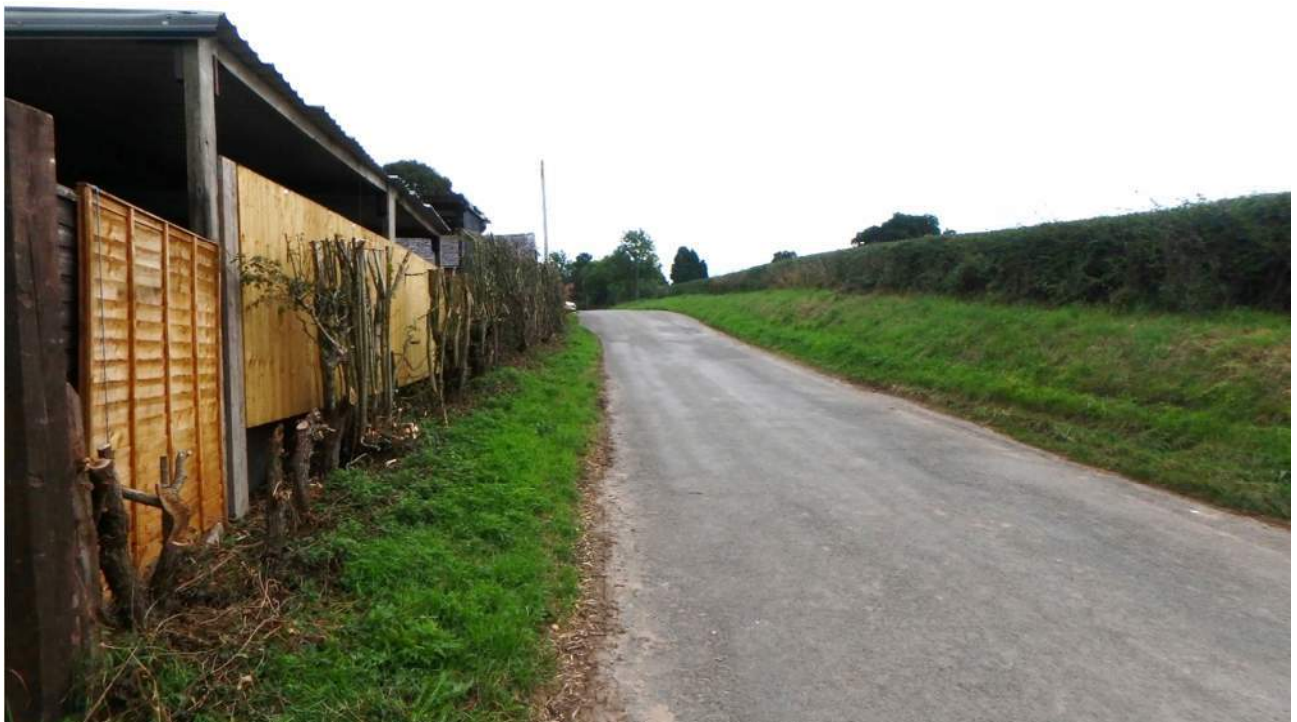
PHOTOGRAPH 4 Road channel in a easterly direction from the existing access
