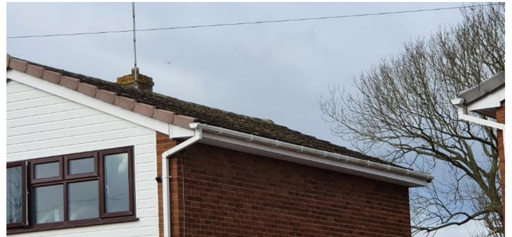
B1 – eastern elevation roof (pictured above).
