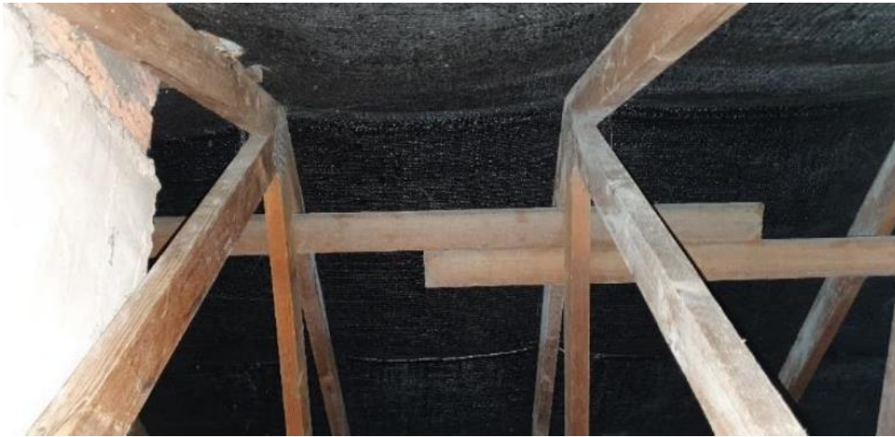
B1 – loft roof structure (pictured above).
