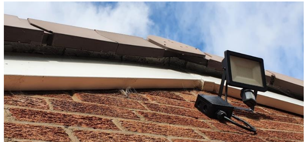
B1 – example of the fascias in good condition with cobwebs present (pictured above).
