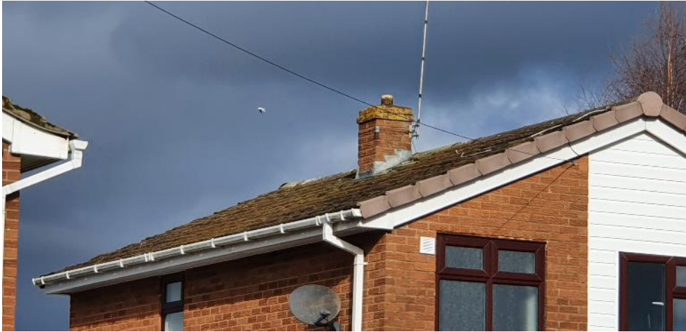
B1 – western elevation roof (pictured above).
