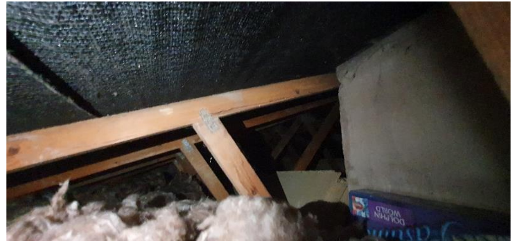
B1 – loft roof structure (pictured above).
