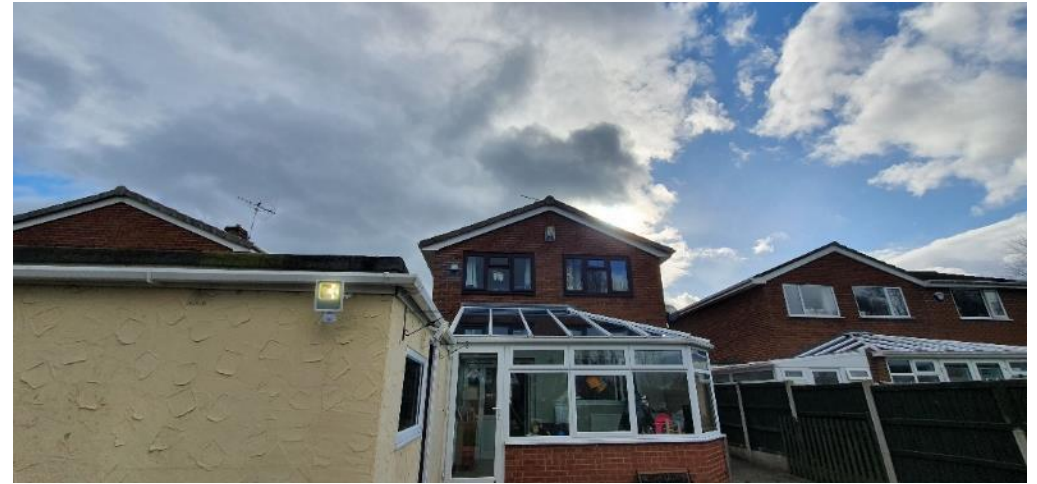
B1 – north western elevation (pictured above).
