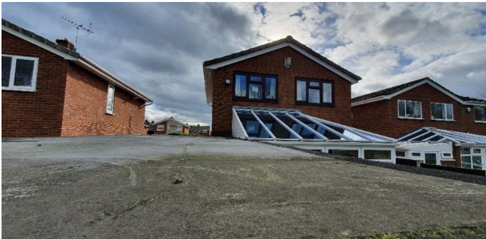
B1 – garage roof and north western elevation (pictured above).
