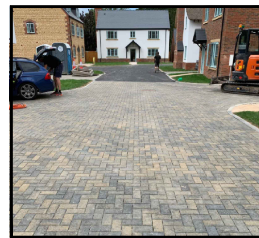
Permeable Block paving
