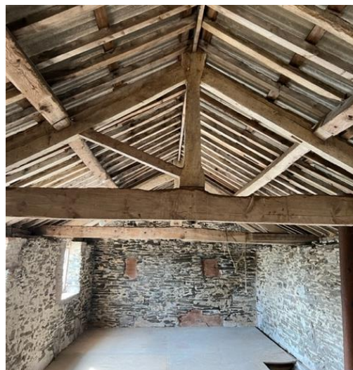
(timber roof structure)
