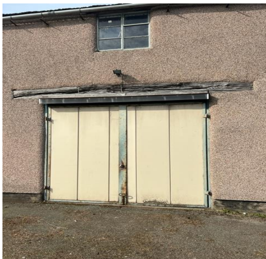
(existing supporting beam on the East elevation)
