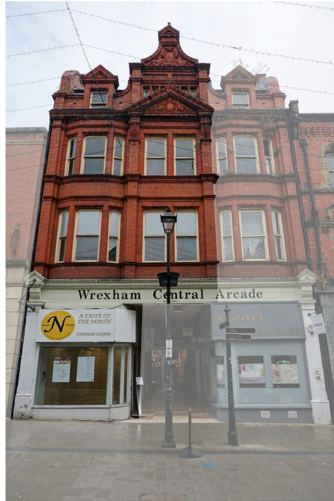
Image 01 - Photograph of existing front elevation with No. 58 highlighted
