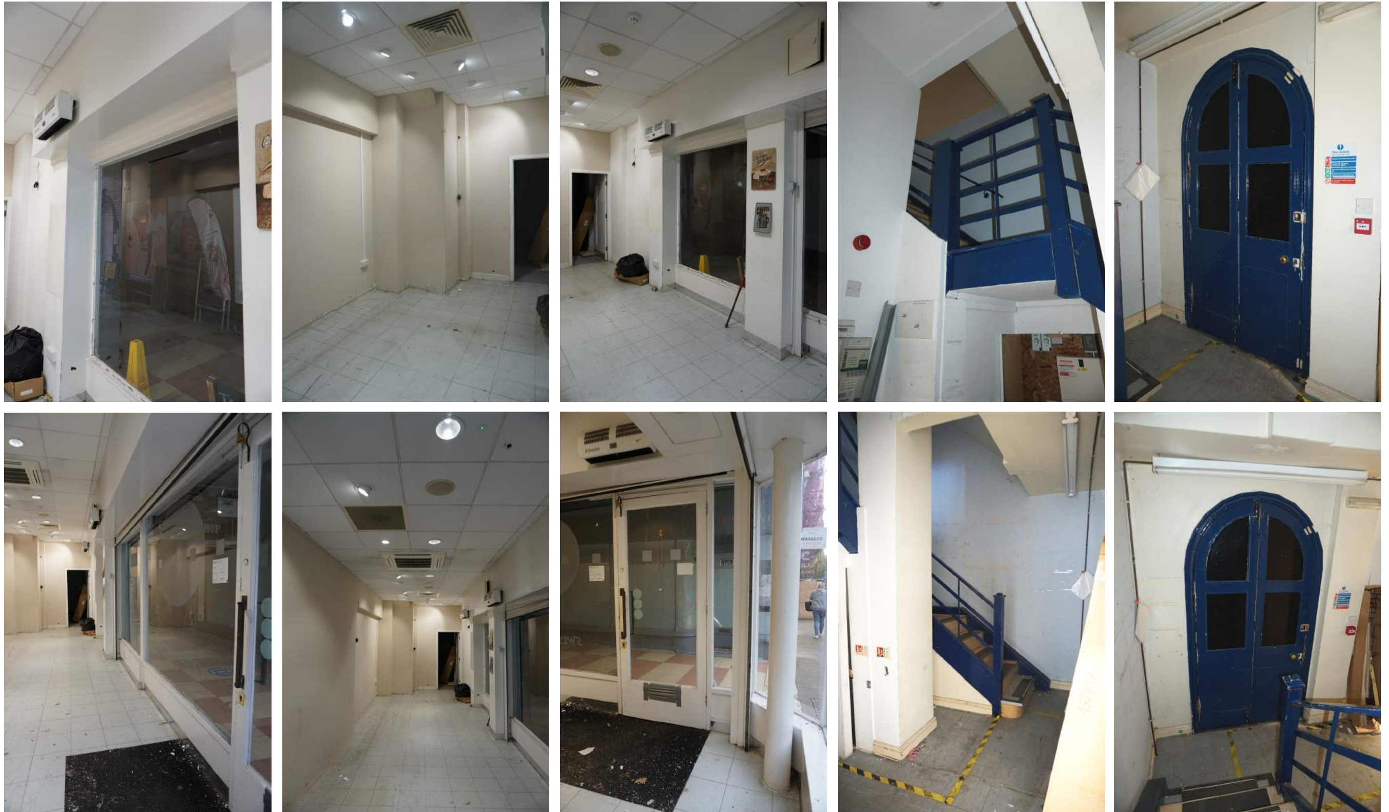
EXISTING GROUND FLOOR PHOTOGRAPHS
