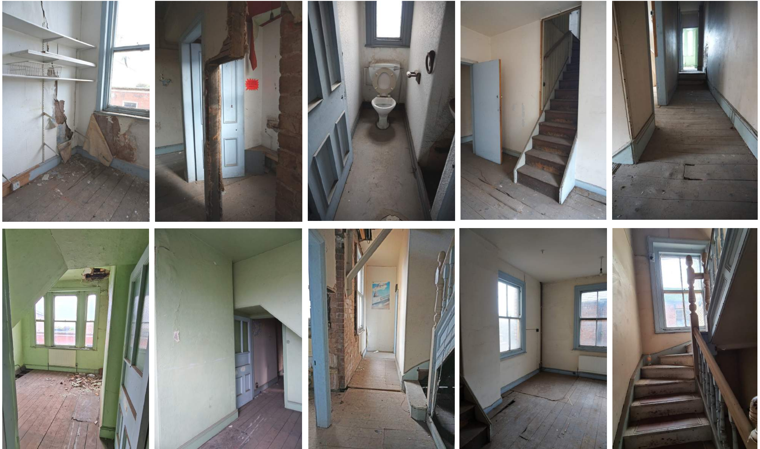
EXISTING SECOND FLOOR PHOTOGRAPHS
