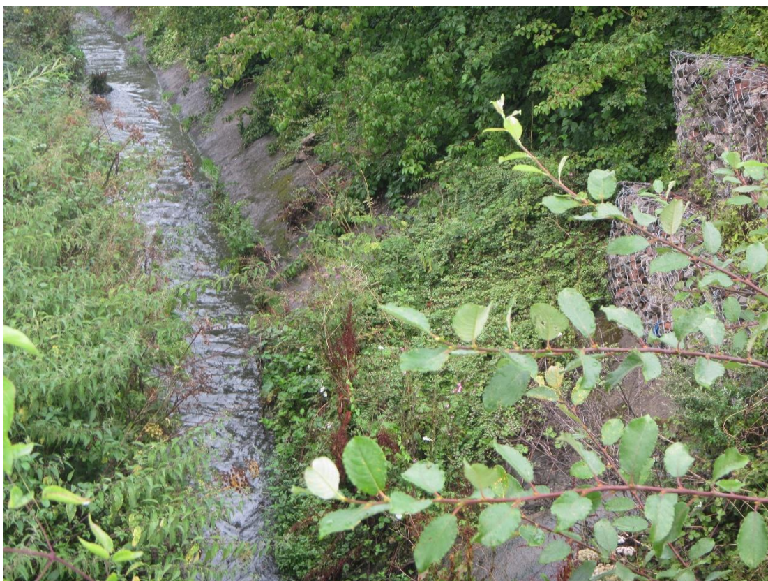
Photograph 7 – View of watercourse and gabion baskets.
