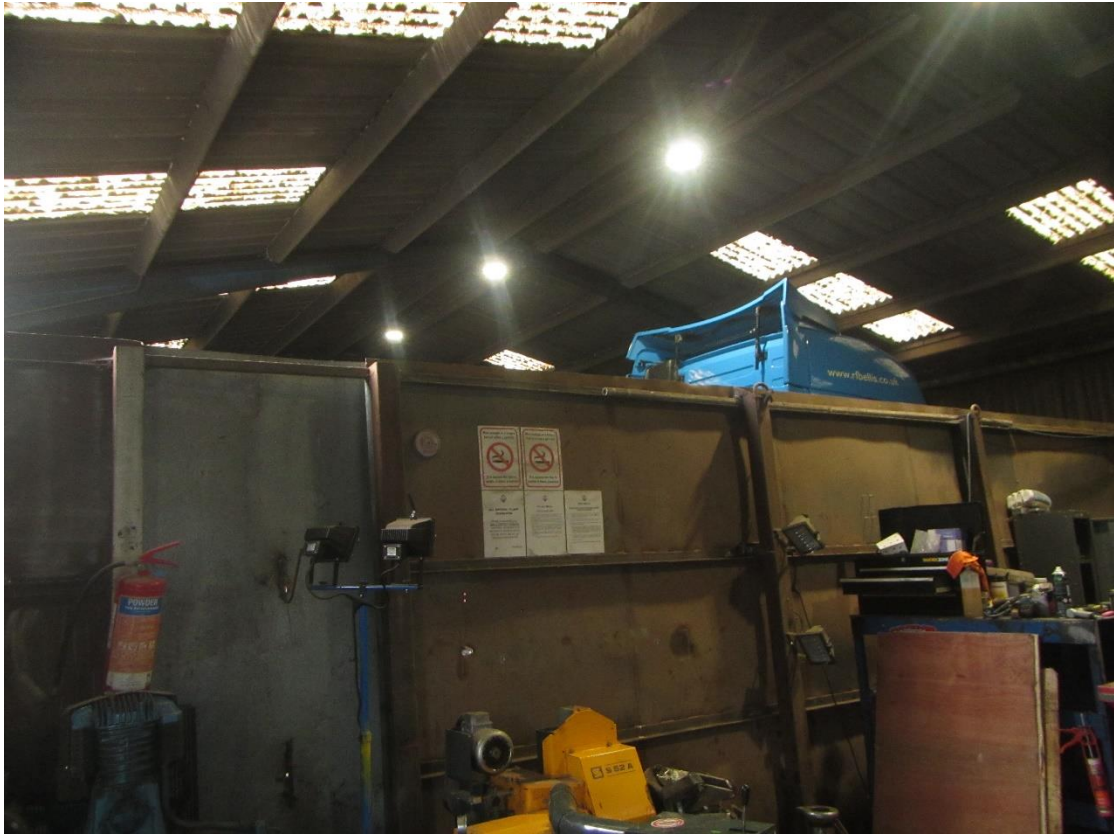
Photograph 23 – Internal view of Building C.
