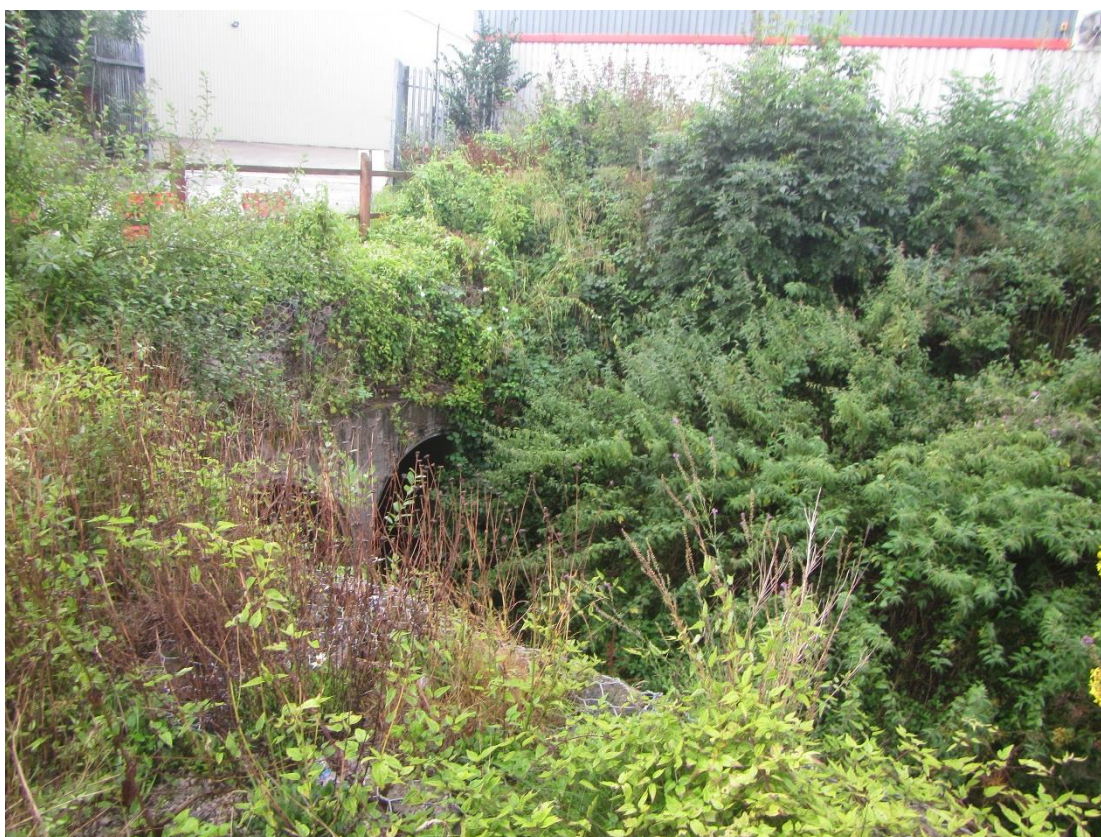
Photograph 8 – View of culvert on the south-eastern survey boundary of Redwither Brook.
