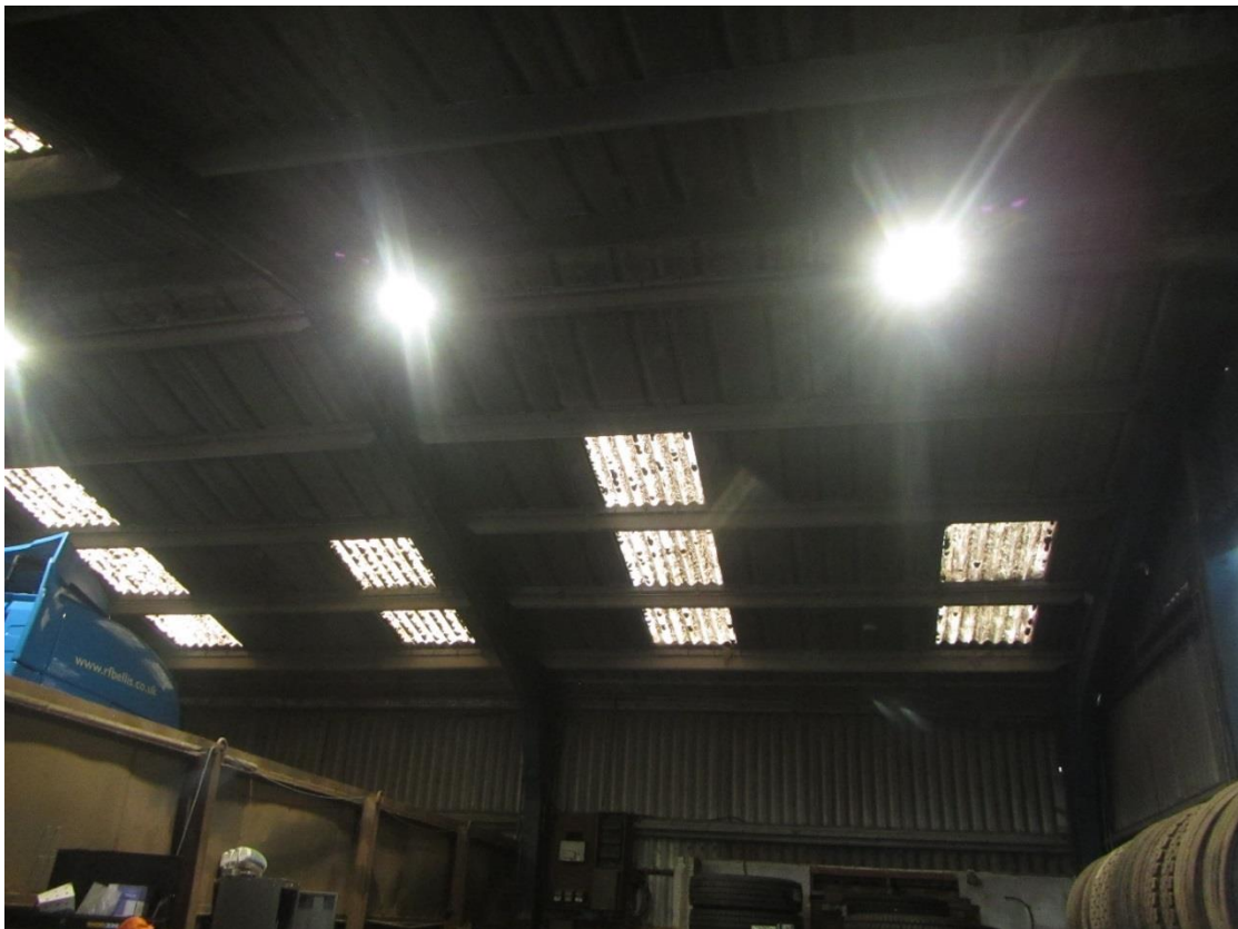
Photograph 16 – View of roof on Building C.
