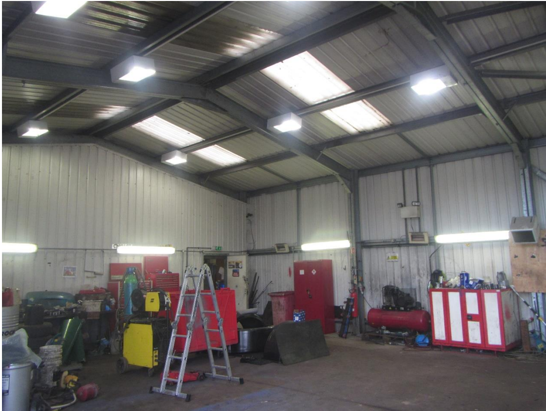
Photograph 25 – Internal view of Building E.
