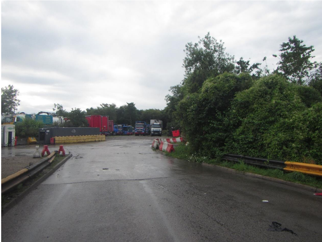
Photograph 1 – Looking south-east across site, view of dense scrub.
