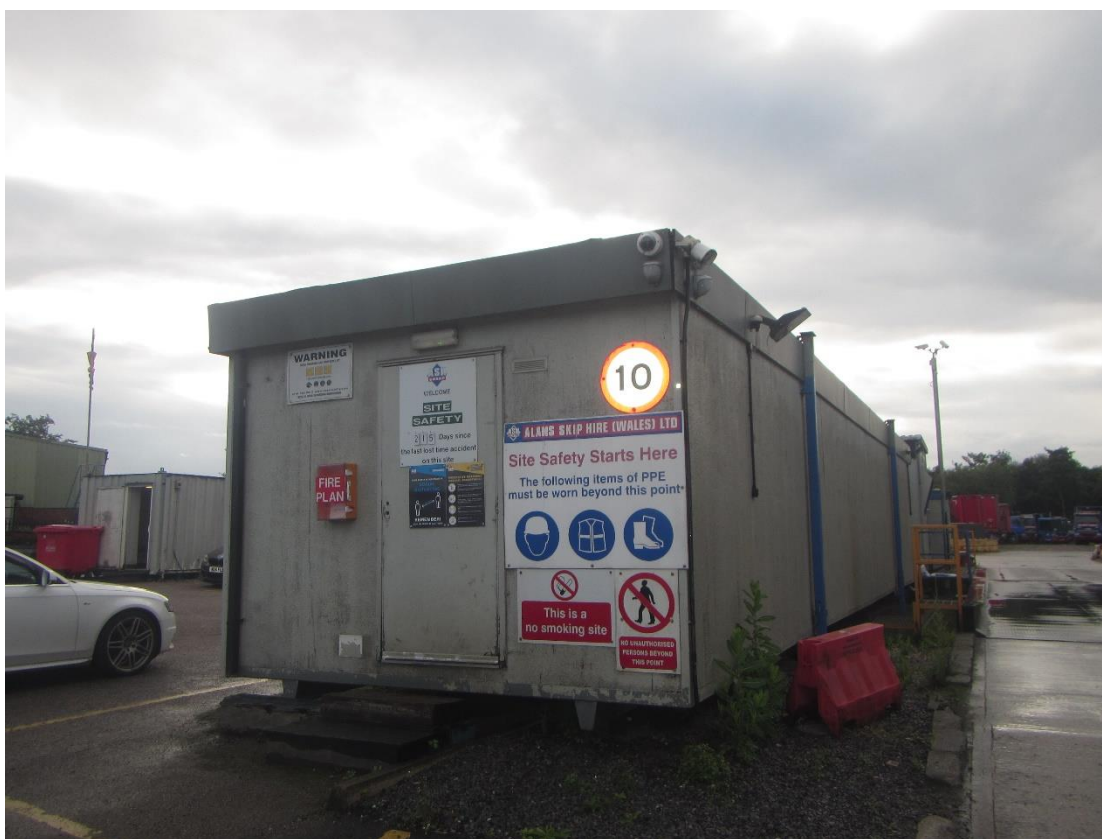
Photograph 12 – Building A viewed from west
