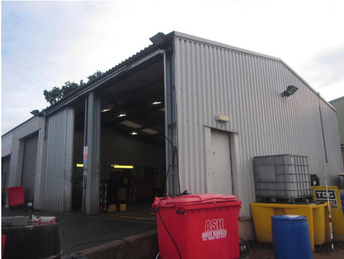
Photograph 19 – Southern and eastern aspects of Building E.
