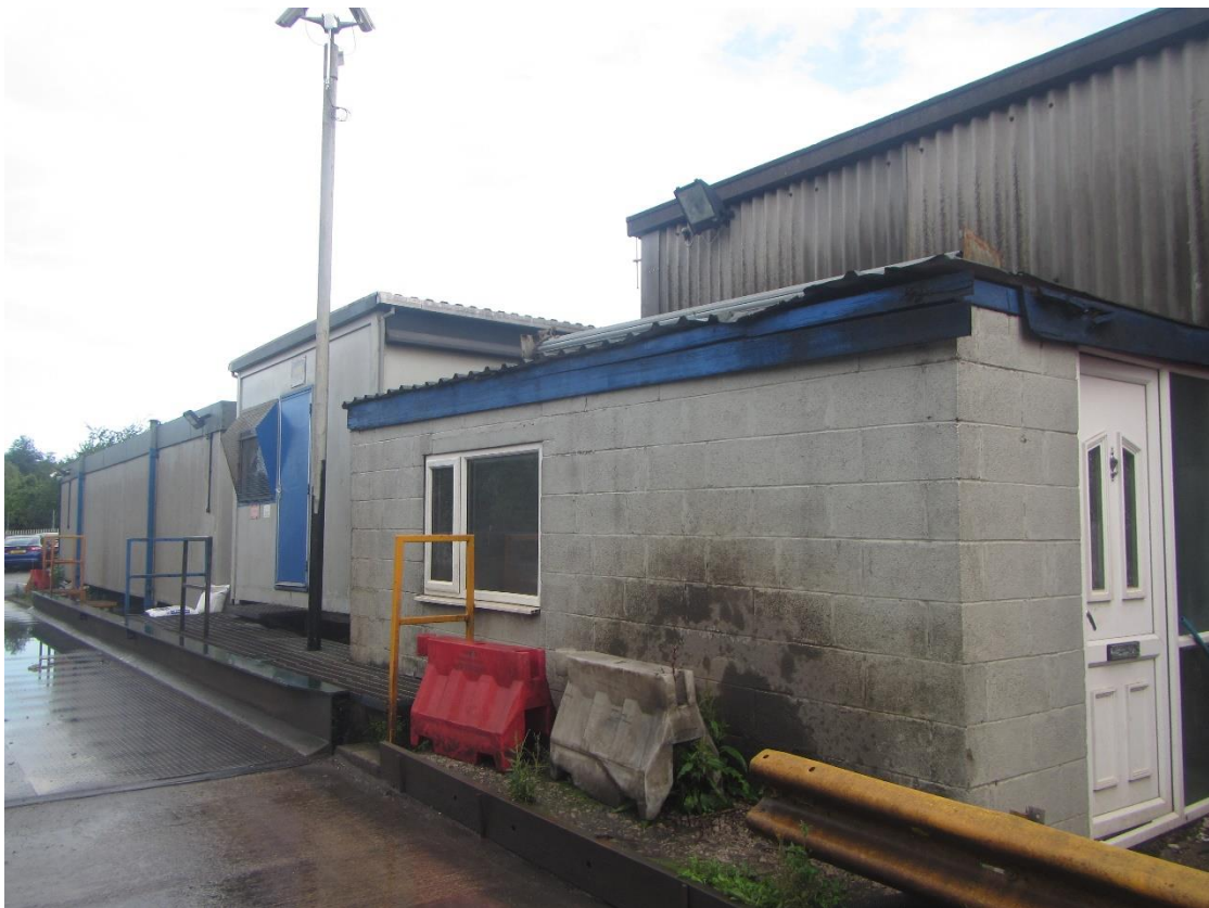
Photograph 18 – Southern aspect of Building D.
