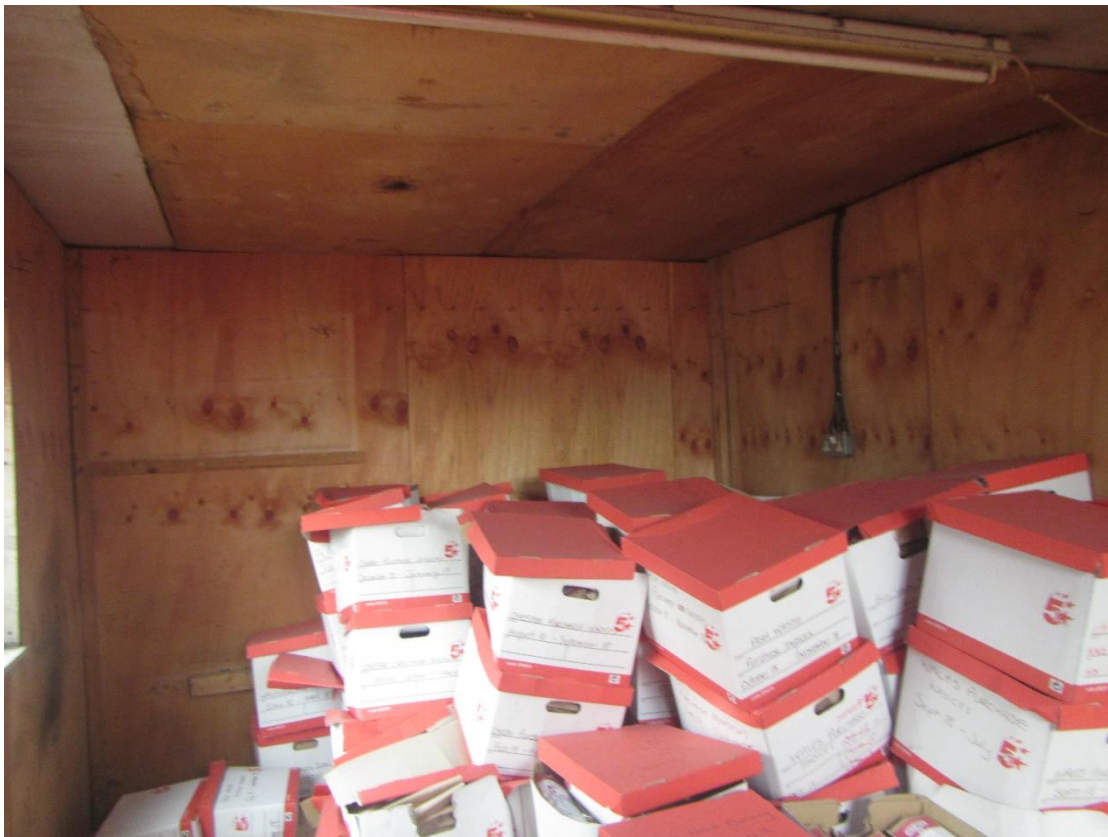
Photograph 24 – Internal view of Building D.
