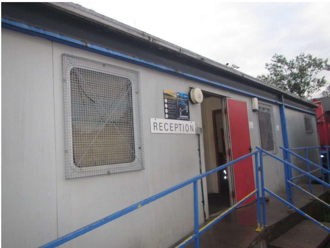
Photograph 14 – Western aspect of Building B.
