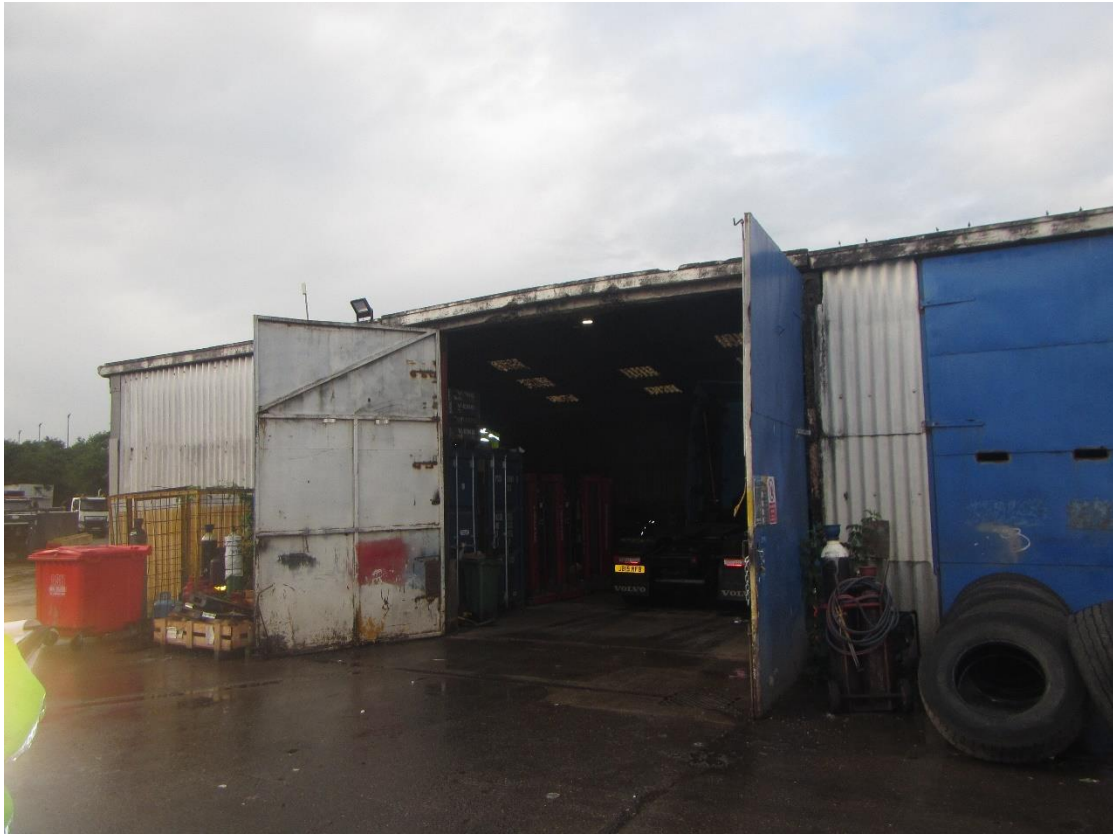
Photograph 15 – Northern aspect of Building C.
