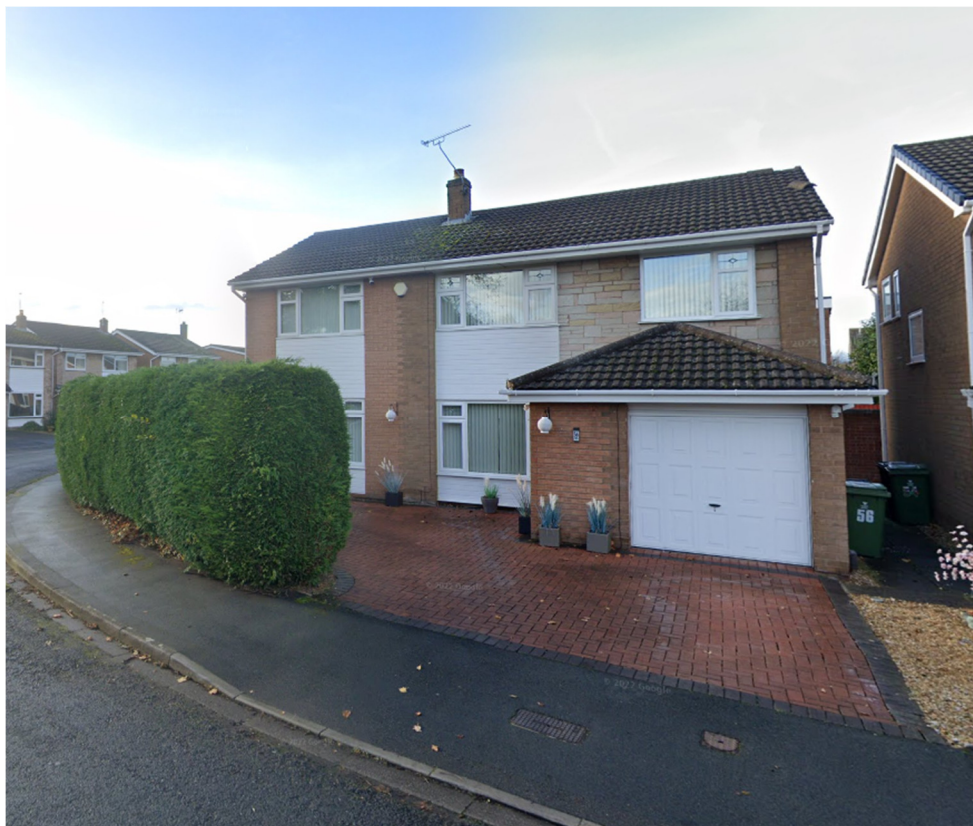
56 Ffordd Llywelyn (Shown above).
