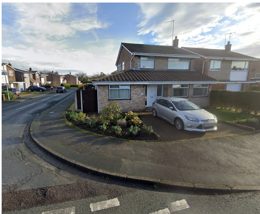
4 Ffordd Llywelyn (Shown above).
