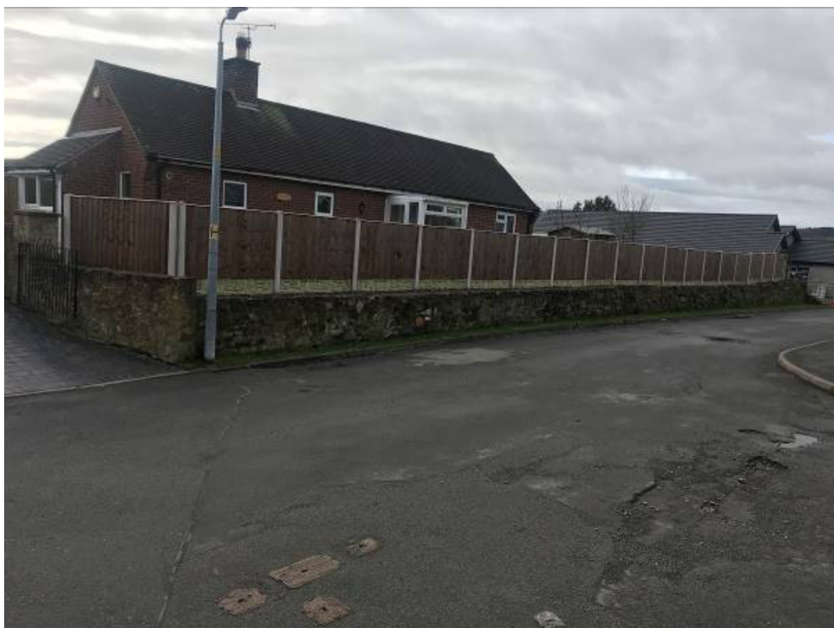
Similar view looking towards neighbouring property (Golygfan)
