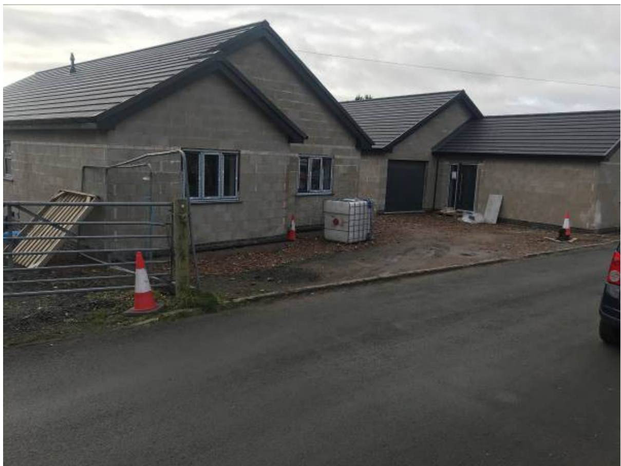
Bungalows currently under construction adjacent to Golygfan
