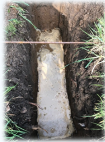
SA3 Water test
