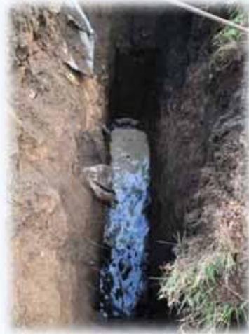
SA1 Water test
