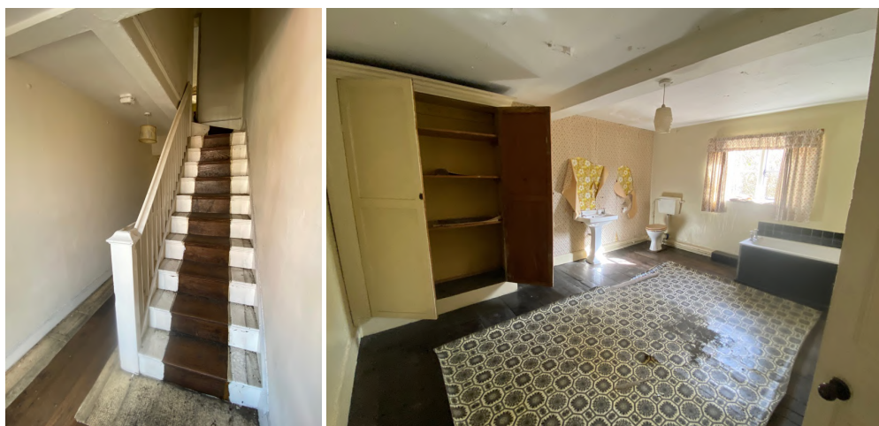
Hall and bathroom
