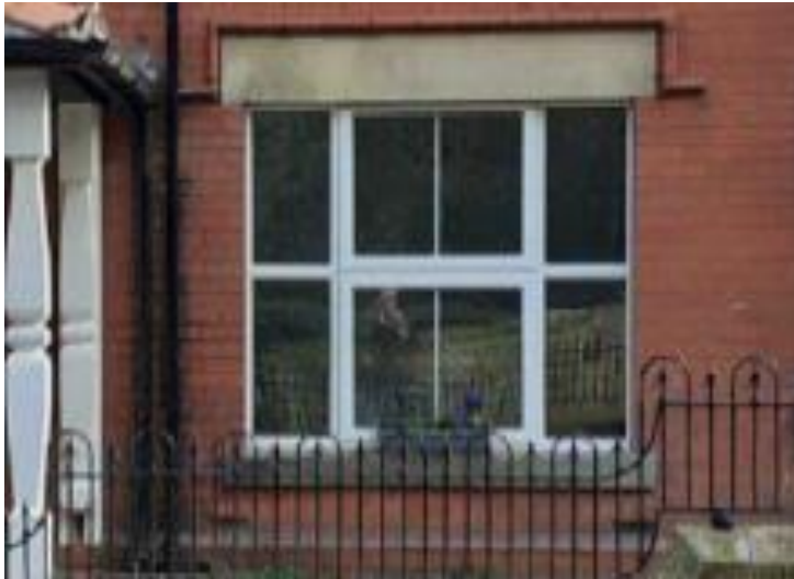
Window as installed
