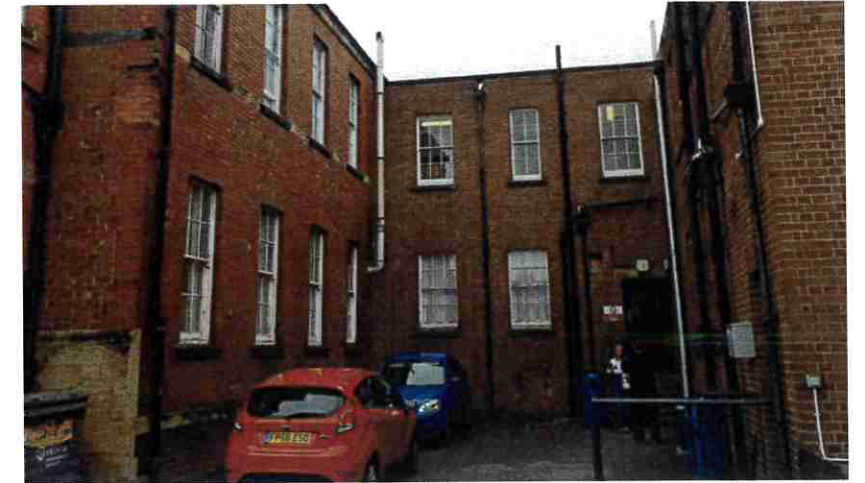
2. View of the existing courtyard
