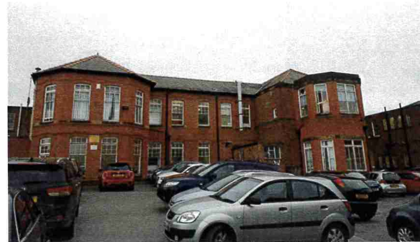
1. View of the existing building internal to the site
