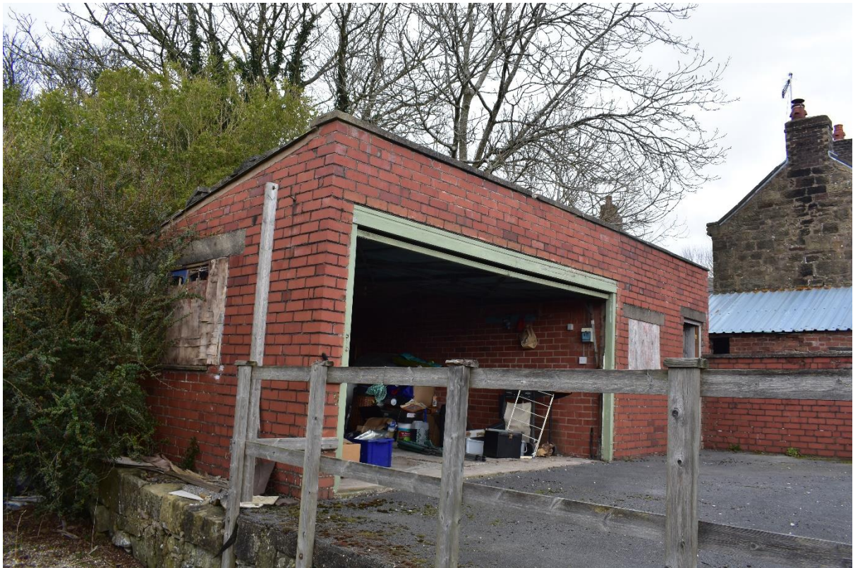
Figure 3.10: The single-pitched roof and the western section of the outbuilding to be removed.
