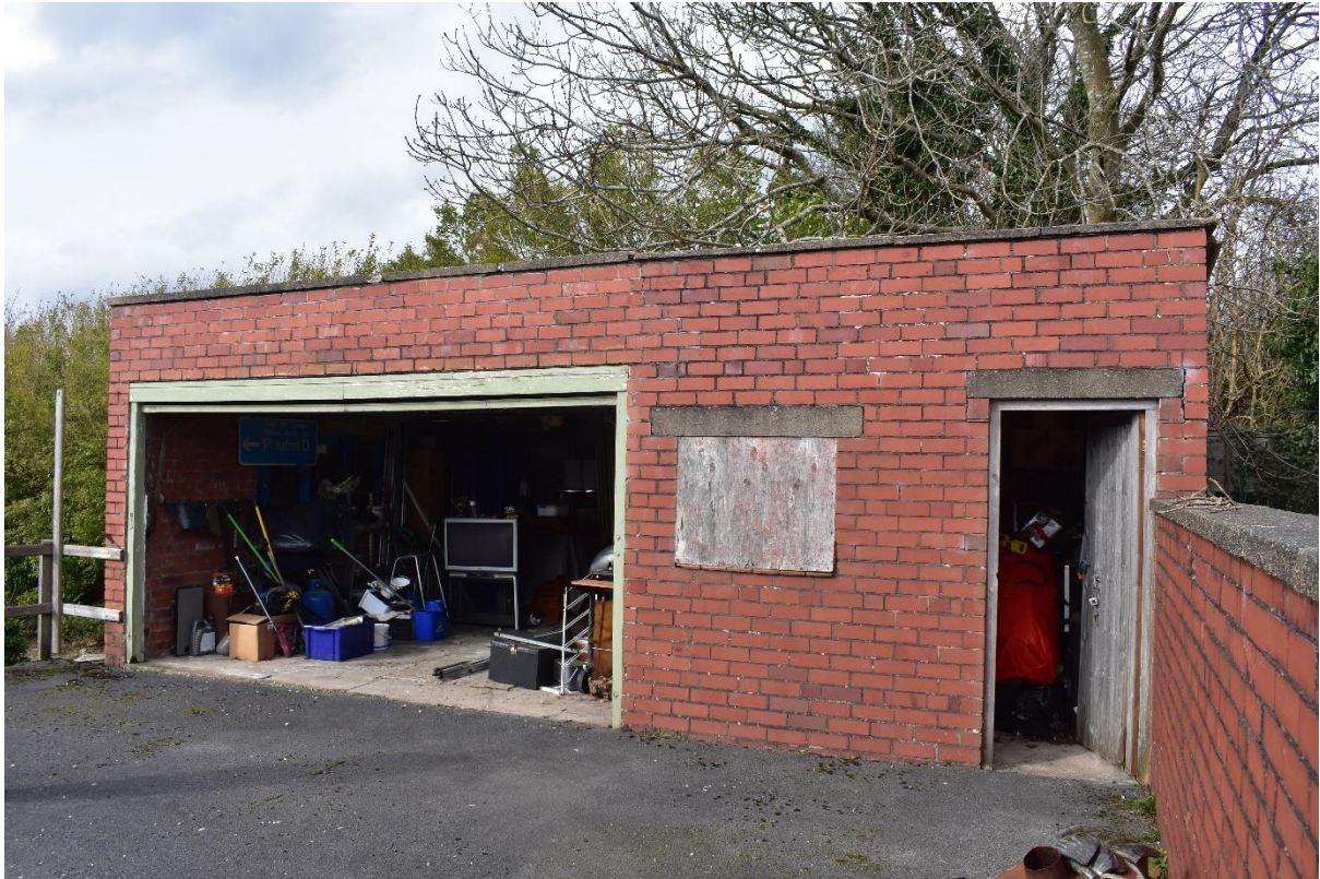
Figure 3.9: The front (south-facing) aspect of the outbuilding to be removed.
