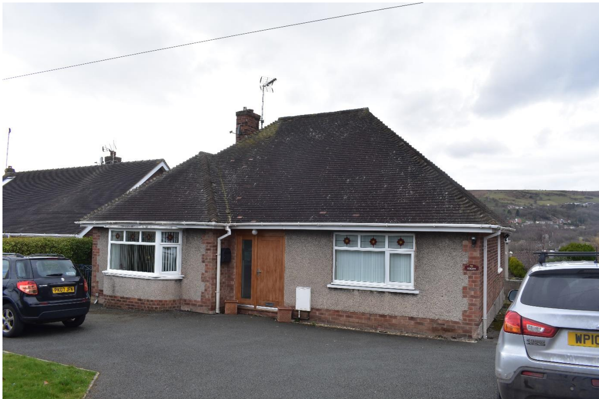
Figure 3.2: The front (east-facing) aspect of the dwelling.
