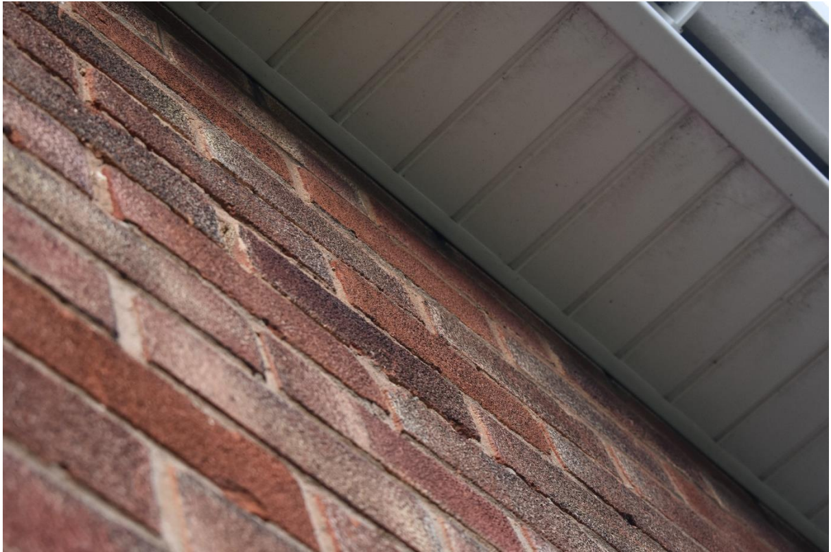
Figure 3.5: The tightly fitted soffits of the dwelling.
