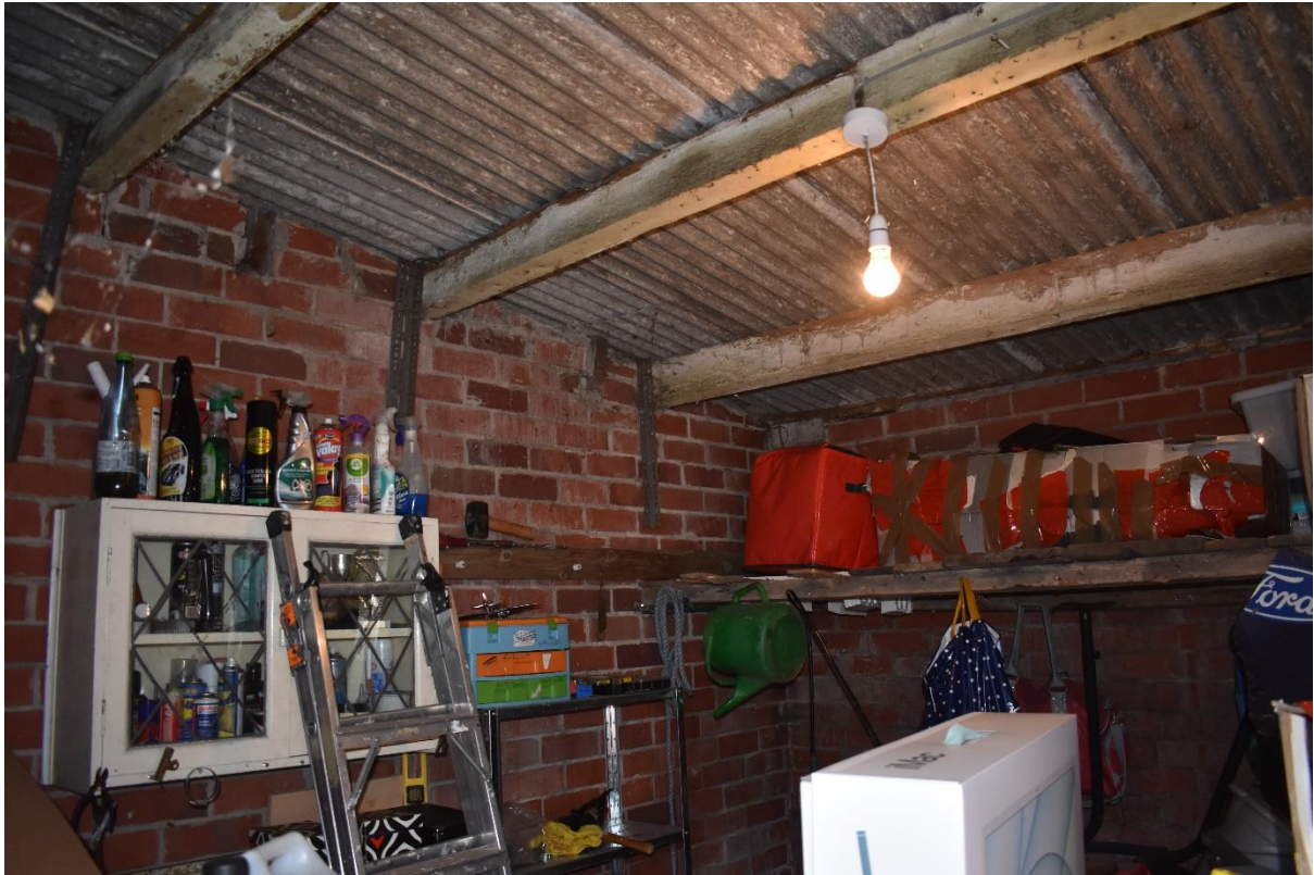
Figure 3.11: The interior of the outbuilding to be removed.
