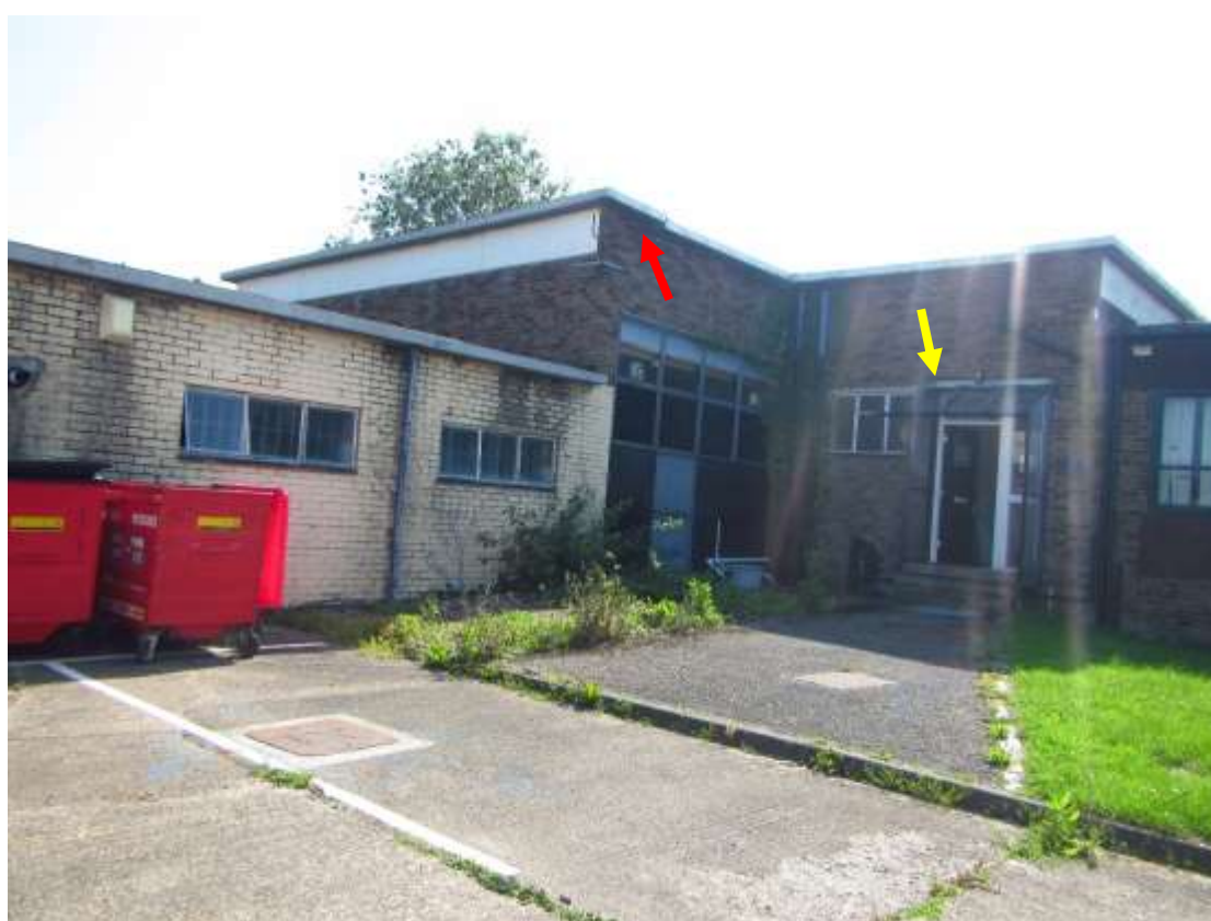
Photograph 4 – Red arrow shows location of gap in brickwork. Yellow arrow shows the location of Roost 1; beneath the lead flashing of the porch.
