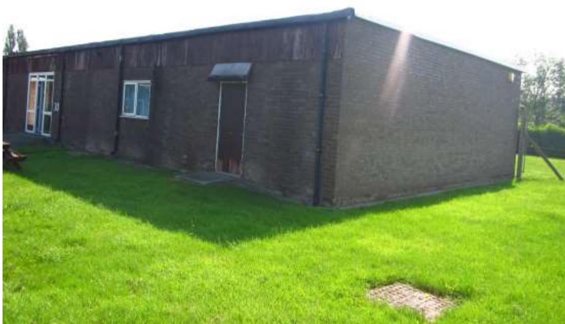
Photograph 2 – Southern aspect of Building 1.
