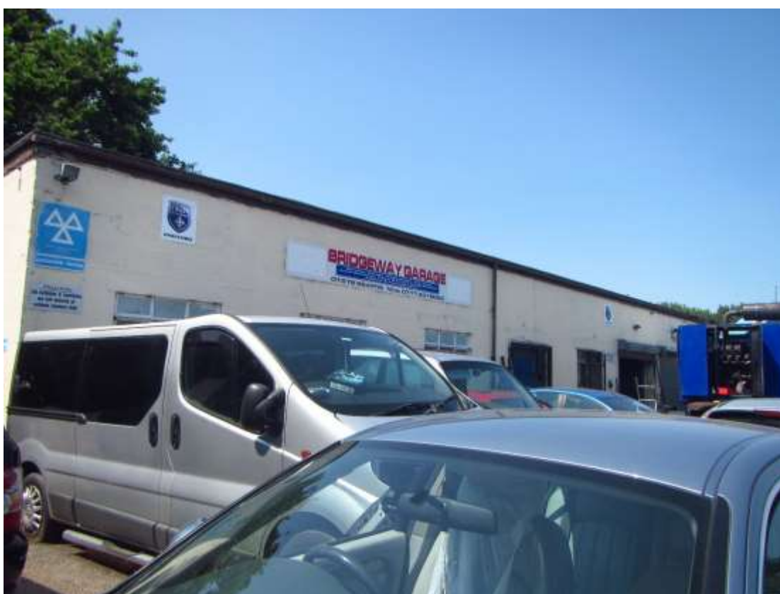
Photograph 24 – Northern aspect of Building 9.
