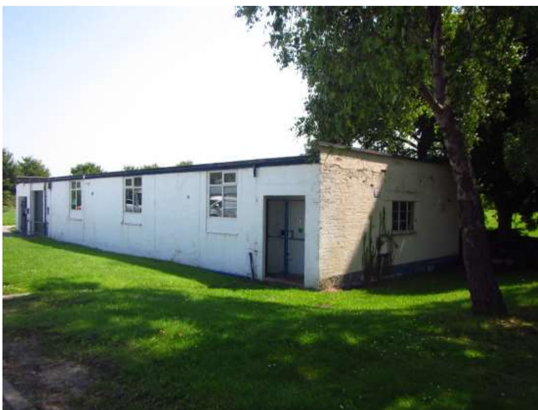
Photograph 22 - Southern and western aspect of Building 6.
