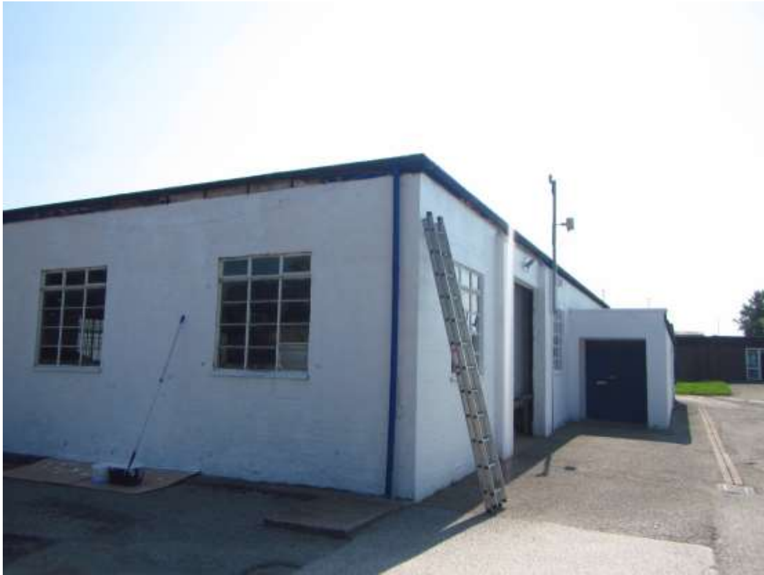
Photograph 11 – Western and southern aspect of Building 2.
