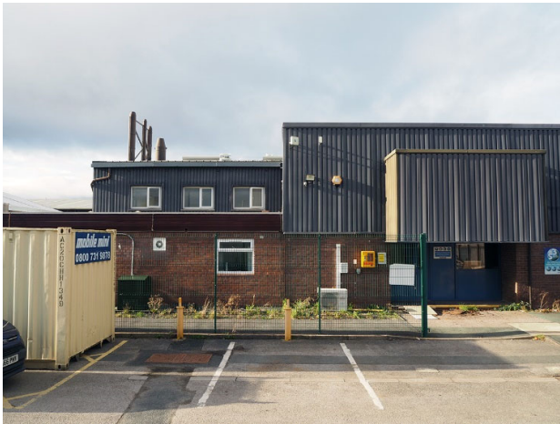
Figure 5 east facade, showing single story portion and portico to be removed
