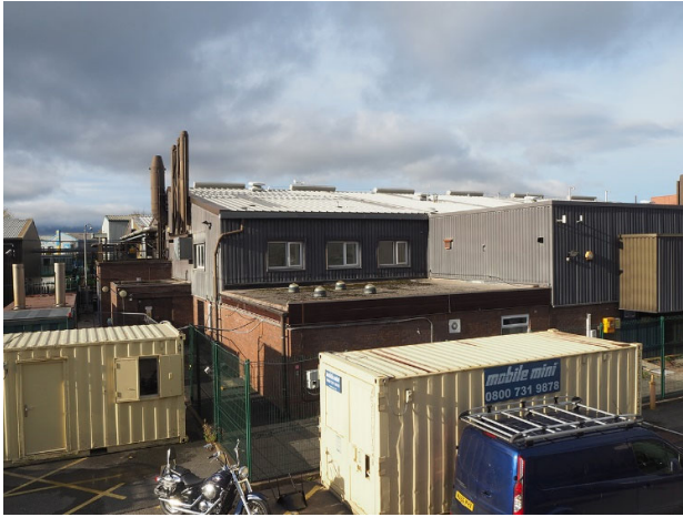
Figure 4 View of existing building from southeast
