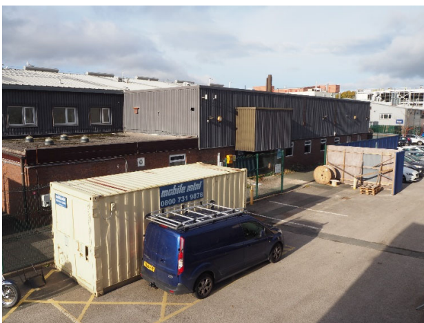
Figure 6 view of east facade
