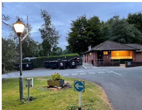
Photograph 1. Lighting levels and 3m lighting column at north-east corner of existing toilet block at dusk (August 2021)
