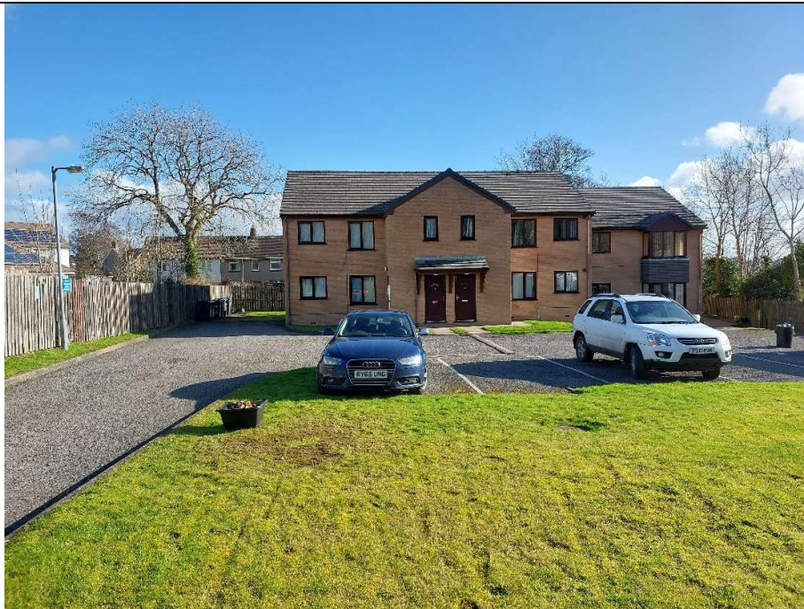
Photograph 8 – Facing east at the existing building and parking area
