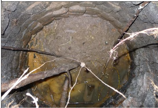
C21. Interior of well at Lion Lane Farm [full of earth, with small patch of water to one side].
