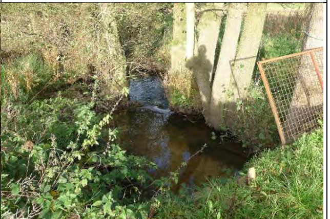
C18. Trees blocking stream downstream of footbridge.
