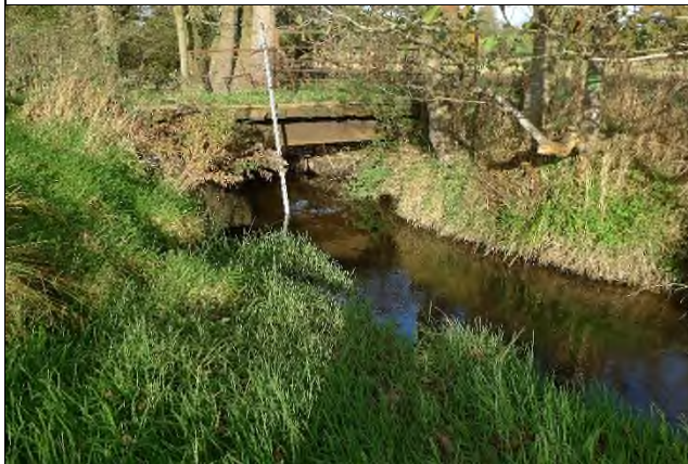
C17. Flow gauging point 2, upstream side of footbridge [view looking downstream].
