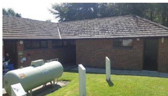
Photograph 2. North-west aspect of toilet block, with bathroom windows and doors.
