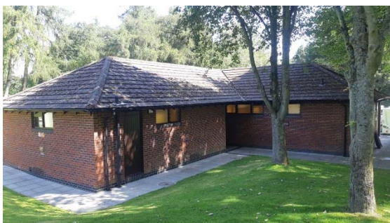
Photograph 1. Rear aspect of the existing toilet block.
