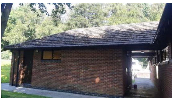
Photograph 1. Southern aspect of adjoining annexe, with connecting corridor.
