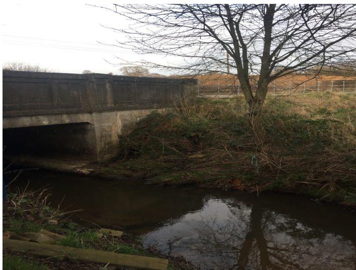
Picture 1: indicates the existing culvert, associated banks and A539.
