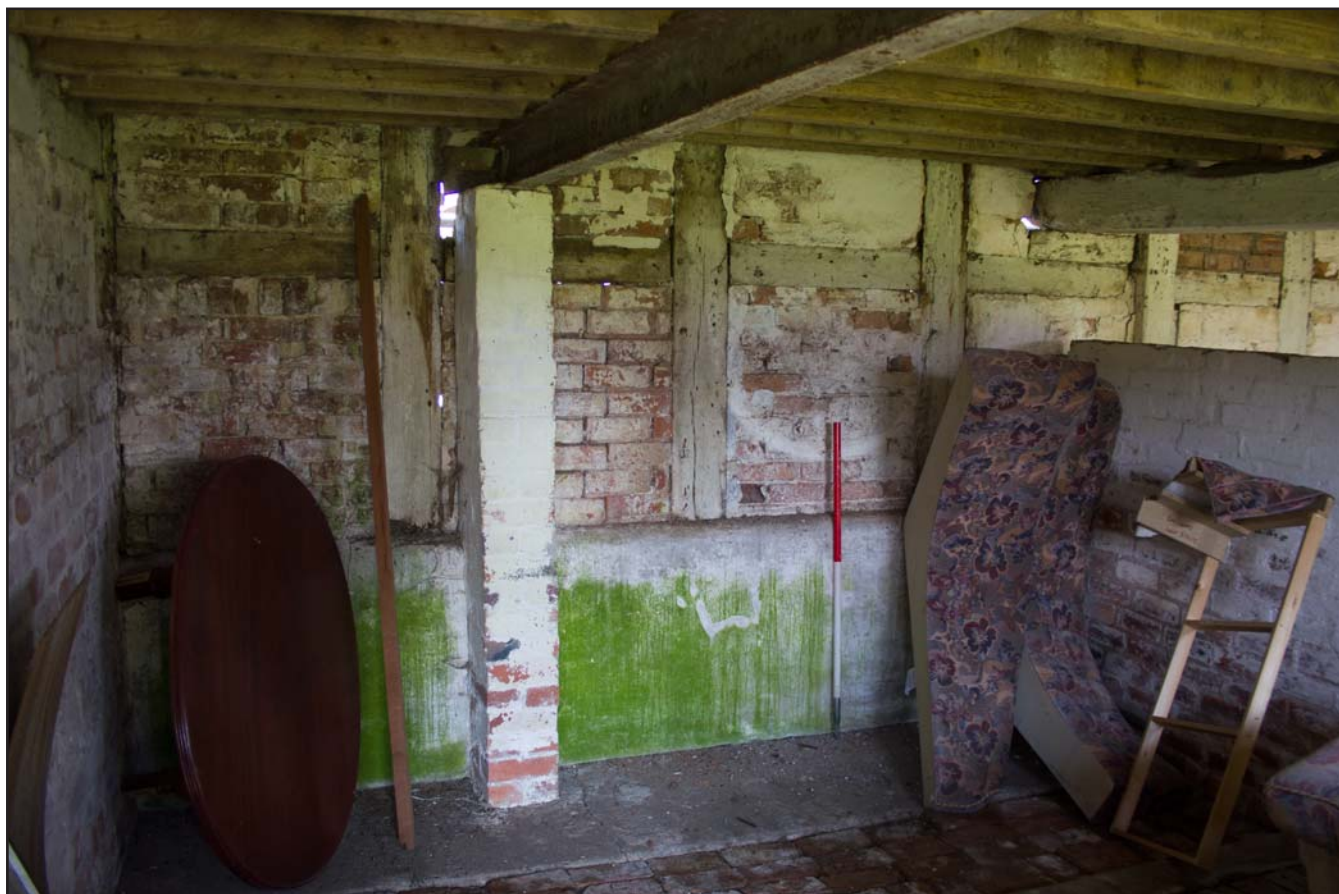
Plate 45: Room 2, ground floor, Shippon 1 at Brunette Farm, Ty Broughton, Wrexham - from the east - scale 1m
