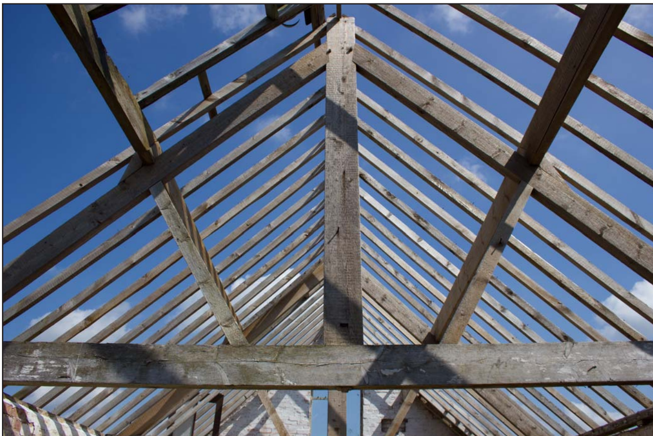
Plate 90: Kingspost truss within Shippon 3 at Brunette Farm, Ty Broughton, Wrexham - from the southwest - no scale
