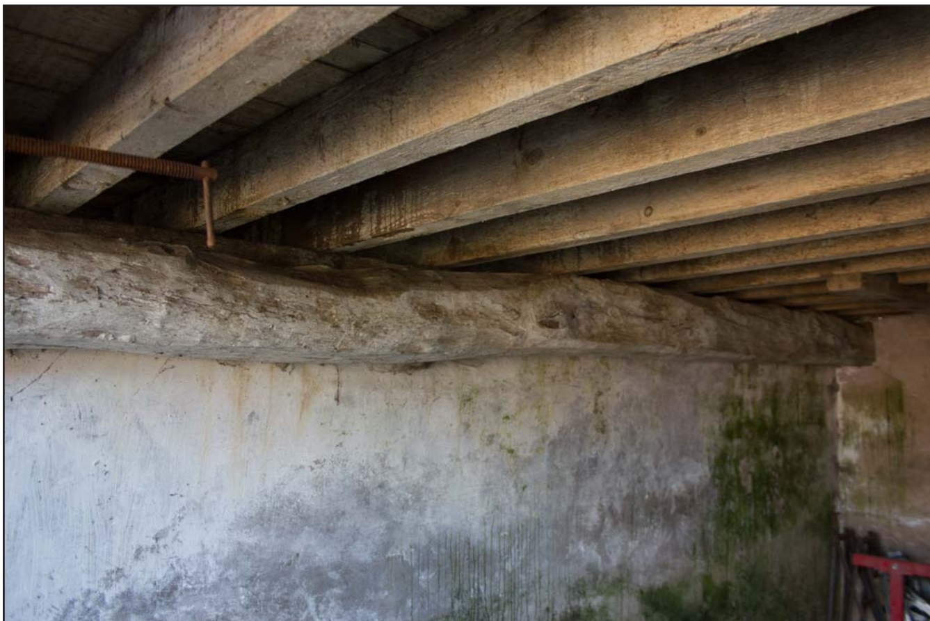
Plate 49: Handhewn beam within Room 4, ground floor, Shippon 1 at Brunette Farm, Ty Broughton, Wrexham - from the west - scale 1m
