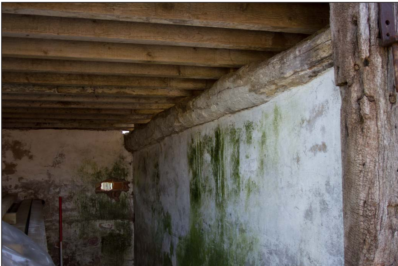
Plate 51: Handhewn beam within Room 5, ground floor, Shippon 1 at Brunette Farm, Ty Broughton, Wrexham - from the north - scale 1m
