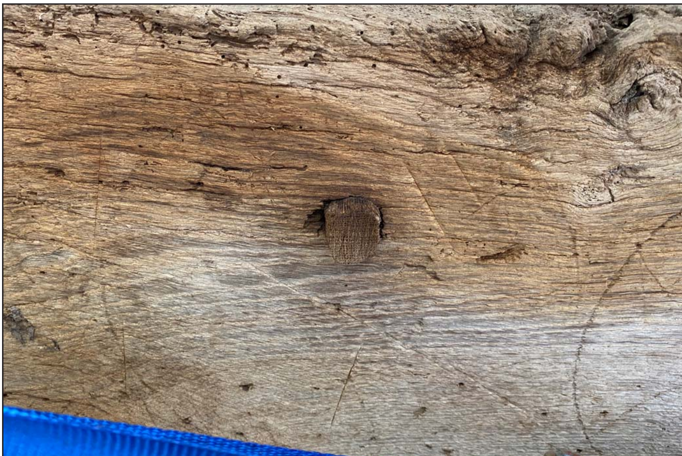
Plate 68: Apotropaic Mark, Hexafoil 'Daisy-Wheel' on southeast side of handhewn tie beam of Truss 2, within Shippon 1 at Brunette Farm, Ty Broughton, Wrexham - from the southwest - no scale
