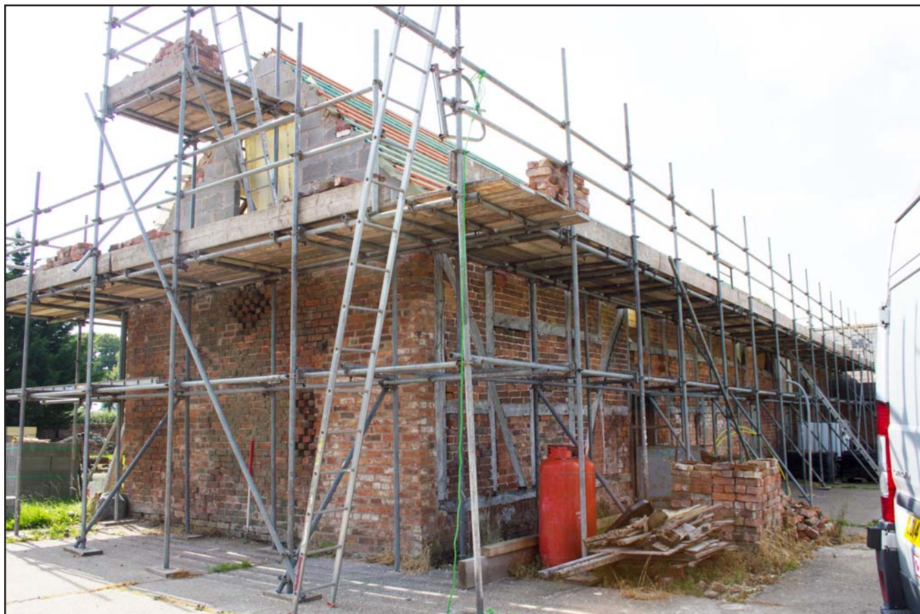
Plate 37: Northwest and northeast elevations of Shippon 1 at Brunette Farm, Ty Broughton, Wrexham - from the north - scale 1m
