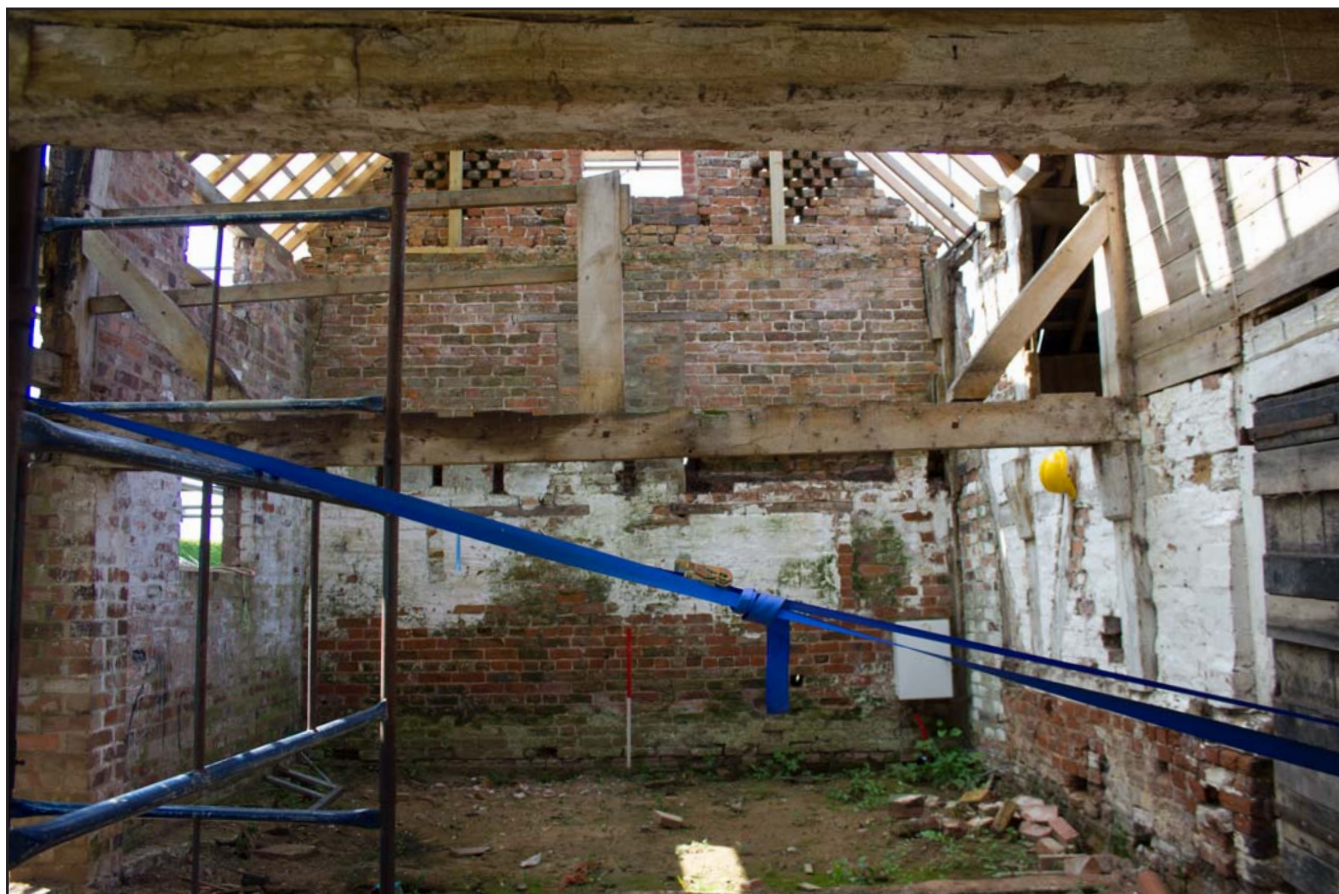
Plate 52: Room 6, ground floor, Shippon 1 at Brunette Farm, Ty Broughton, Wrexham - from the northeast - scale 1m
