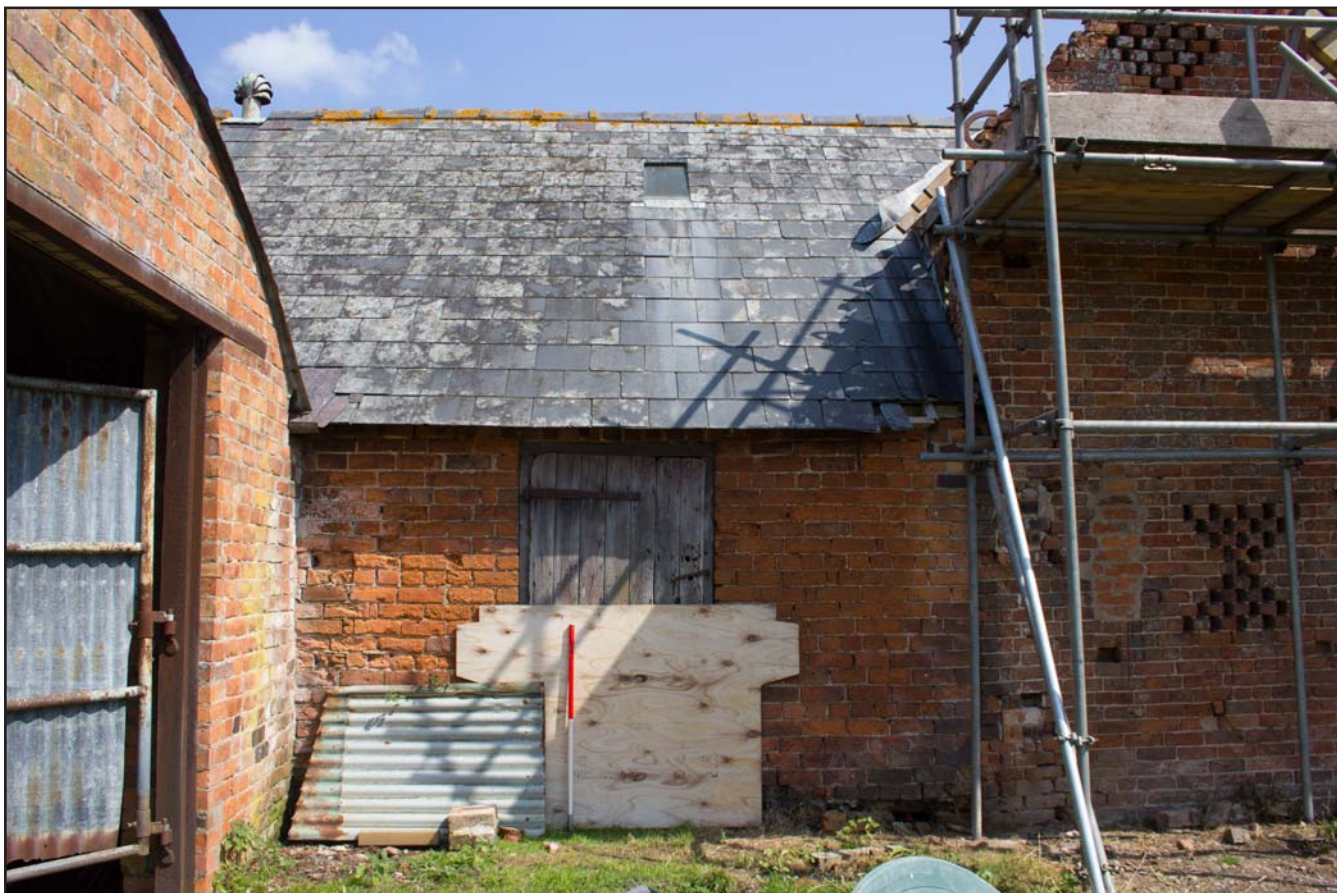
Plate 78: Southwest facing elevation of Shippon 2 at Brunette Farm, Ty Broughton, Wrexham - from the southwest - 1m scale
