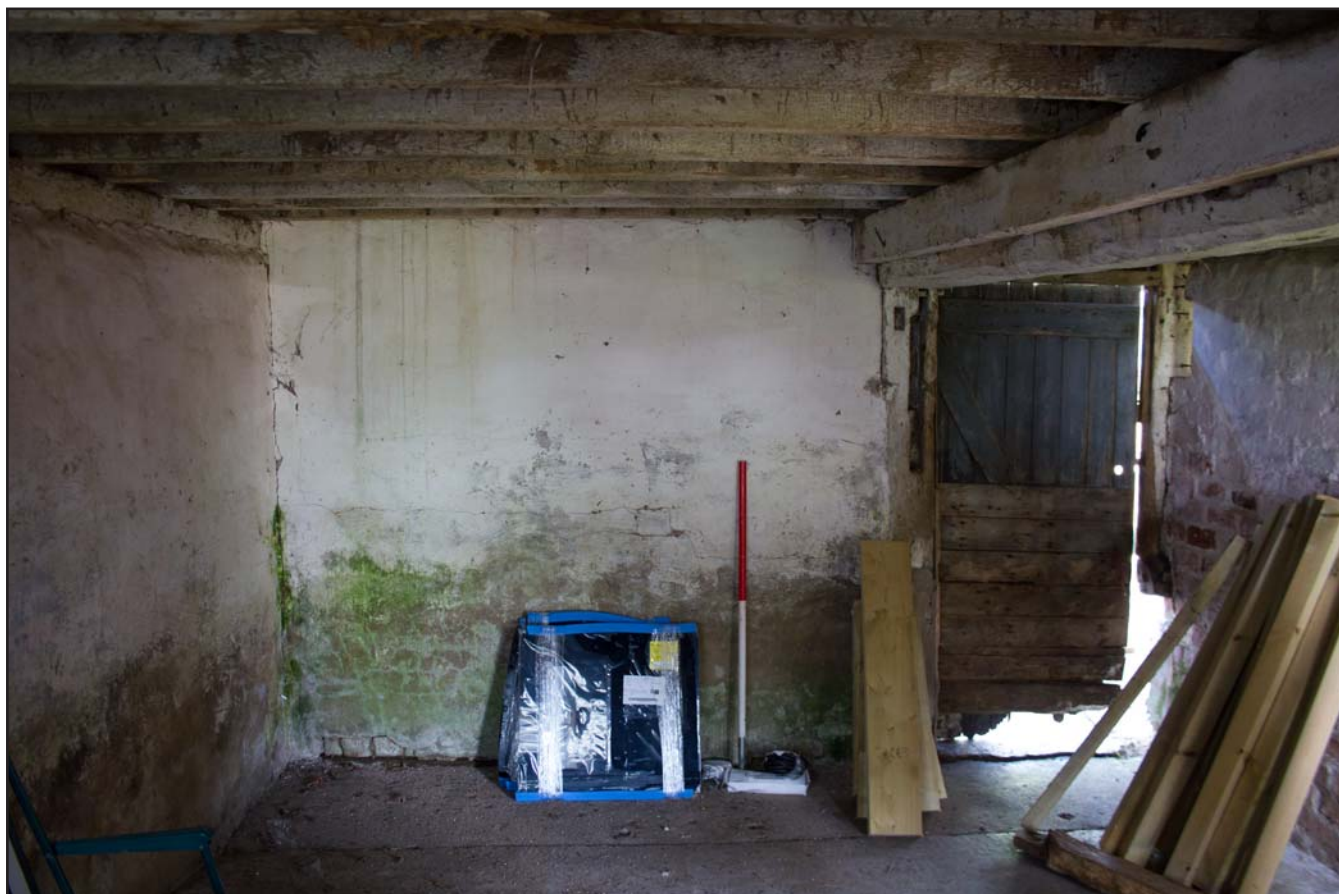
Plate 46: Room 3, ground floor, Shippon 1 at Brunette Farm, Ty Broughton, Wrexham - from the southeast - scale 1m
