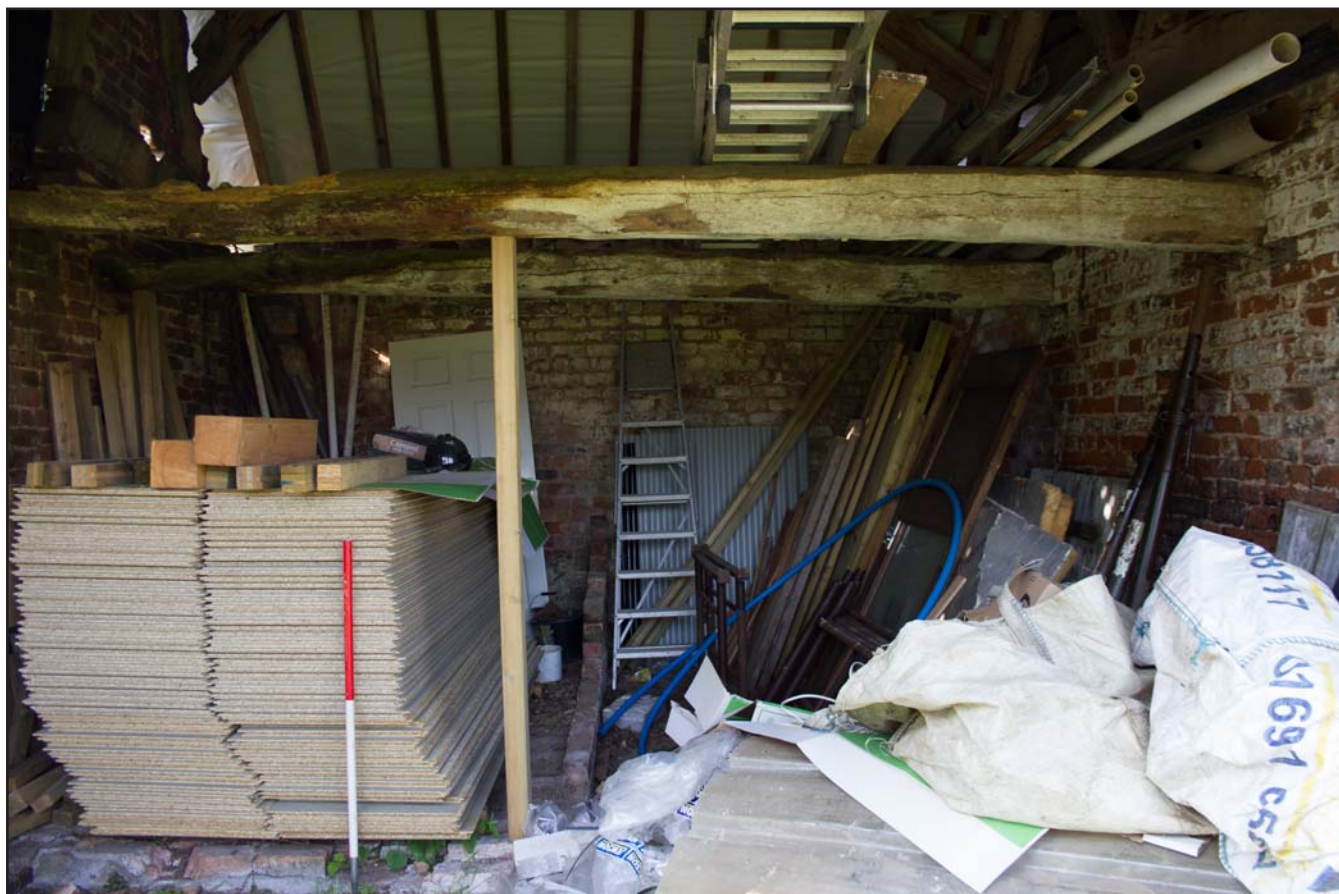
Plate 12: Room 1 within the Stable at Brunette Farm, Ty Broughton, Wrexham - from the northeast - scale 1m
