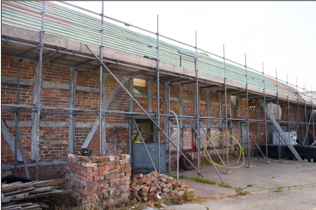
Plate 36: Oblique shot of northwest elevation of Shippon 1 at Brunette Farm, Ty Broughton, Wrexham - from the west - scale 1m
