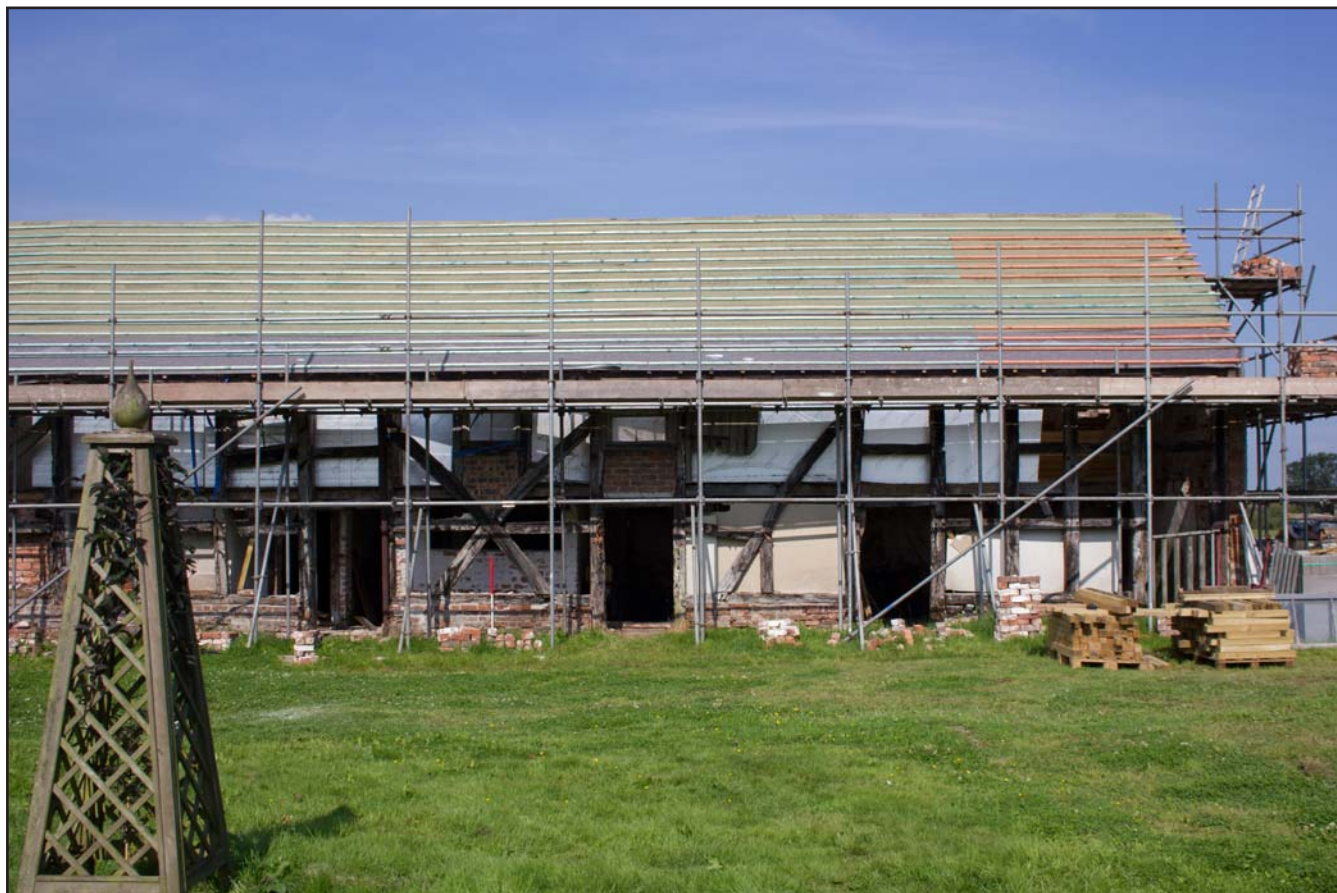
Plate 26: Right hand end of southeast elevation of Shippon 1 at Brunette Farm, Ty Broughton, Wrexham - from the southeast - scale 1m
