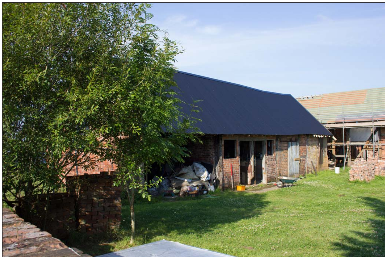
Plate 02: Oblique shot of northeast facing elevation of the Stable at Brunette Farm, Ty Broughton, Wrexham - from the east - scale 1m
