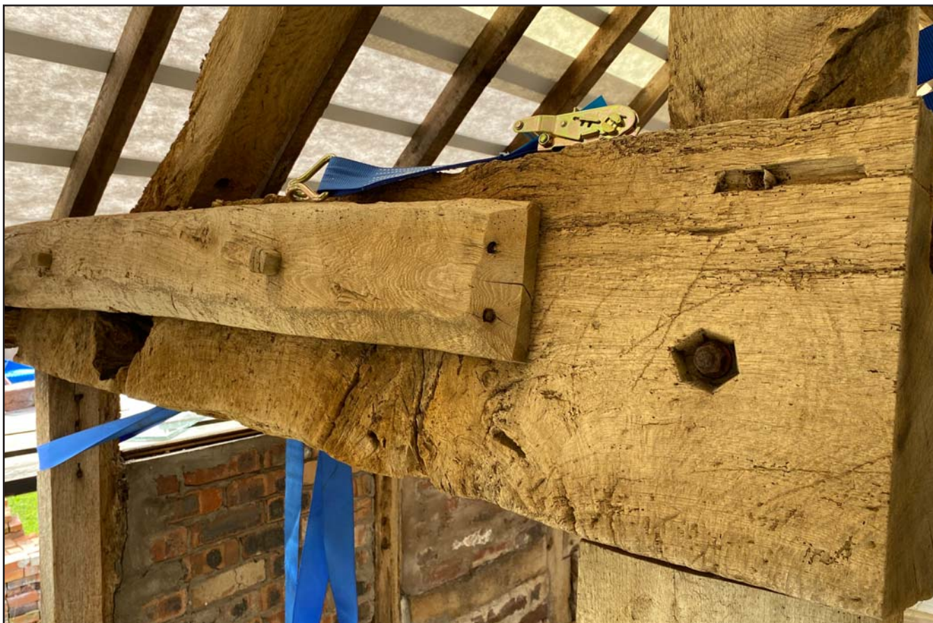
Plate 75: Possible faint Apotropaic Marks on northwest side of handhewn tie beam: Marian & Hexafoil? Truss 2, within Shippon 1 at Brunette Farm, Ty Broughton, Wrexham - from the southwest - no scale
