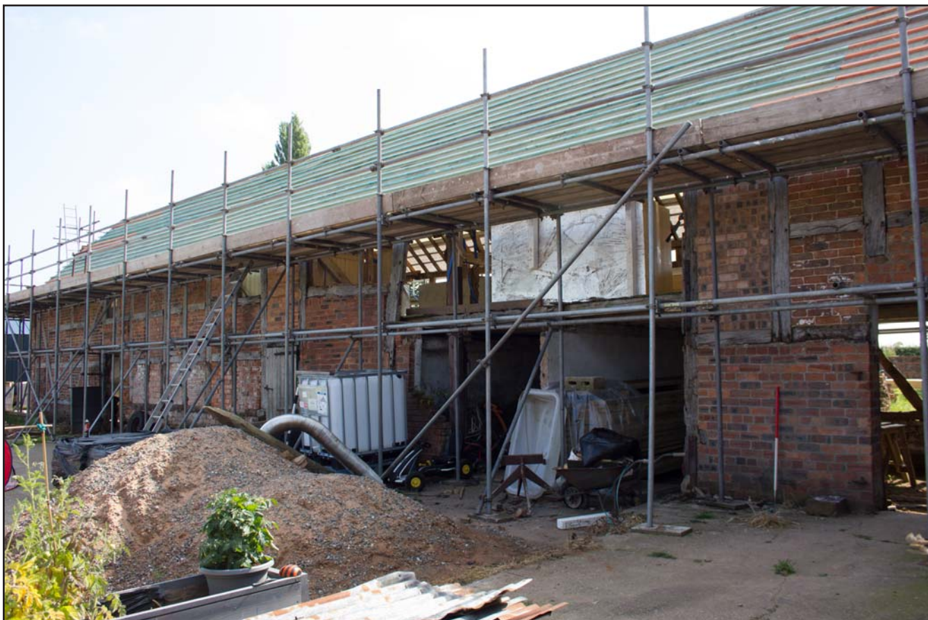
Plate 32: Oblique shot of northwest elevation of Shippon 1 at Brunette Farm, Ty Broughton, Wrexham - from the west - scale 1m
