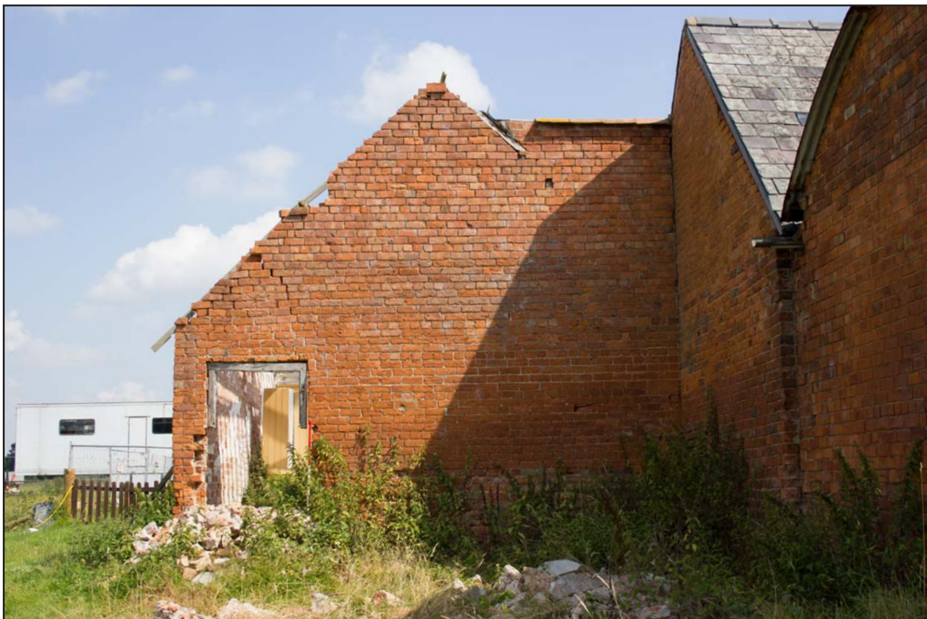
Plate 87: Southwest facing elevation of Shippon 3 at Brunette Farm, Ty Broughton, Wrexham - from the southwest - scale 1m
