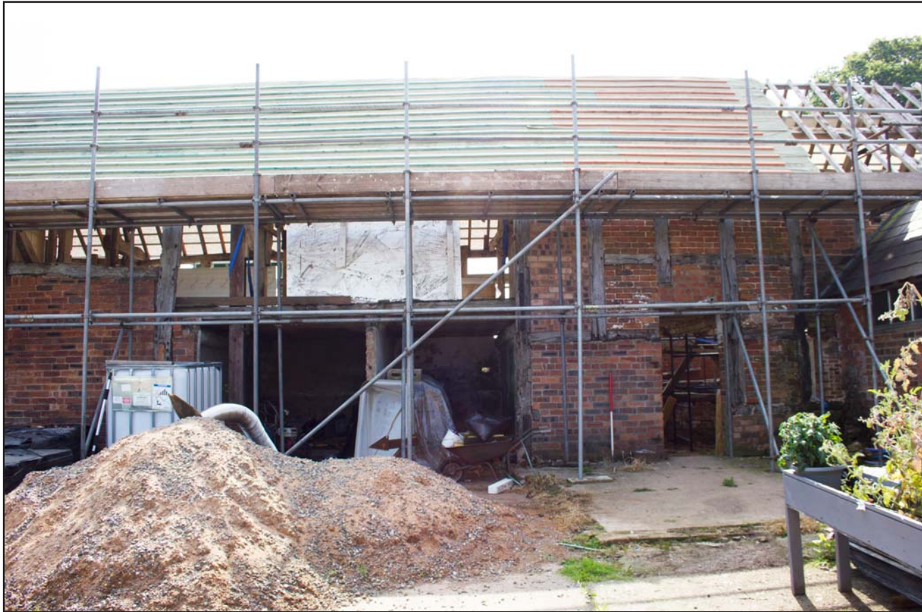
Plate 33: Right hand end of northwest elevation of Shippon 1 at Brunette Farm, Ty Broughton, Wrexham - from the northwest - scale 1m
