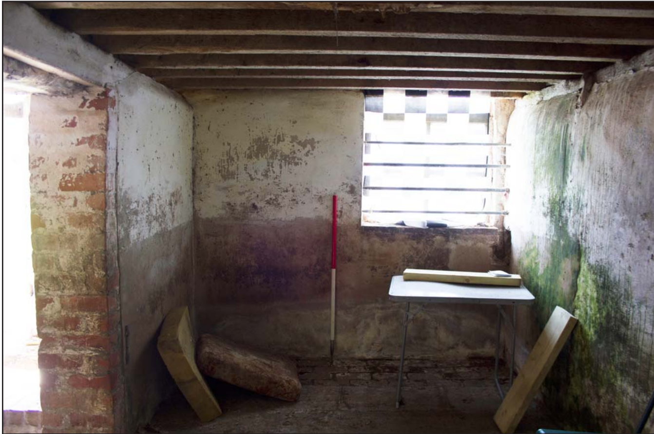
Plate 47: Room 3, ground floor, Shippon 1 at Brunette Farm, Ty Broughton, Wrexham - from the northwest - scale 1m
