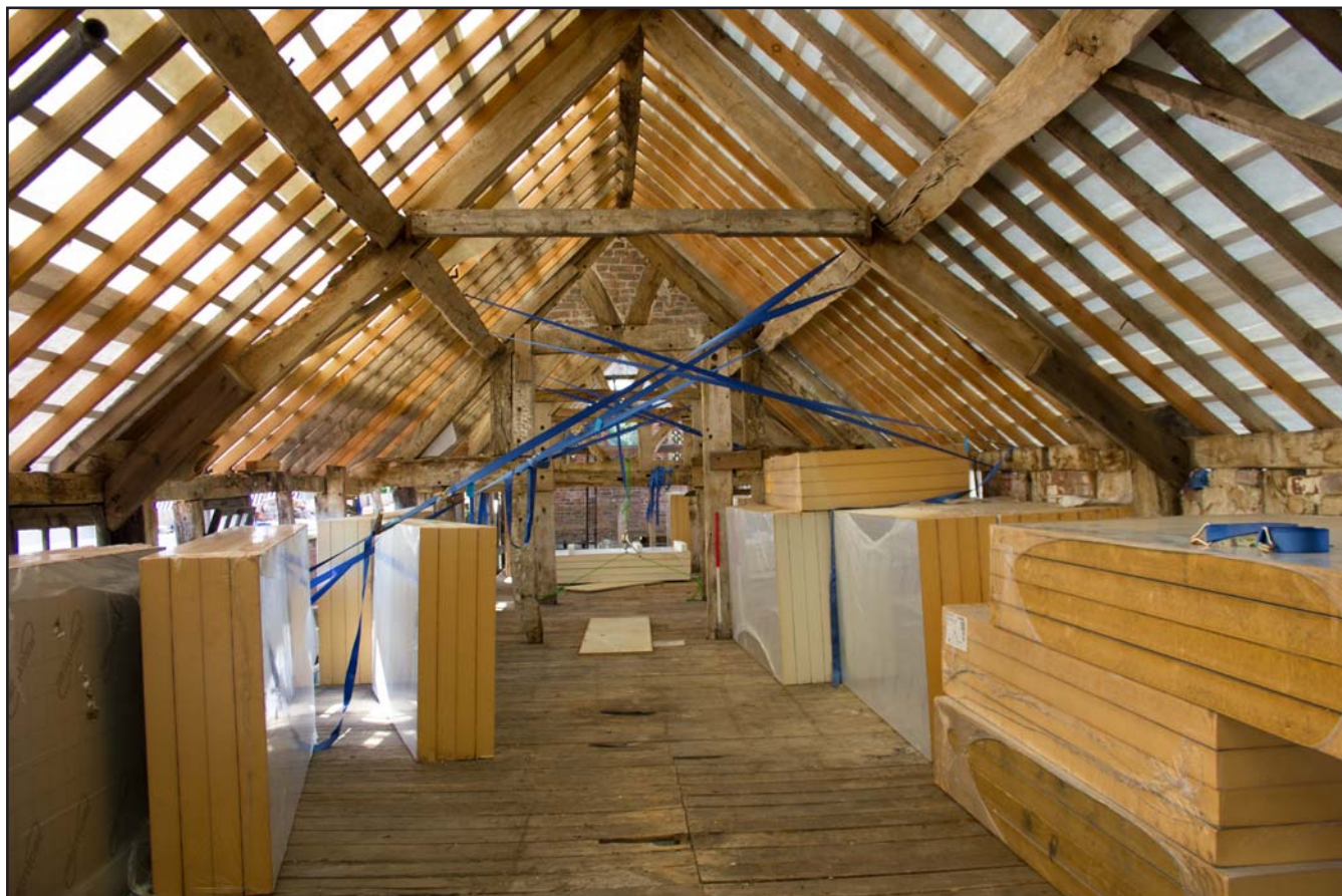
Plate 56: First floor, Shippon 1 at Brunette Farm, Ty Broughton, Wrexham - from the northeast - scale 1m
