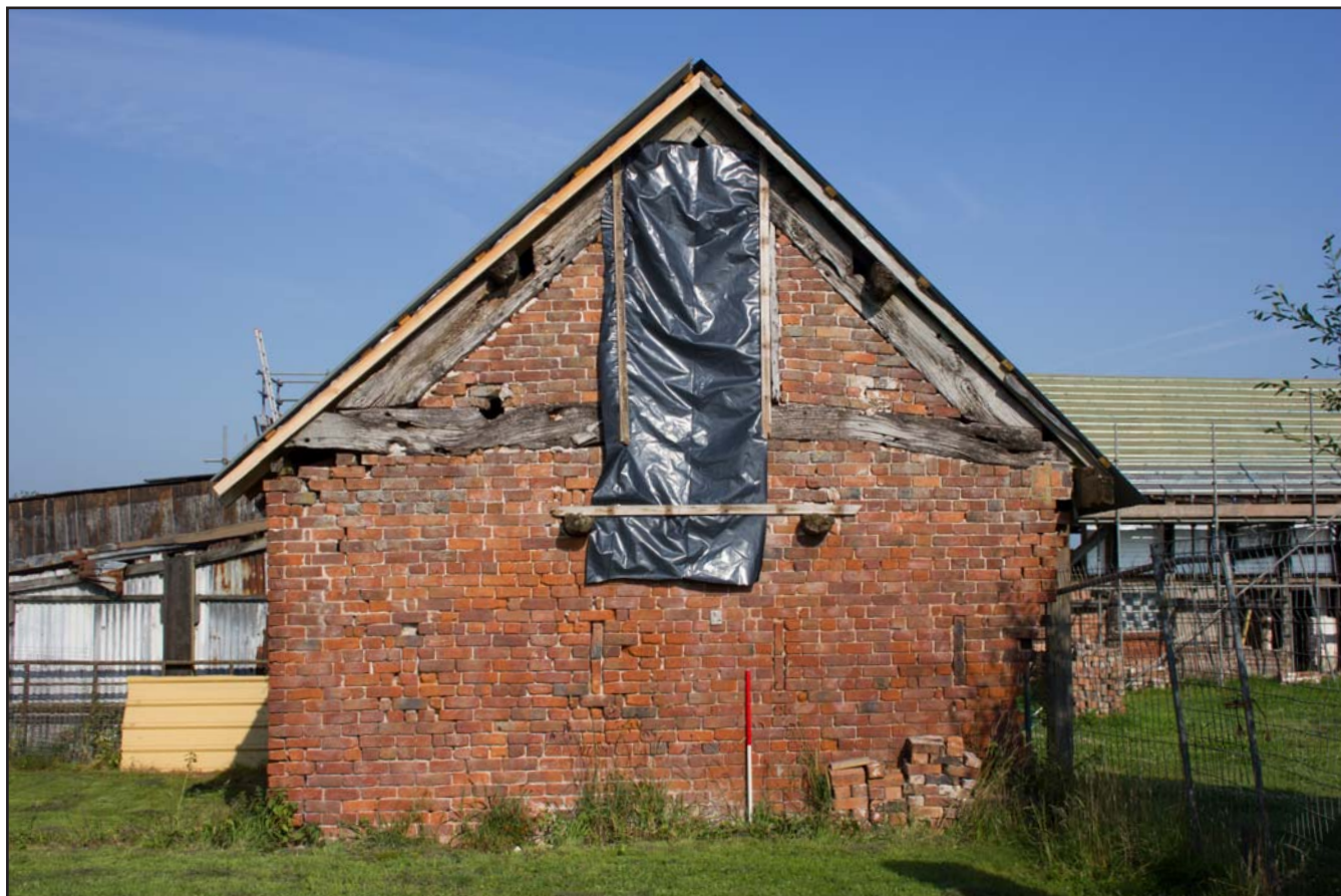
Plate 03: Southeast facing gable elevation of the Stable at Brunette Farm, Ty Broughton, Wrexham - from the southeast - scale 1m
