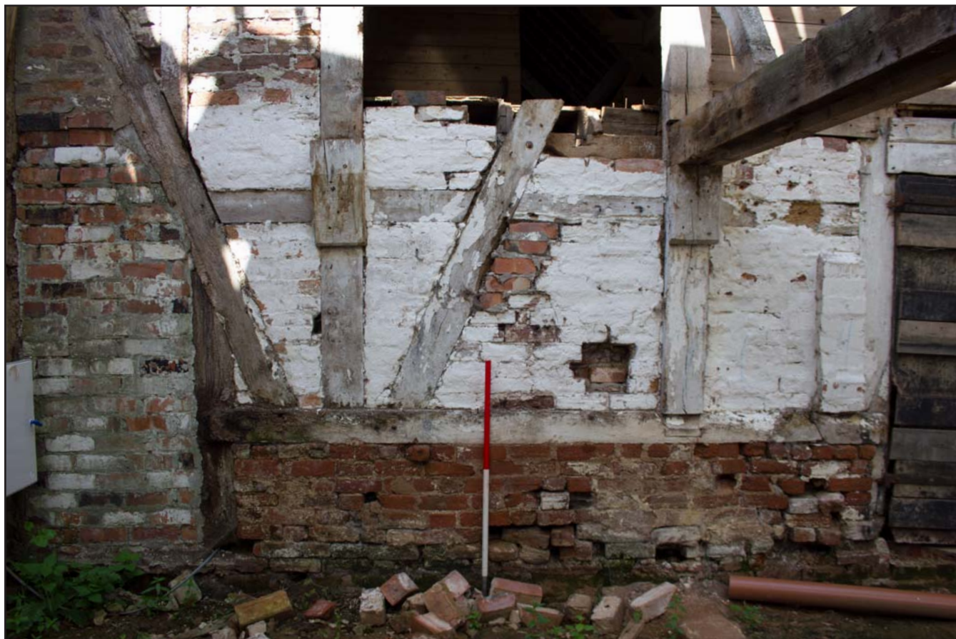
Plate 55: Northwest elevation within Room 6, ground floor, Shippon 1 at Brunette Farm, Ty Broughton, Wrexham - from the southeast - scale 1m
