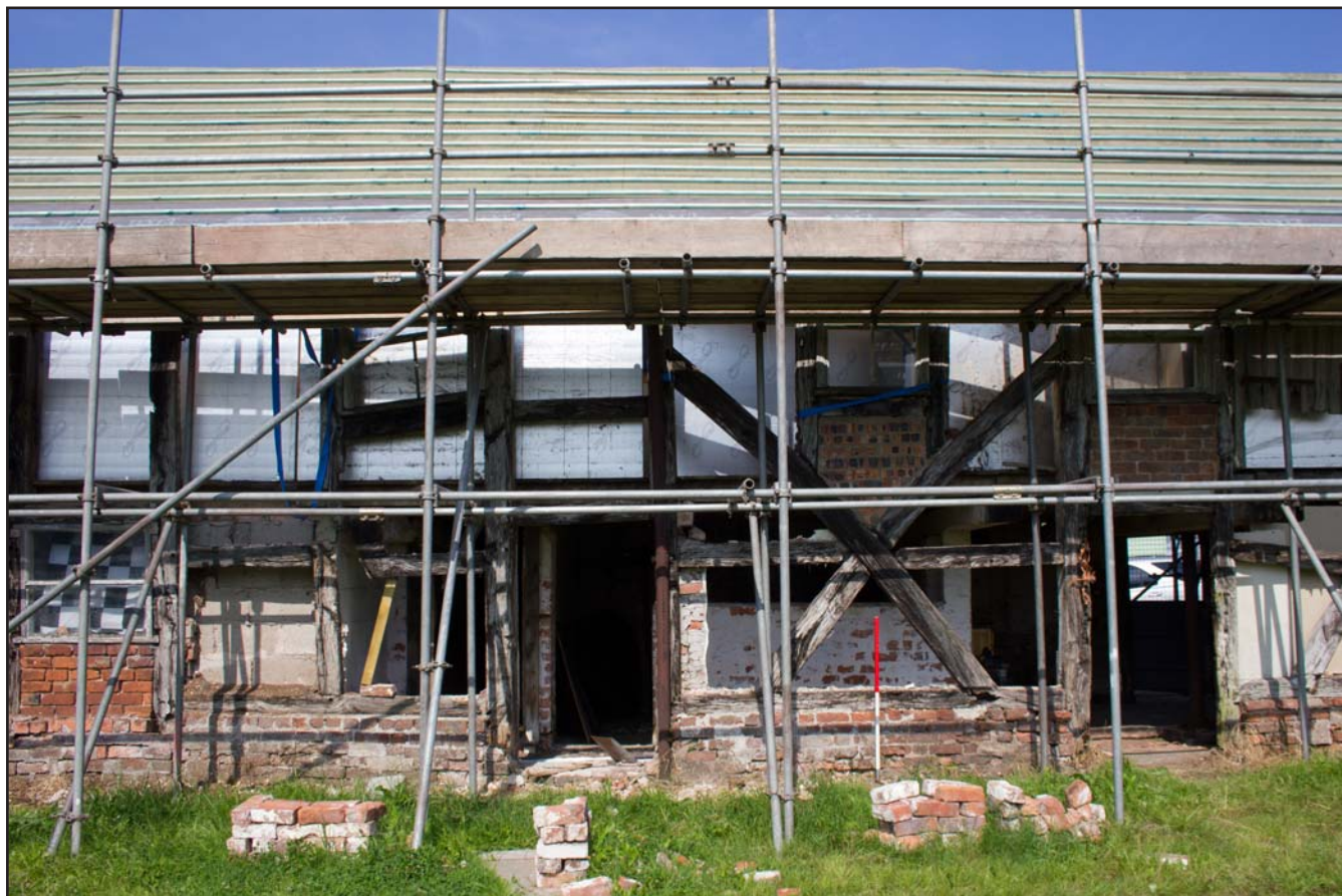
Plate 28: Centre of southeast elevation of Shippon 1 at Brunette Farm, Ty Broughton, Wrexham - from the southeast - scale 1m
