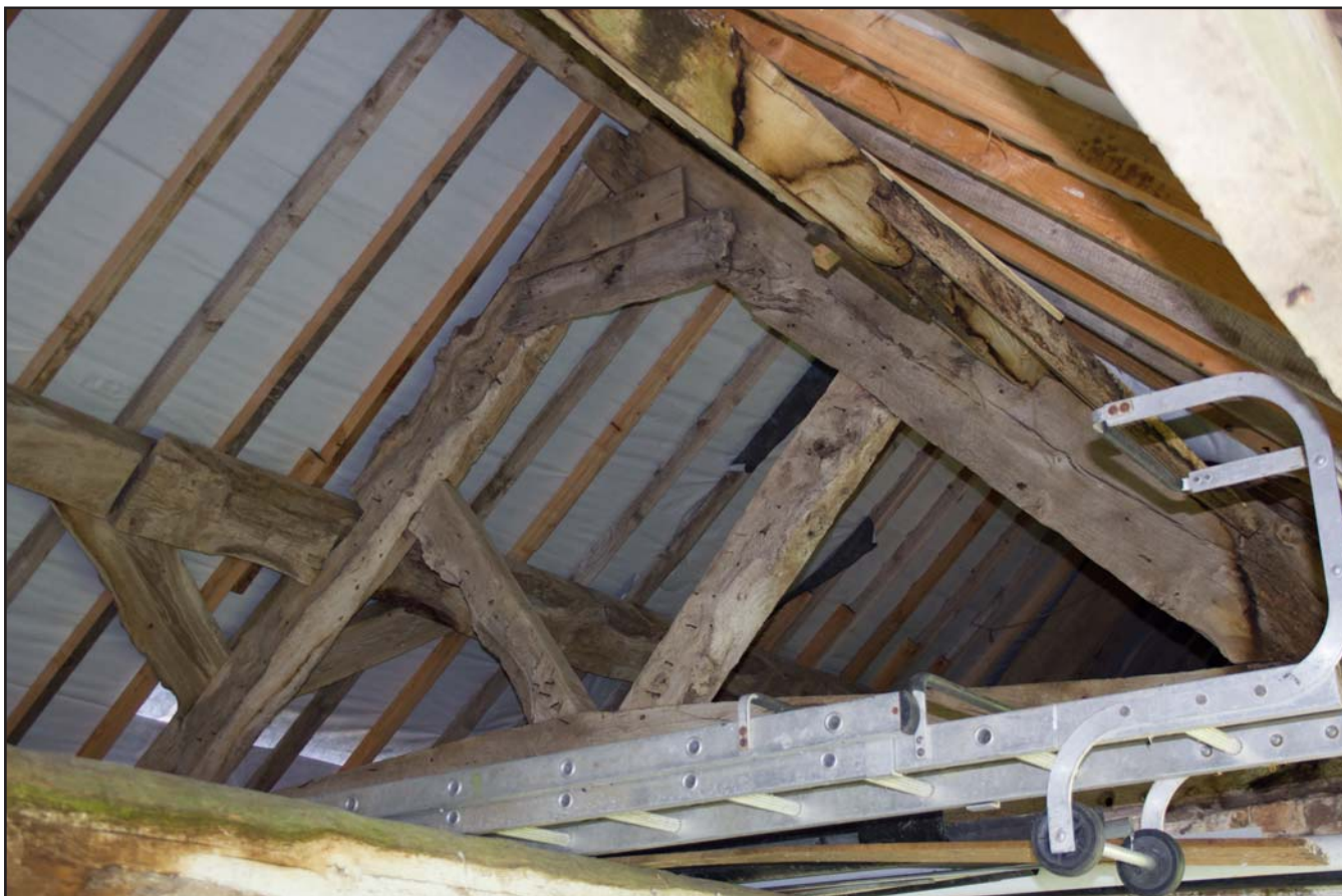
Plate 14: North western handhewn truss and blades in Room 1, Stable at Brunette Farm, Ty Broughton, Wrexham - from the east - no scale
