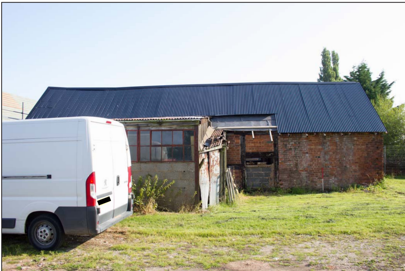
Plate 05: Southwest facing elevation of the Stable at Brunette Farm, Ty Broughton, Wrexham - from the southwest - scale 1m
