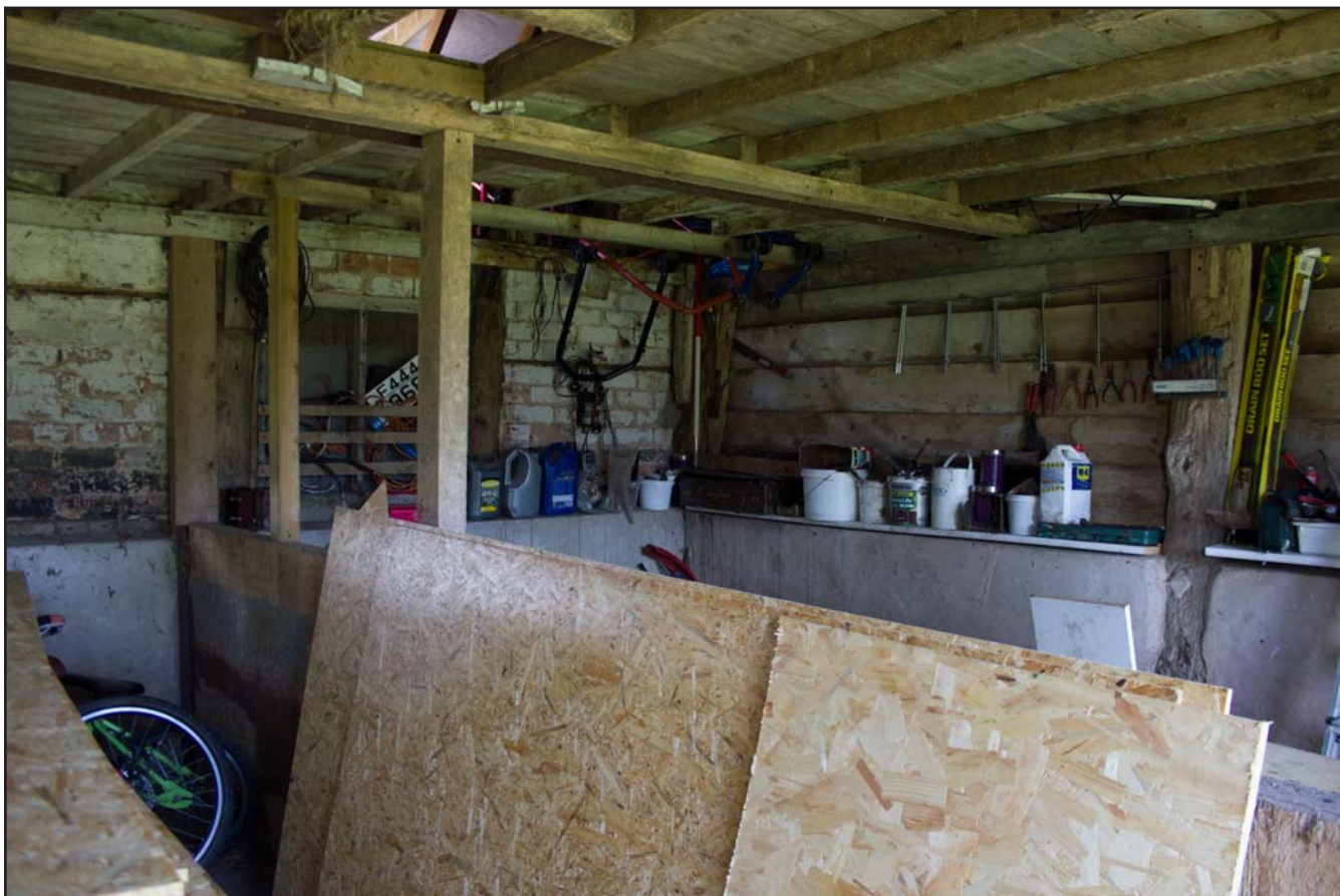
Plate 16: Room 2 within the Stable at Brunette Farm, Ty Broughton, Wrexham - from the east - scale 1m
