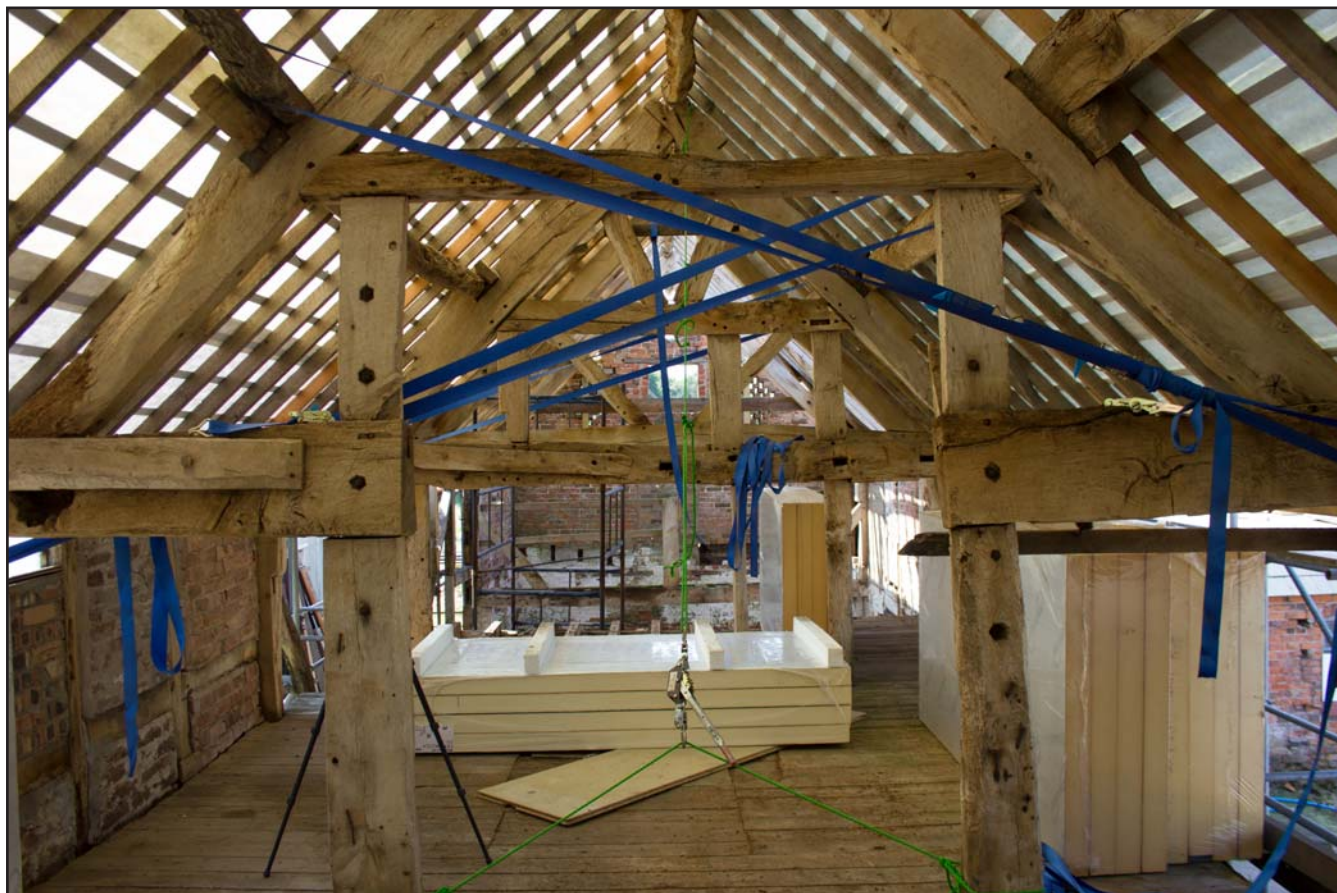
Plate 58: Truss 2, First floor, Shippon 1 at Brunette Farm, Ty Broughton, Wrexham - from the northeast - no scale
