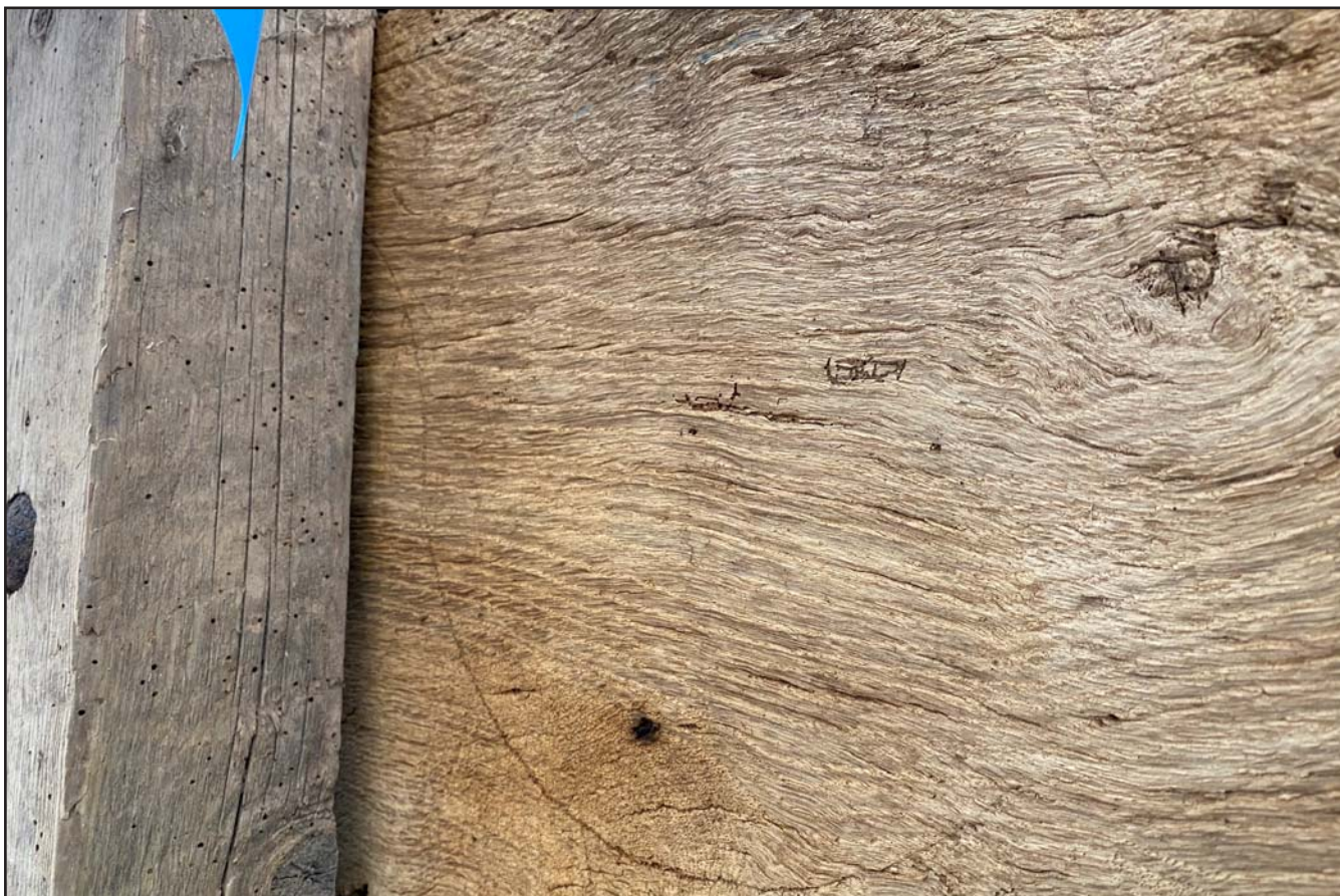
Plate 69: Apotropaic Mark, Hexafoil 'Daisy-Wheel' on southeast side of handhewn tie beam of Truss 2, within Shippon 1 at Brunette Farm, Ty Broughton, Wrexham - from the southwest - no scale
