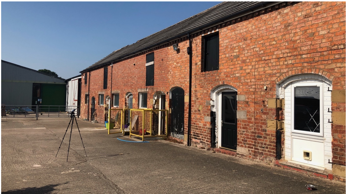
Figure 8 – View to site front
