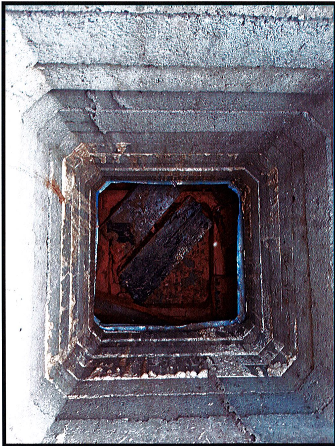
Photograph 2: Looking down shaft manhole, dipped at 2.20m
