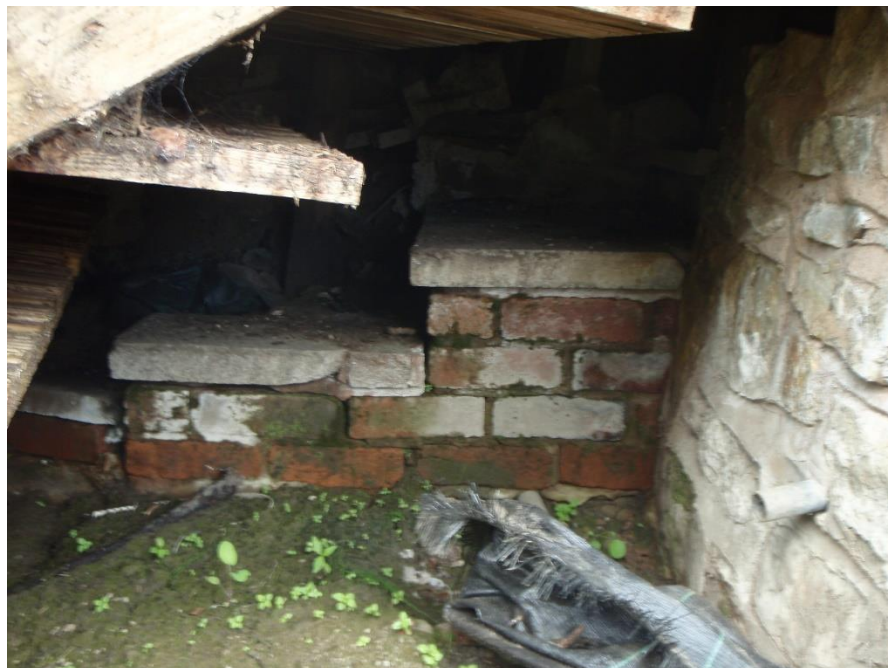
Defunct brick/ patio slab steps located underneath the raised wooded decking at Targe Note 2 .
