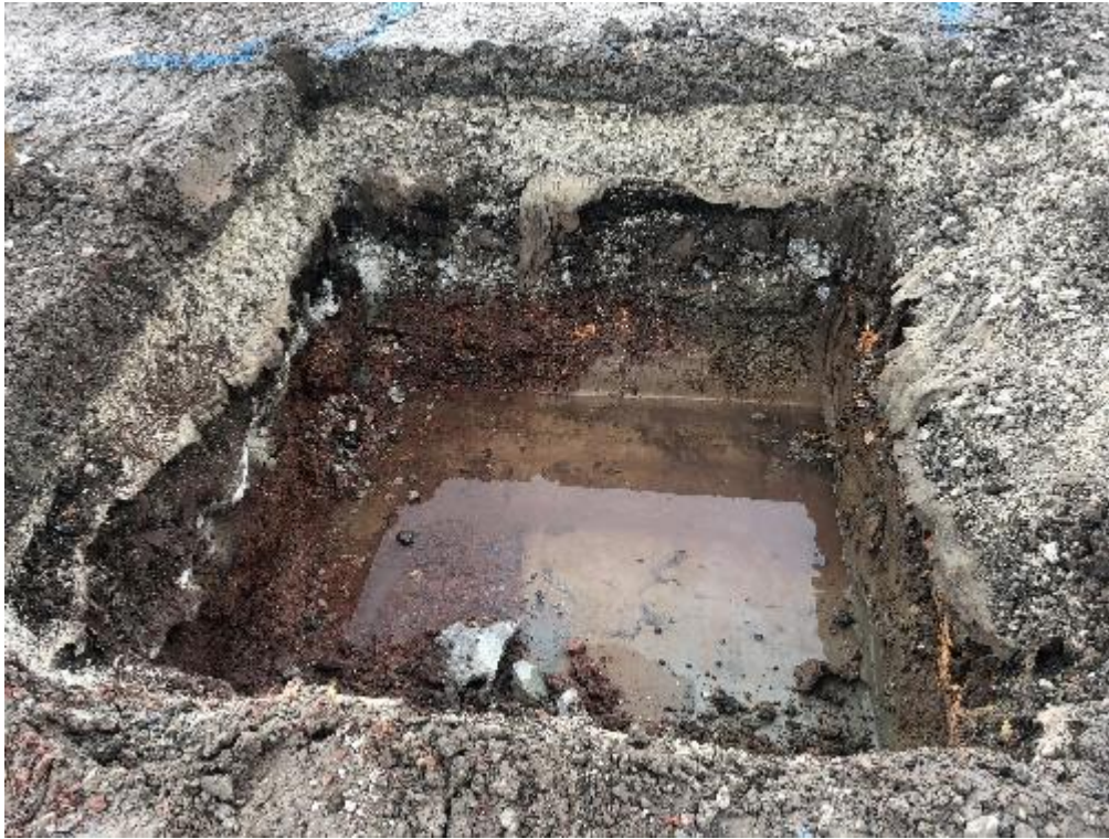
PLATE 1 GROUND CONDITIONS IN VICINITY OF FORMER POND SHWOING NO ORGANIC OF DELETRIOUS MATERIALS AND GENERAL MADE GROUND DEPOSITS
