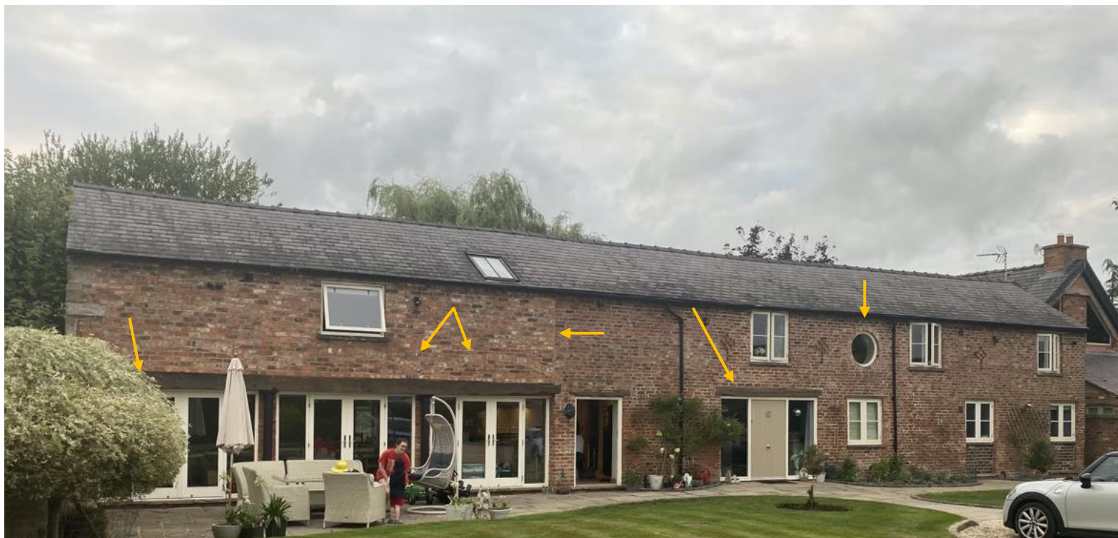
Fig 4. Existing front elevation - south-east (Copyright: Willacy Horsewood Architects). Note cart shed openings – the flat lintel is probably dating from the 1860's or later, note the straight join, the pitching holes and domestic cottage appearance. Including full length French doors.
