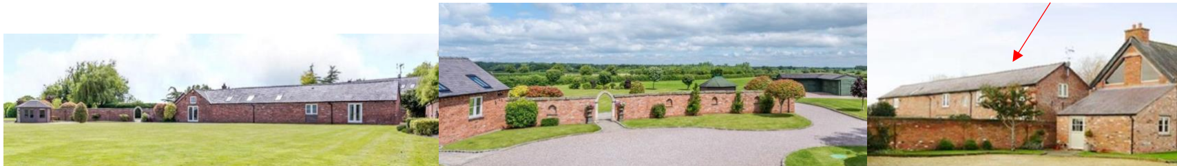
Fig 9. Former outbuildings to Trevalyn Farm, all converted to residential, with ancillary domestic structures and domestic windows and doors. Sandford Barn arrowed red.
