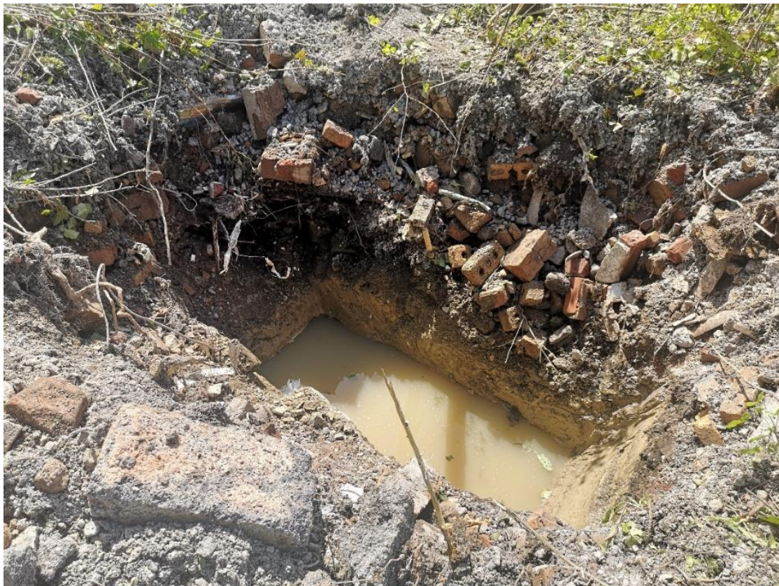
Figure 20 Engineer’s test pit with demolition debris and yellow clay subsoil. (photo D. Bailey).
