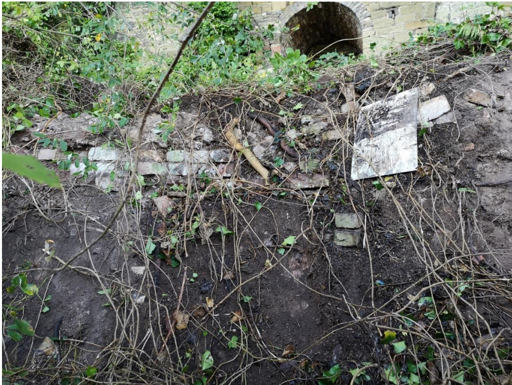
Figure 19 Fragment of brick wall at top of slope immediately behind palisade fence. (courtesy D. Bailey)
