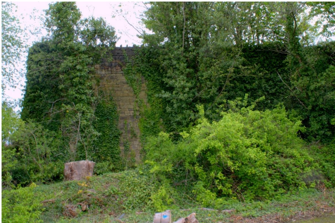
Figure 8 Revetment Wall at NE end of site, Llangollen Rd to left.
