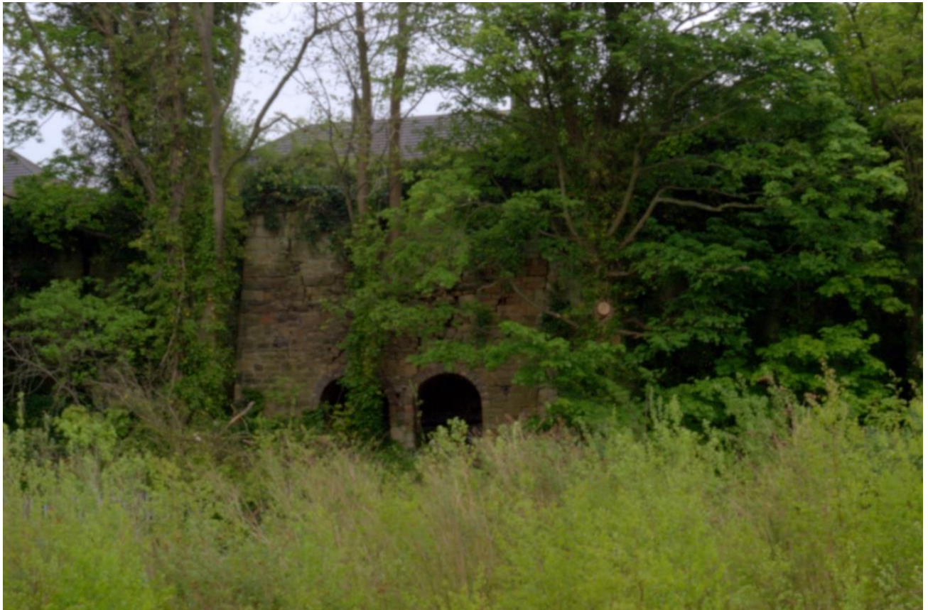
Figure 24. Phase 2 furnace. Phase 1 on right, joint behind tree to right of furnace arch.
