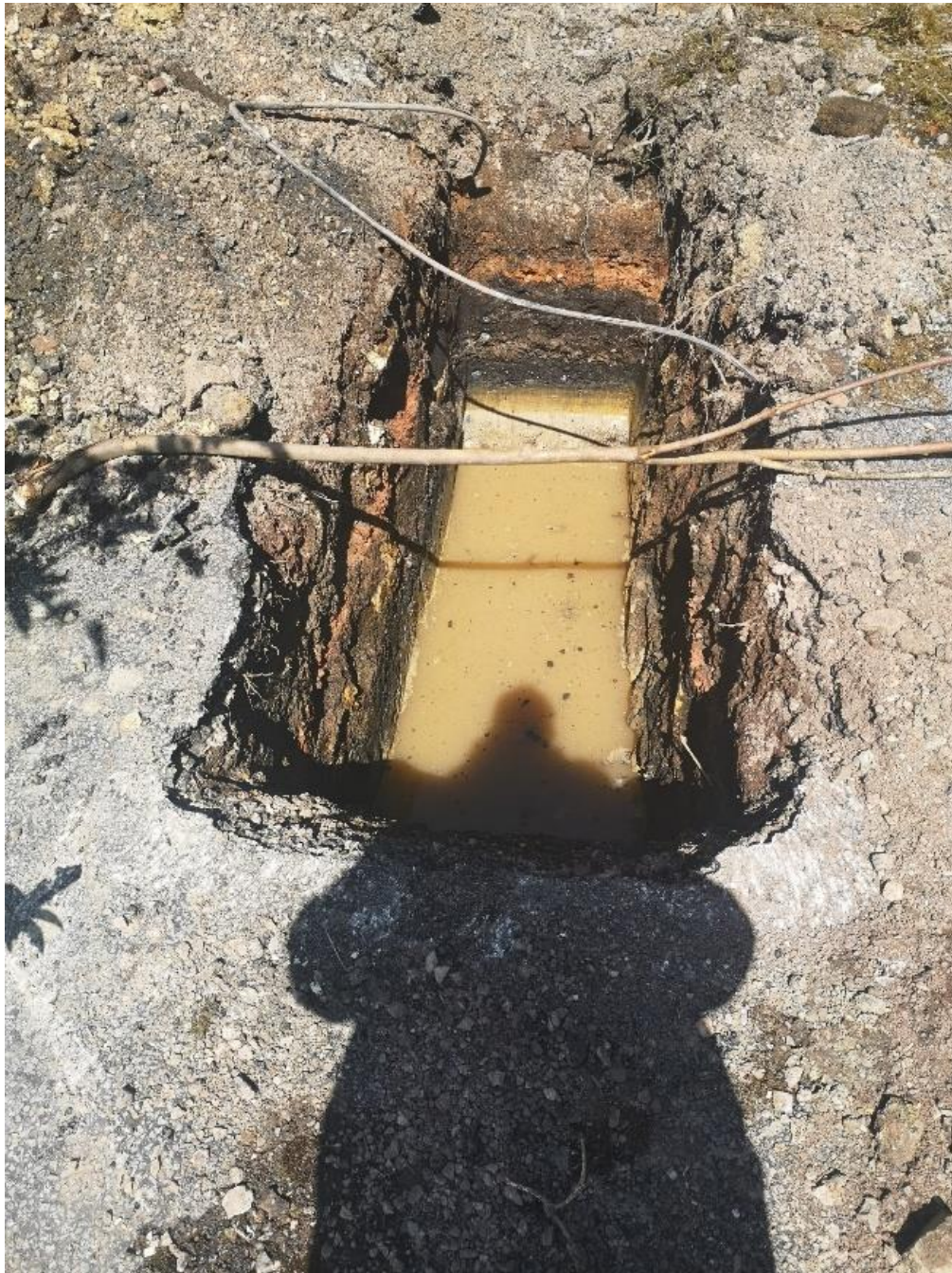
Figure 21 Engineer's test pit showing layers of material levelling up site in sections (Photo D. Bailey).
