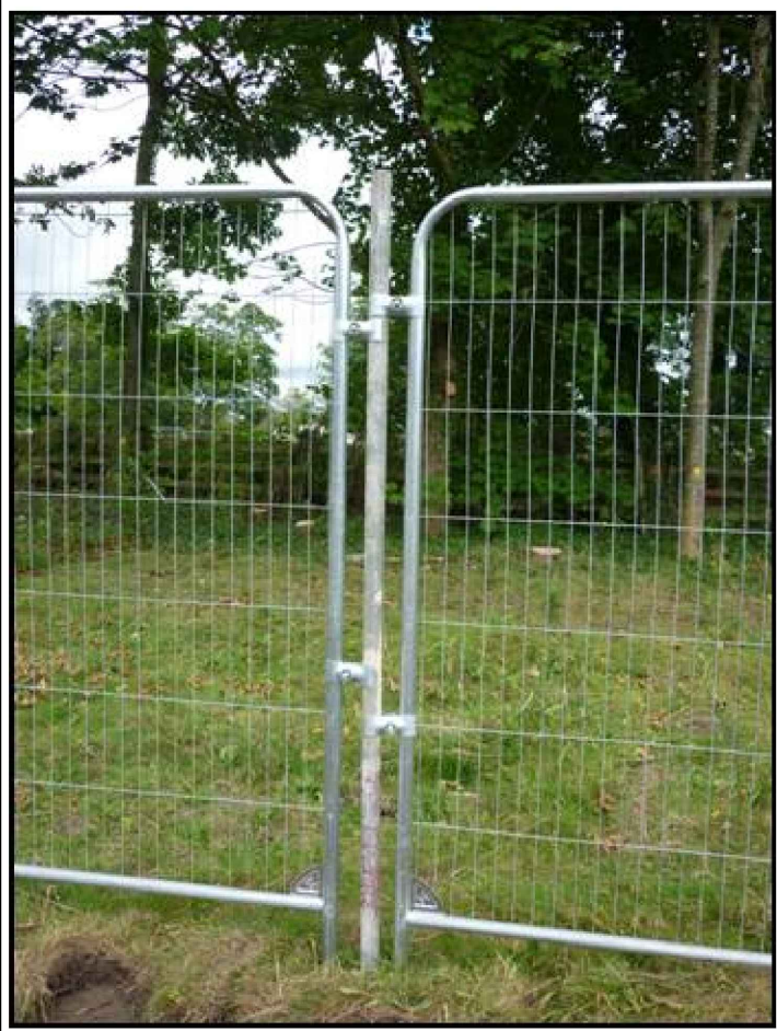
Tree Protective Fencing Specification
