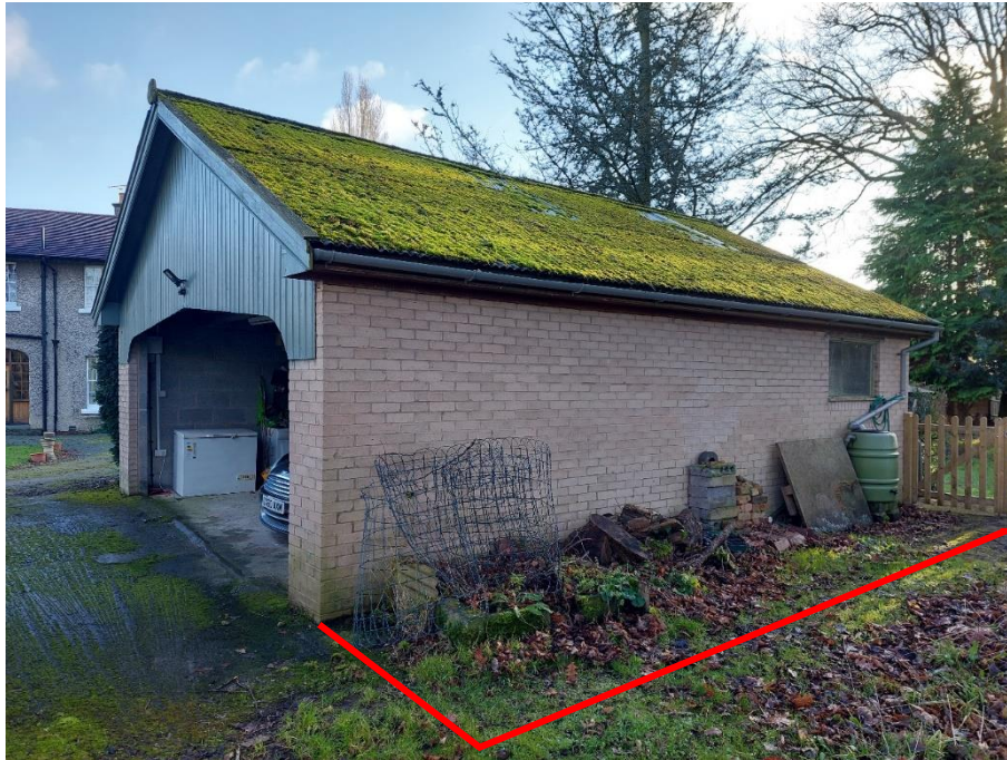
Figure 4.3. Site as viewed from northwest with area of hardstanding in red
