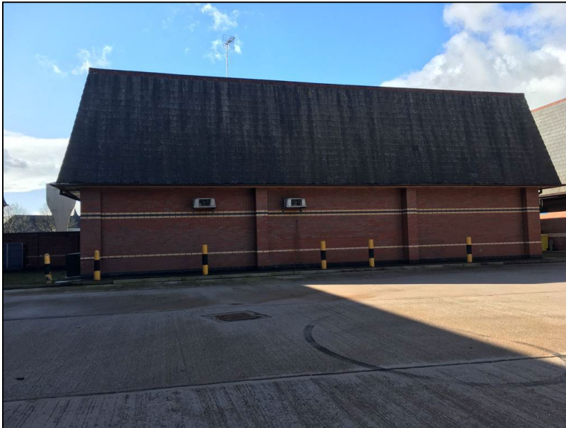
Photograph 1 Site view - rear of building
