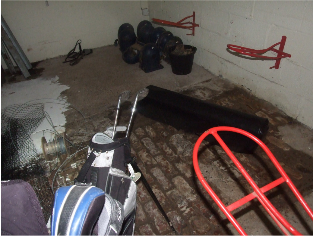
Brick and concrete ground floor
