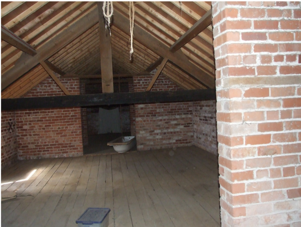
First floor timber floor and truss.
