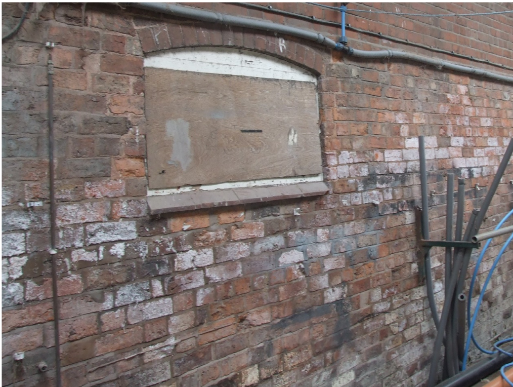
Rear elevation within adjacent barn.
