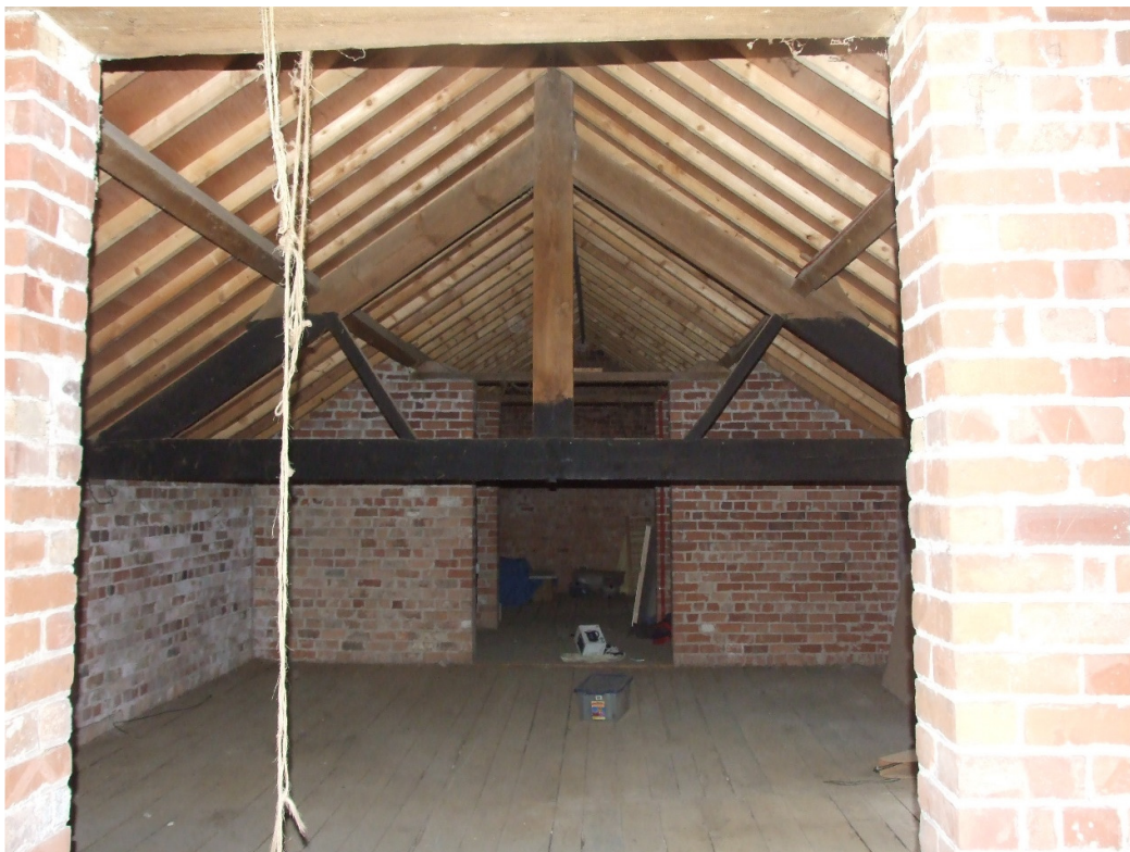
First floor internal, showing truss and walls along with rafters, purlins and sarking board.
