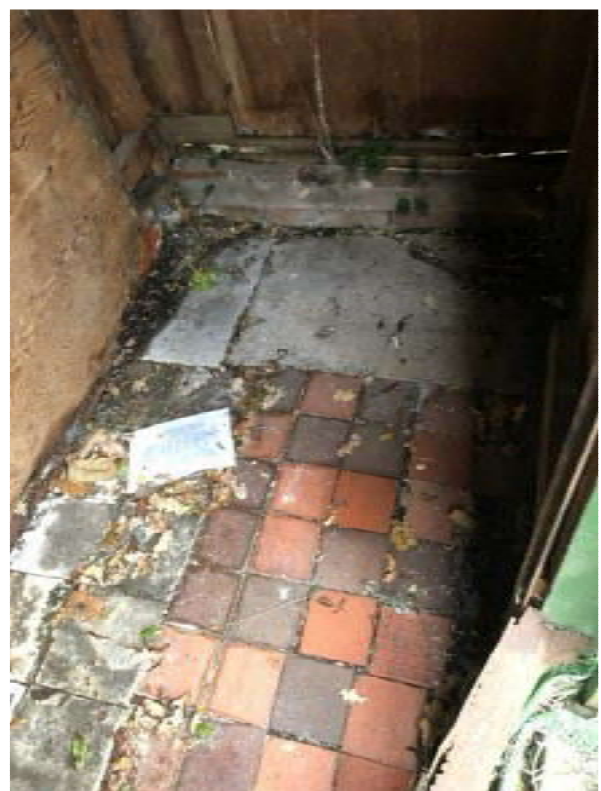
Quarry-tiles to floor of smaller outbuilding
