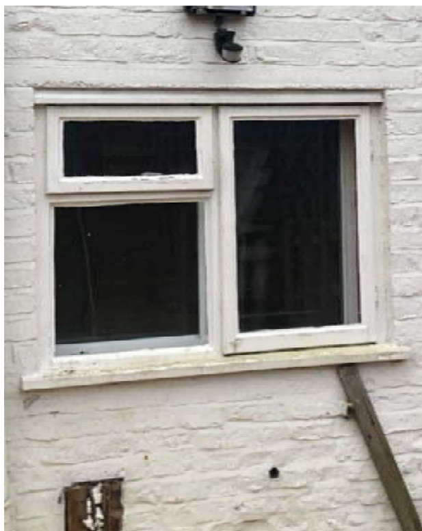
Image 1: Existing ground floor window
