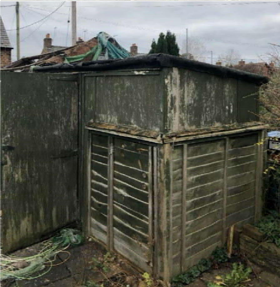
Rear of outbuilding
