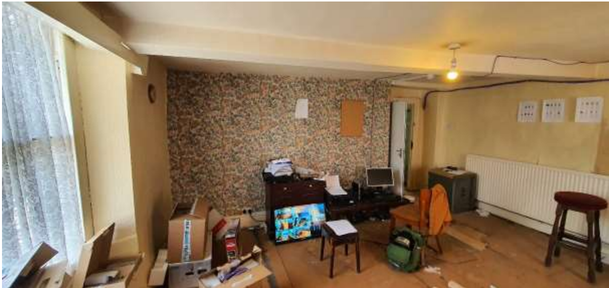
F04. General refurbishment in order to reinstate accommodation to upper levels.
