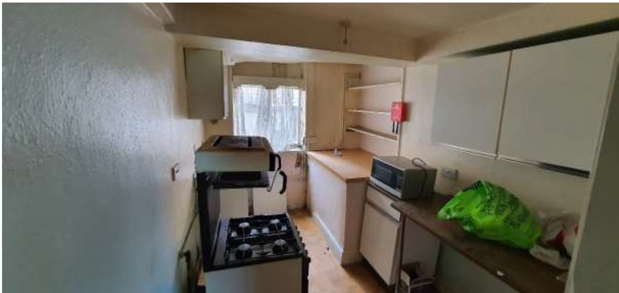
F08. New kitchen installed.
