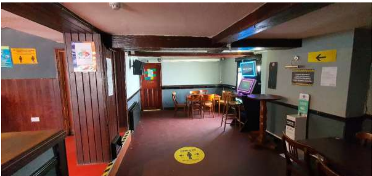
G09. New fixed seating along wall. New carpet and cosmetic redecoration works. New opening formed to structural wall.
