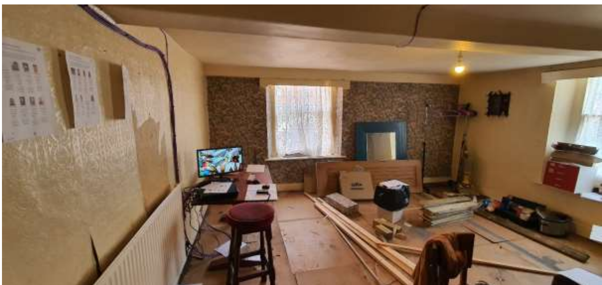
F03. General refurbishment in order to reinstate accommodation to upper levels.
