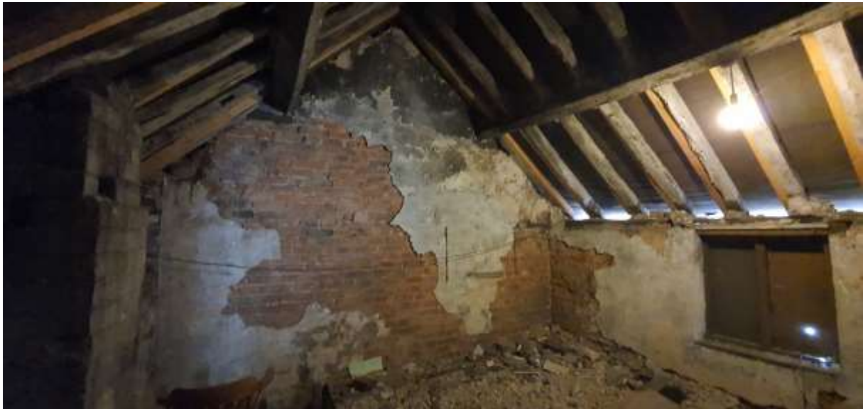
F19. General clear out and roof repairs for use at a later date.
