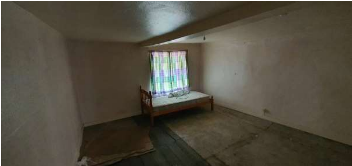
S07. General refurbishment in order to reinstate accommodation to upper levels.
