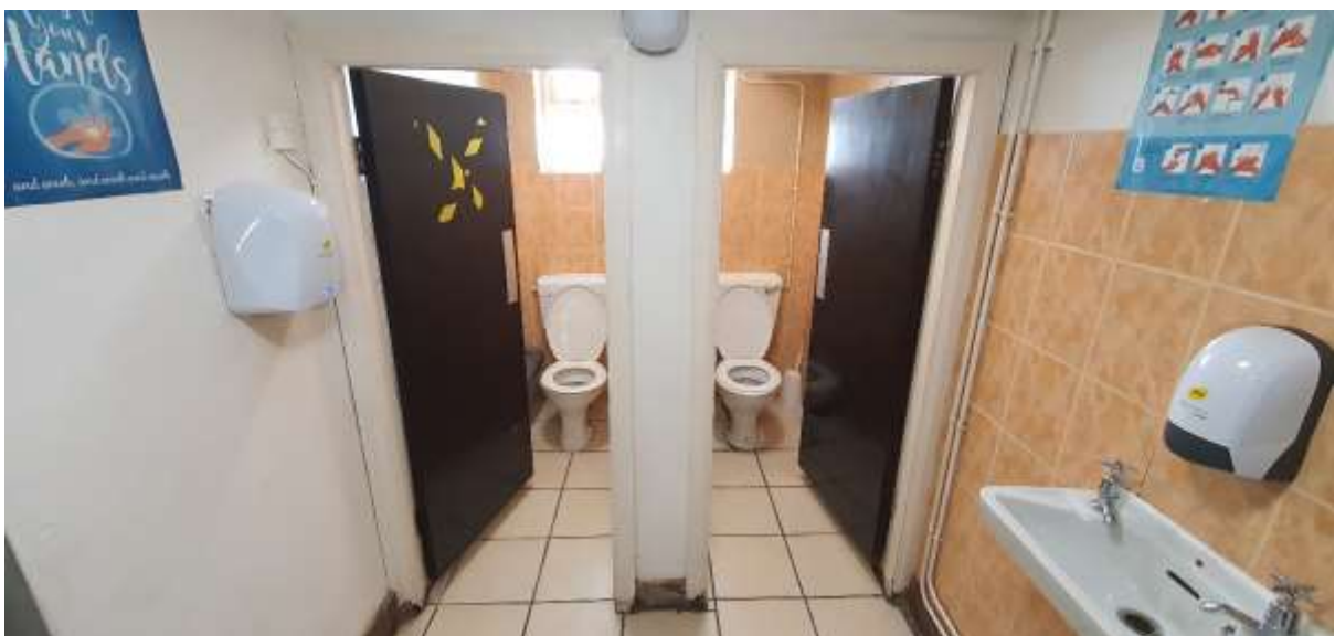
G12. Toilets removed and relocated. This area is to be opened up in to the public area with the opening formed within the existing wall on the right.
