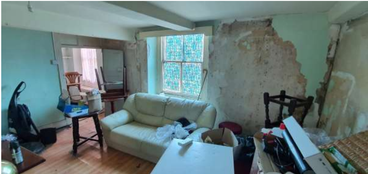
F07. General refurbishment in order to reinstate accommodation to upper levels.
