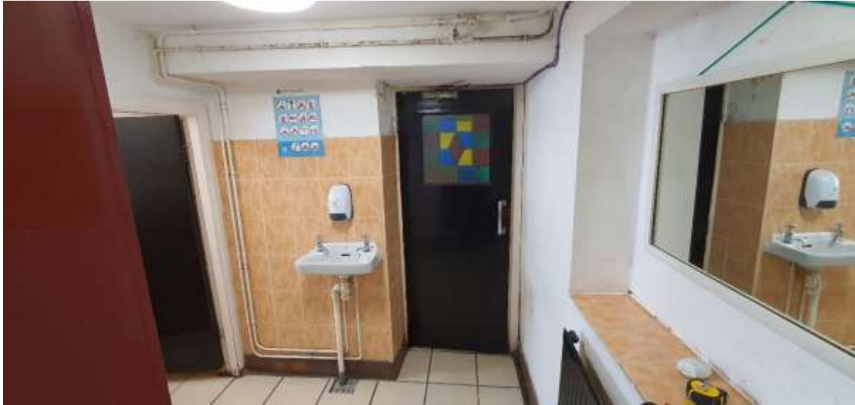
G13. Toilets removed and relocated. This area is to be opened up in to the public area with the opening formed within the existing wall.
