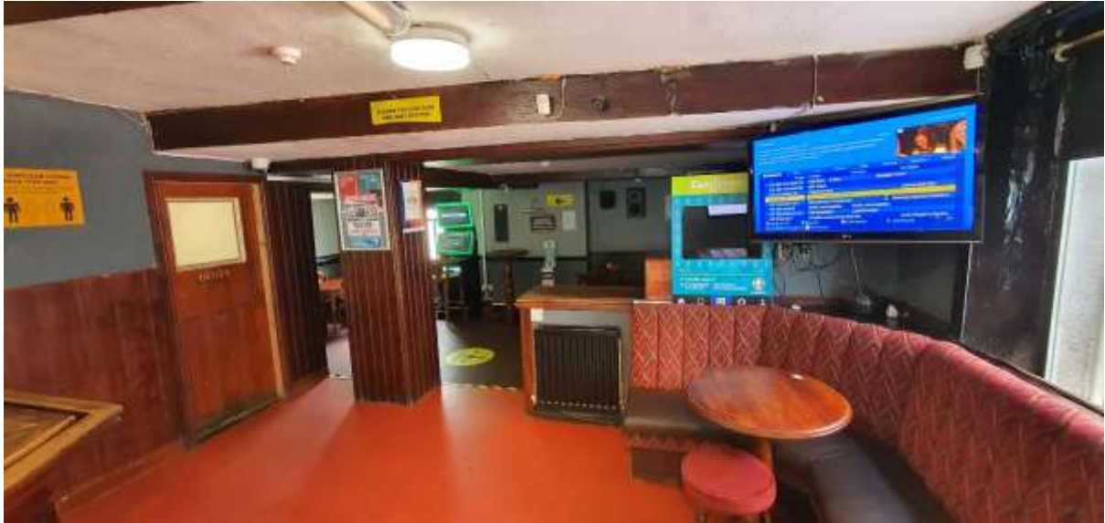
G04. Fixed seating removed. New timber flooring and cosmetic redecoration works.
