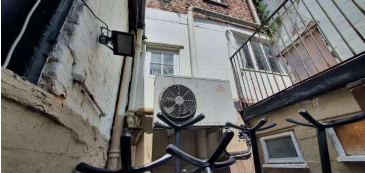
G18. Existing Yard area to be enclosed to form new toilet facilities.
