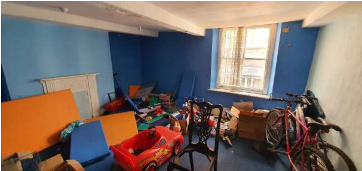
F13. General refurbishment in order to reinstate accommodation to upper levels.
