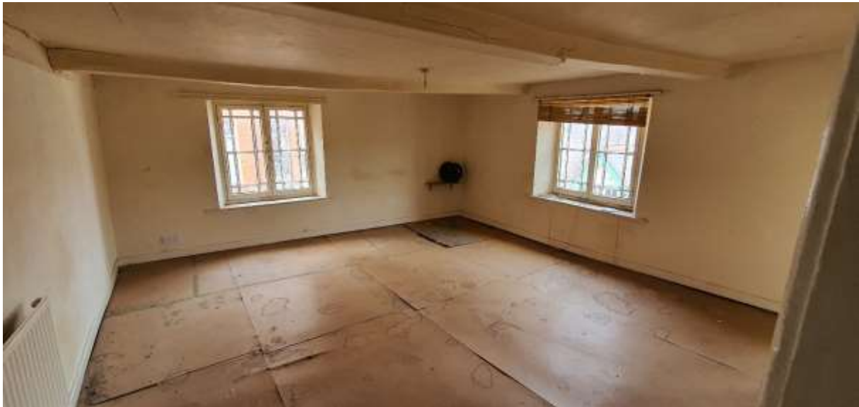
S01. General refurbishment in order to reinstate accommodation to upper levels.
