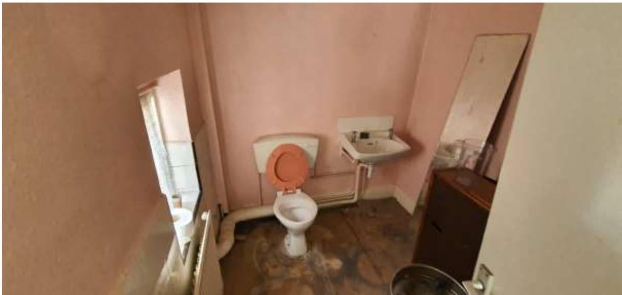
F11. General refurbishment in order to reinstate accommodation to upper levels.
