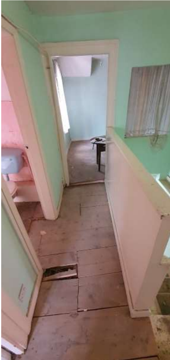
S09. General refurbishment in order to reinstate accommodation to upper levels.
