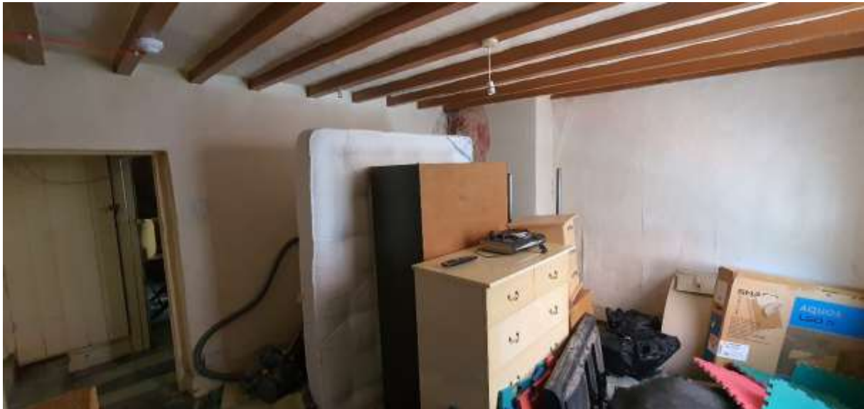
F16. General refurbishment in order to reinstate accommodation to upper levels.
