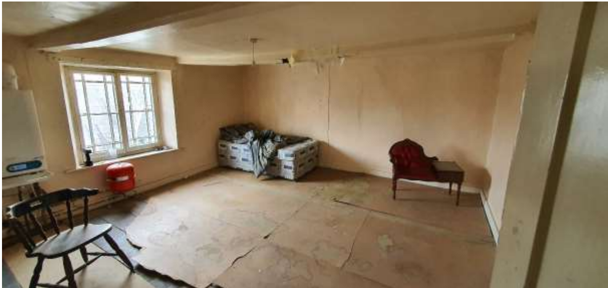
S04. General refurbishment in order to reinstate accommodation to upper levels.
