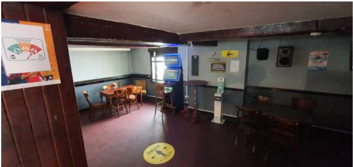
G08. New fixed seating along wall. New carpet and cosmetic redecoration works. New opening formed to structural wall.
