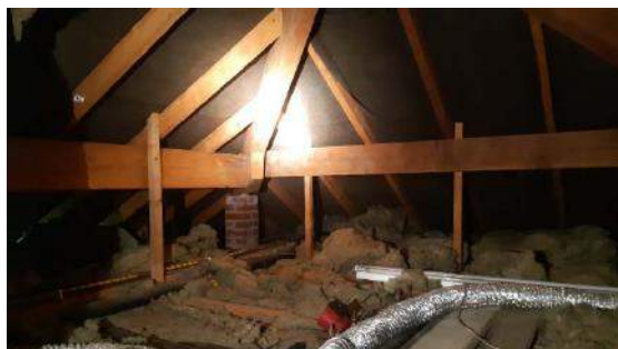
Photograph 8. Southern end of main roof space, with bitumen felt lining and insulated floor.
