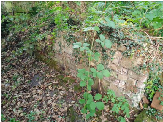
Photo 3 – Typical condition of external wall.
