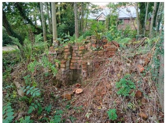
Photo 5 – Typical view of chimney
