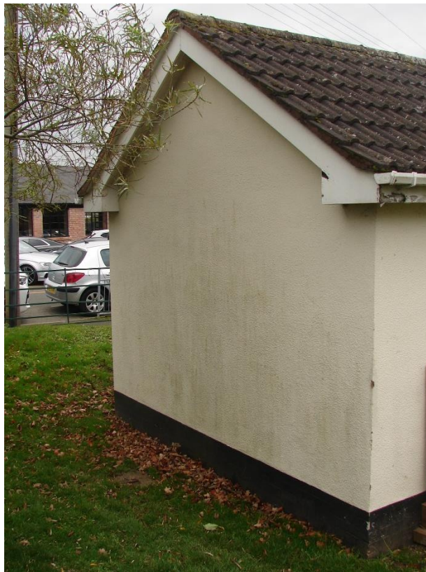
The northwest elevation.
